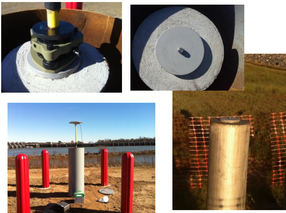
Figure 2-7. Reference point monumentation. Concrete pier construction vicinity of a lock and dam. Forced centering plug set into concrete pier. (Little Rock District).
