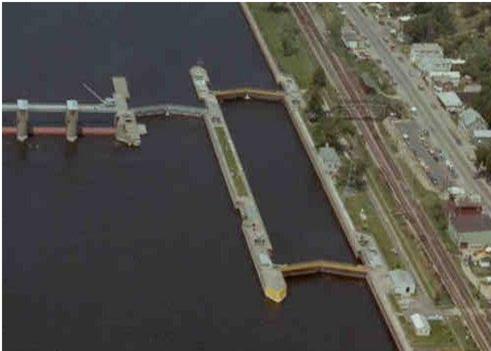
Figure B-3. Lock and Dam No. 4 showing Intermediate Wall and Land Wall.
