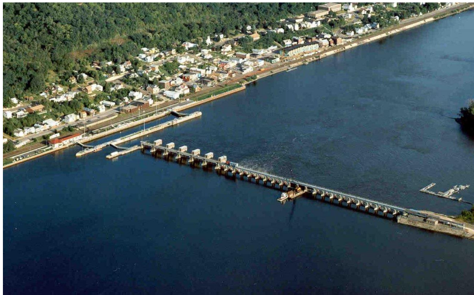
Figure B-2. Aerial View of Lock and Dam No. 4, Alma, WI.
