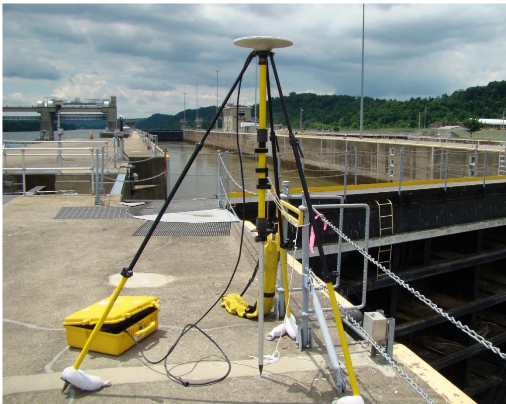
Figure 3-4. GPS equipment setup on Racine Lock and Dam.
