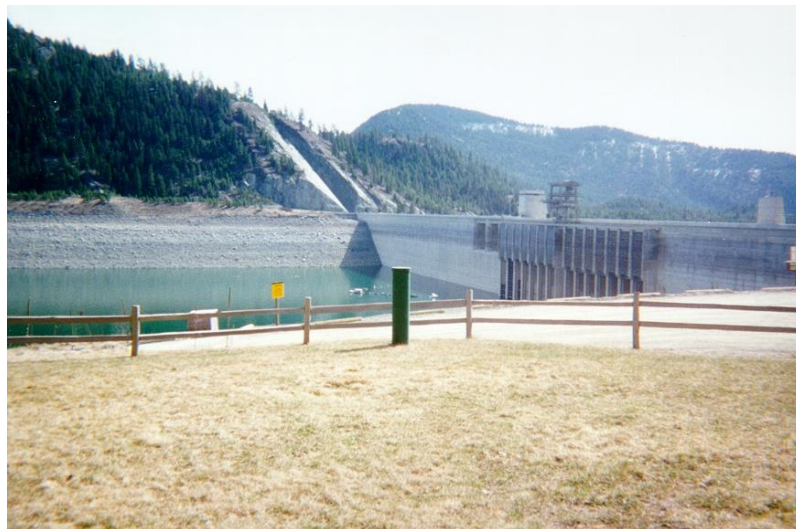
Figure C-5. Existing survey station, Libby Dam.
