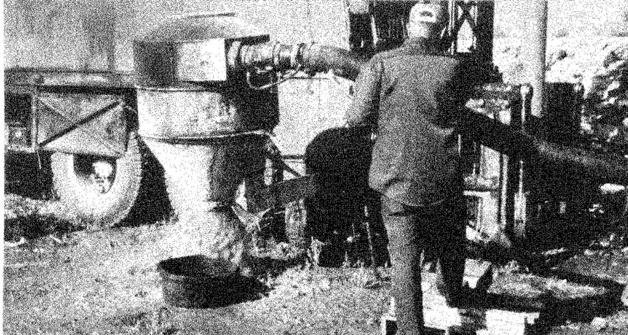
**Figure 3-9. Soil is collected by a cyclone during Becker hammer drilling operations (Harder 1993). Note: Safety is a very important consideration for Corps of Engineers projects. Safety items, including hardhats, gloves, safety shoes, protective clothing, and dust or vapor masks, should be worn, as appropriate, for the particular drilling and sampling operations**
