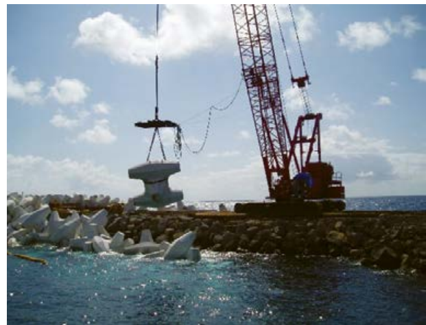
Figure 18. Core-locs and Core-loc placement on the jetty at Kaunapali Harbor, Lanai, HI in 2007.
