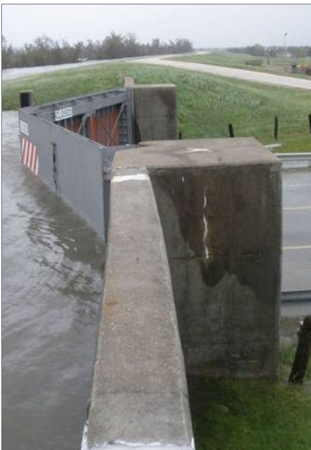
GATE CLOSURE DURING HIGH WATER, PRAIRIE DUPONT LEVEE SYSTEM PROJECT, DUPO, ILLINOIS.
