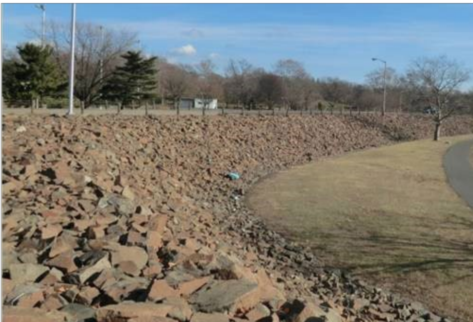
EMBANKMENT ARMORED WITH RIPRAP, STAMFORD HURRICANE/SHORELINE PROTECTION PROJECT, STAMFORD, CONNECTICUT.
