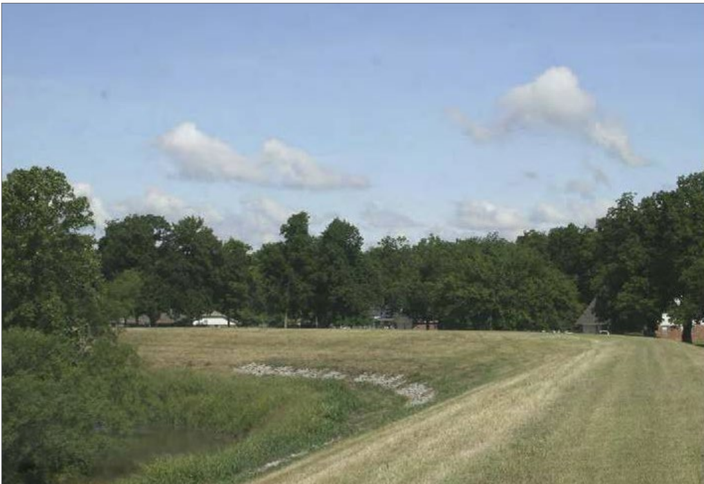
HAIKEY CREEK LEVEE. TULSA, OKLAHOMA
