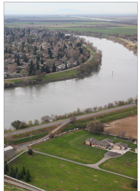
EARTHEN EMBANKMENT, SACRAMENTO RIVER LEVEE, SACRAMENTO, CALIFORNIA
