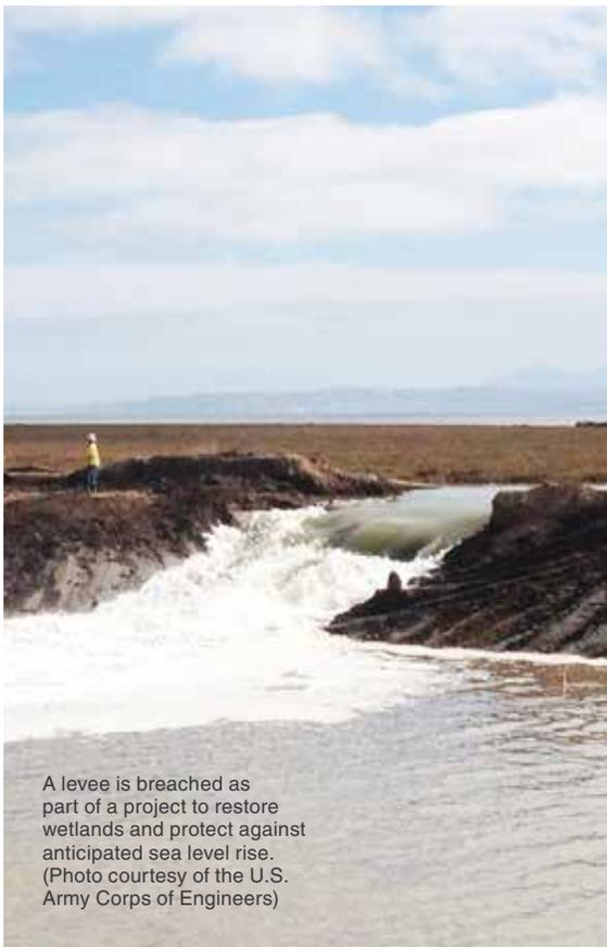
A levee is breached as part of a project to restore wetlands and protect against anticipated sea level rise. (Photo courtesy of the U.S. Army Corps of Engineers)
