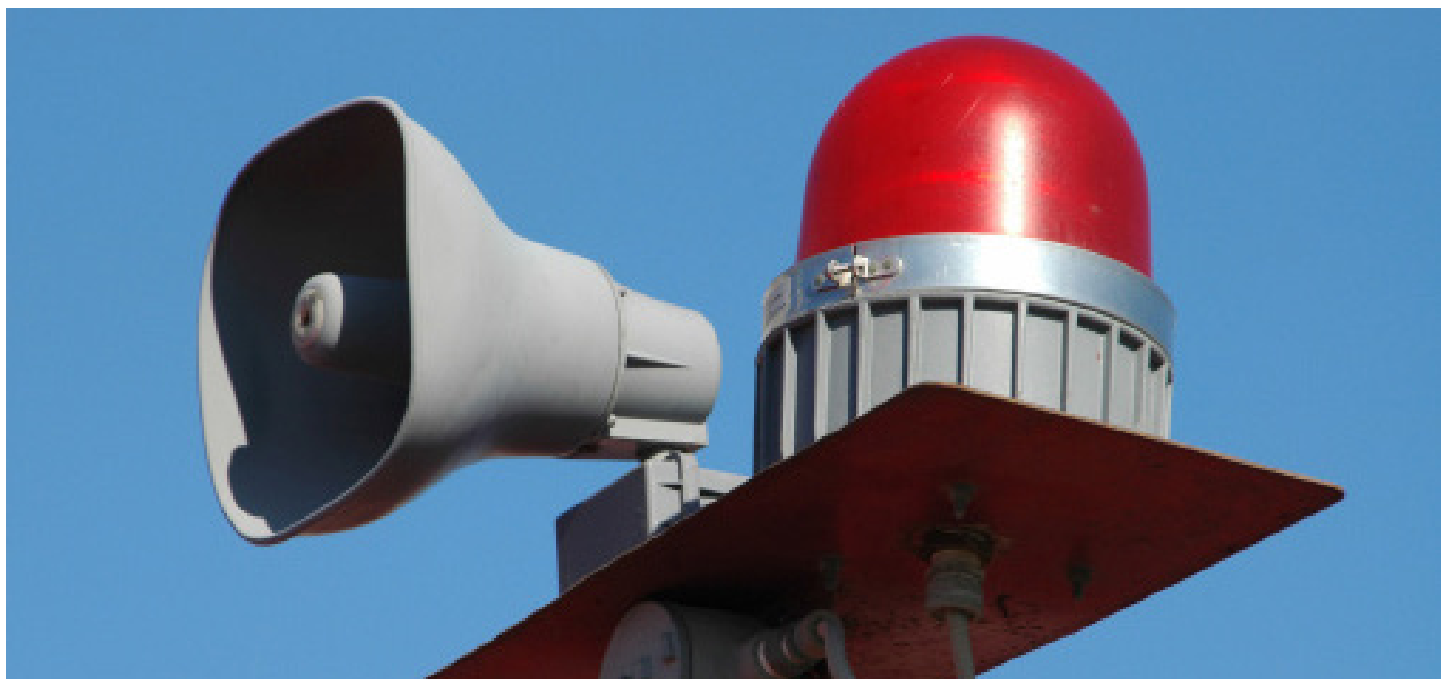
Warning siren with visual alerting capabilities. Assists with alerting hearing impaired.
