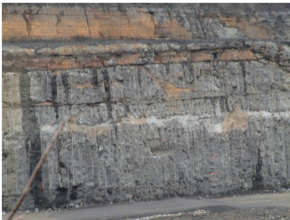
Figure 6-8. Over 1.5 Million Feet of Detonating Cord used on USACE Precision Presplit Project, Grundy, VA.
