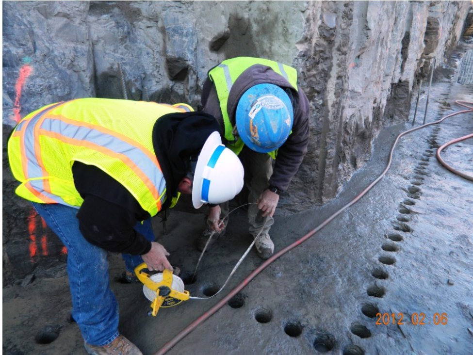
Figure 6-13. Line Drilling Holes on an inside and outside Corner. Crew Checking the Depths to Quality Control (QC) the Drillers Work.
