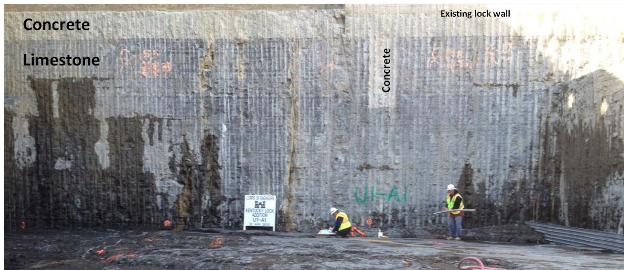
Figure 6-6. Line Drilling at Kentucky Lock Project Used for Construction of Excavation for New Lock Chamber Located Adjacent to and Immediately below the Existing Lock Wall.
