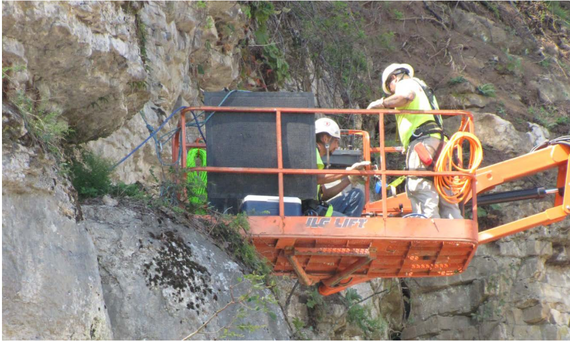
Figure 6-21. Airbag with Scalers in a Man Lift before Being Placed behind a Large Unstable Column of Rock to Be Removed from a Slope.
