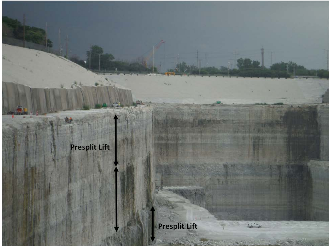
Figure 6-5. View of Highwall Excavation in Limestone Using Presplit Blasting with up to 125 ft Presplit Lifts.
