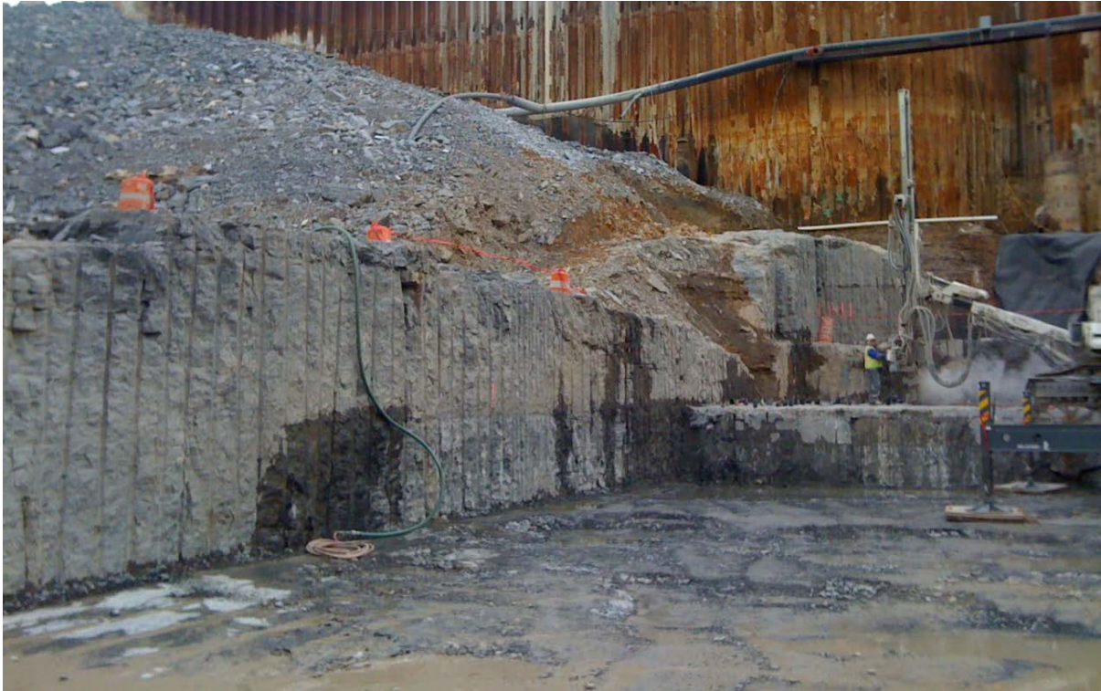
Figure 4-1. View of “Half Casts” on Rock Slope after Blasting at Kentucky Lock.
