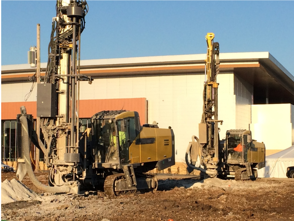
Figure 4-5. Two Air-Percussion OHD Drill Rigs. Note Pile of Rock Fines (Drill Cuttings) in Front of the Rigs Removed from the Hole.
