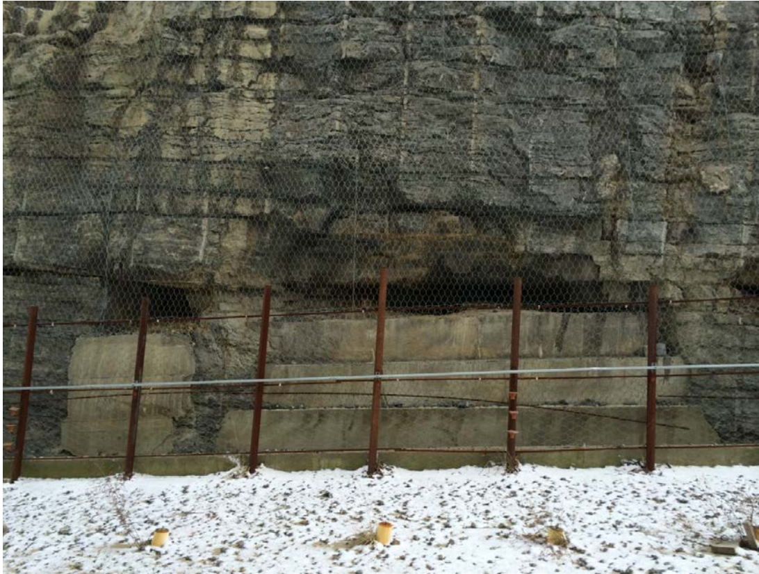
Figure 3-9. View of Karst Feature at Base of Presplit with Concrete Added at Cave Mouth.
