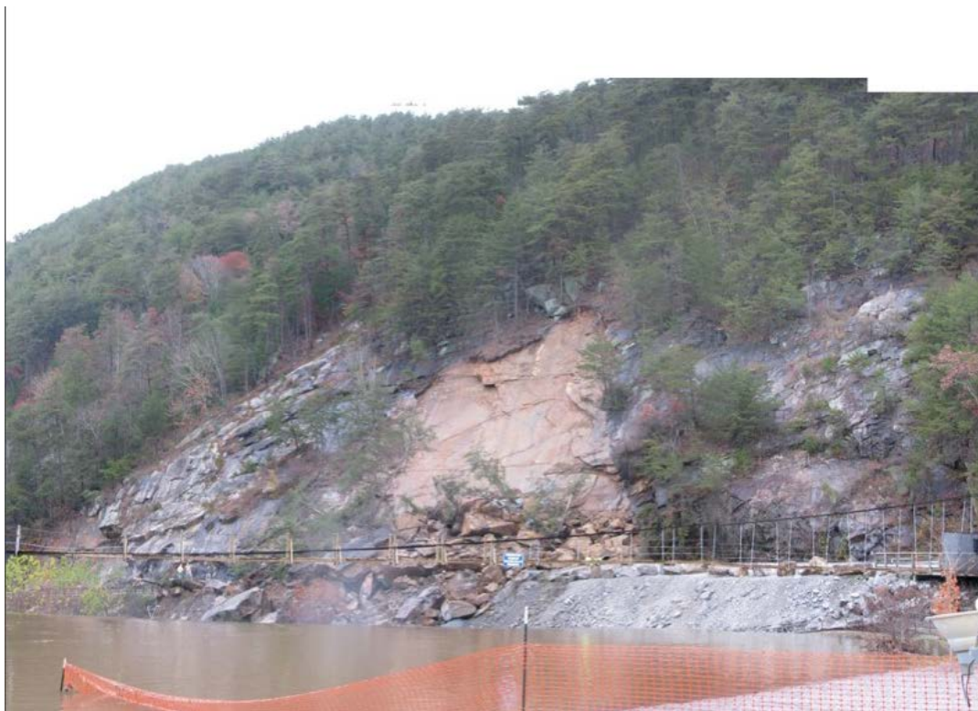
Figure 6-17. Rock Slide along US64 in the Ocoee River Gorge across from Parksville Dam, Immediately after the Slide.
