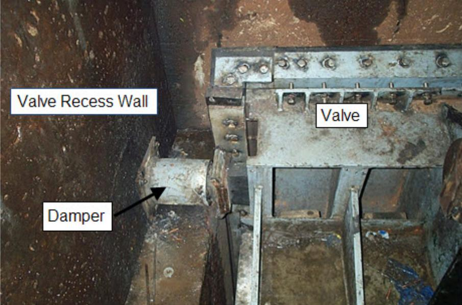
Figure 5-2. Damper attached to valve recess wall, Chickamauga Lock (top view looking downstream).
