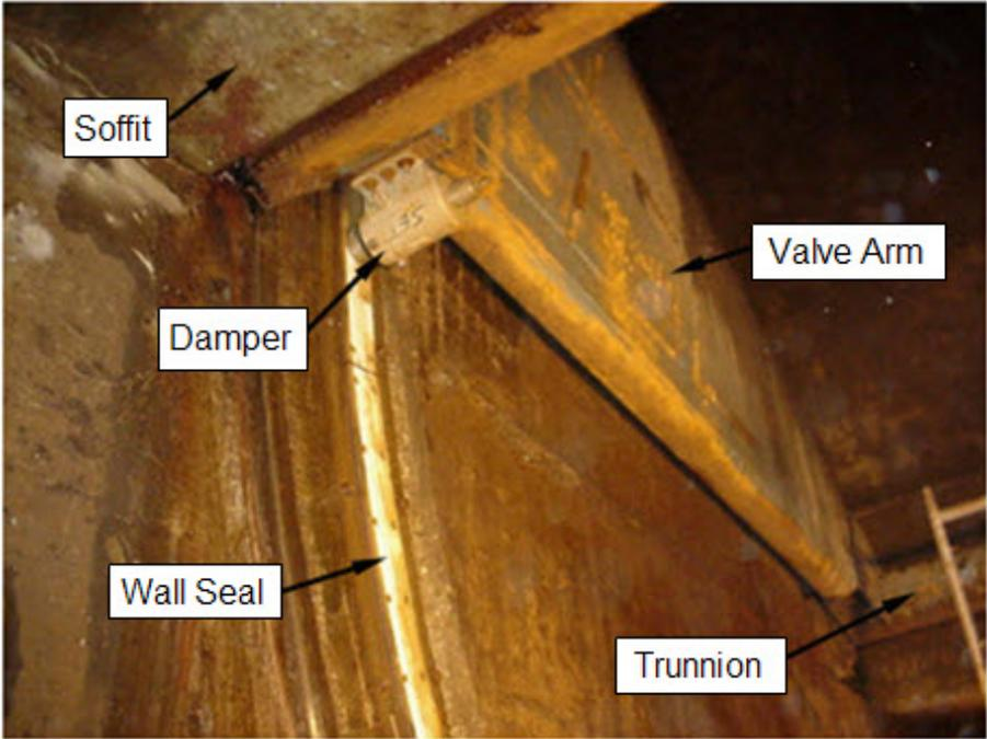
Figure 5-1. Damper attached to bottom of valve arm, Eisenhower and Snell Locks.
