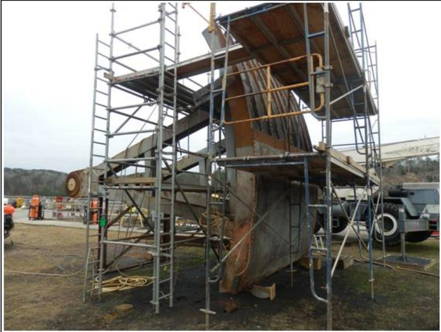
**Figure B-1. Repairing cavitation damage on Bankhead Lock valve skin plate.**
