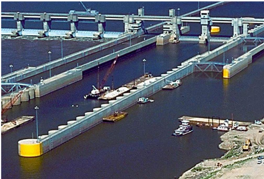
Figure 6.1. Semi-Circular Bullnose Structure
