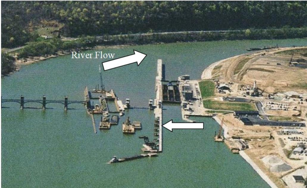
Figure C.8. Upper Approach Guard Wall at Winfield L&D
