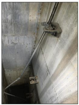
(Courtesy of USACE Louisville District) Figure 9-1. Failed closure system due to damaged sluice gate stem.
