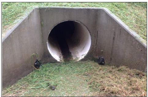
(Courtesy of Louisville District) Figure 5-30. Landside headwall with seepage filter drainage ports.
