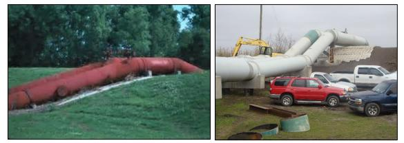
(From America's Wetland Foundation Resource Center [left] and Courtesy of USACE New Orleans District [right]) Figure 1-4. Pressurized water pipe installation elevated over levee sideslopes and crest.
