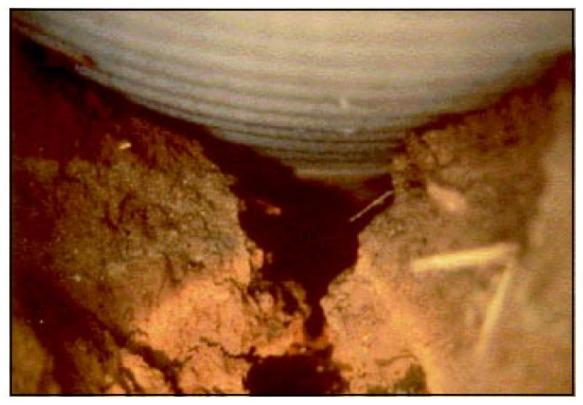
(From Low-Volume Roads Engineering, USDA-Forest Service, 2003) Figure 2-6. Substantial void space beneath pipe caused by poorly placed backfill.
