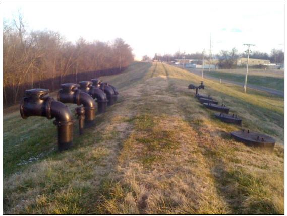
(Courtesy of USACE Louisville District) Figure 6-11. Potential inspection access points for pump station discharge pipes.
