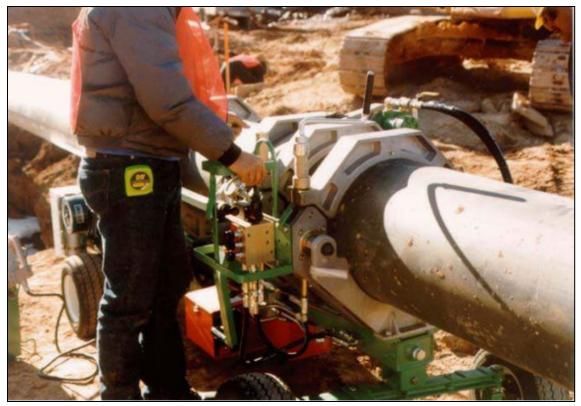
(From FEMA, 2007) Figure 5-35. Apparatus for heat fusing solid-wall high density polyethylene (SW-HDPE) pipe.
