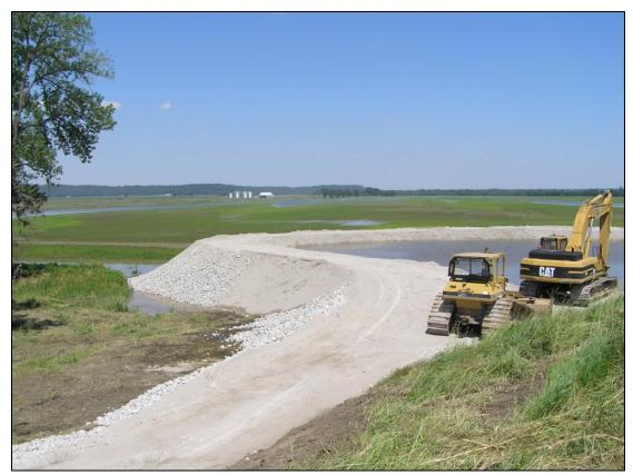
(Courtesy of USACE St. Louis District) Figure 2-61. Landside intervention using an aggregate berm to retain flow of 36-inch pipe.
