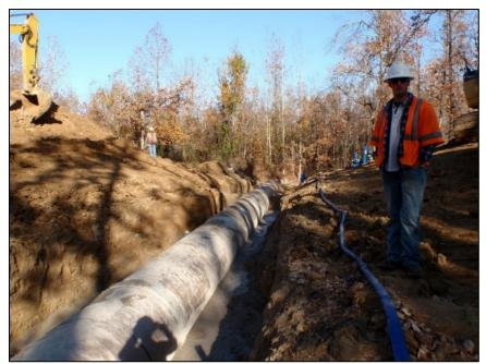
(Courtesy of USACE Louisville District) Figure 1-3. Non-pressurized gravity fiber-reinforced pipe installation within an embankment.
