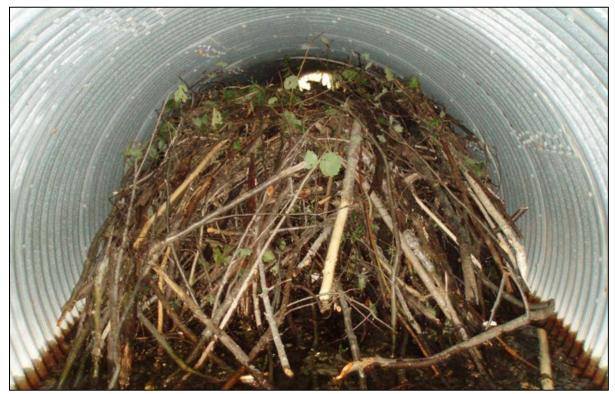
(Courtesy of Lizotte Solutions) Figure 2-55. Internal debris accumulation severely restricting flow.
