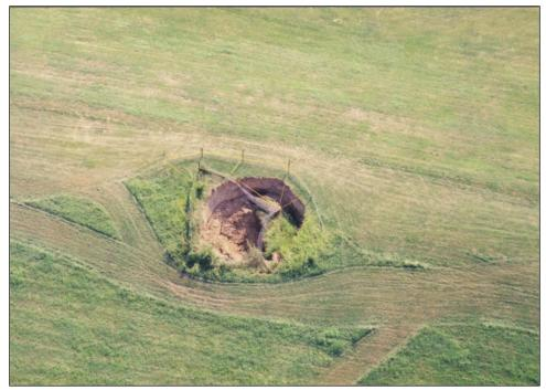
(Courtesy of USACE Louisville District) Figure 8-1. Sinkhole in levee due to collapsed pipes.
