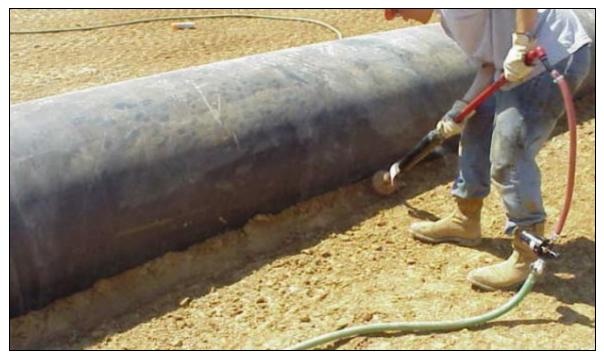
(Courtesy of FEMA) Figure 5-23. Compaction of Soil Backfill in the Pipe Haunches.
