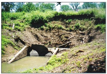
(Courtesy of USACE Louisville District) Figure 2-48. Result of successive slope failures around pipes.
