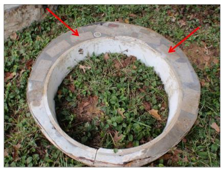
(Courtesy of USACE Louisville District) Figure 7-23. Concrete blocks and brick used to fill annular space in bulkhead zone.
