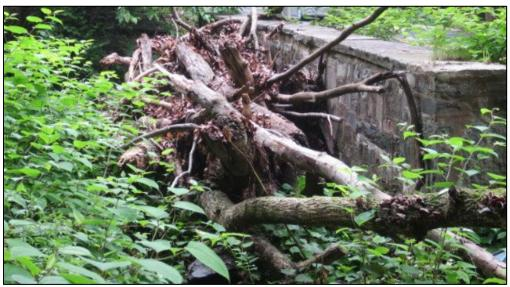
(Courtesy of Forest Hills CONNECTION, Marlene Berlin) Figure 2-56. External debris accumulation severely restricting flow.
