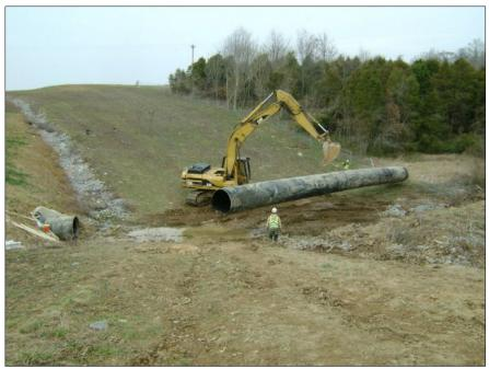
(Courtesy of Indiana Reline) Figure 7-22. Installation of two previously joined slip liner segments using headwall access.
