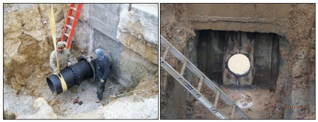
(Courtesy of USACE Louisville District) Figure 5-16. Penetrations through floodwall key (left and pipe #2 in Figure 5-15) and sheet piling (right and pipe #3 above).
