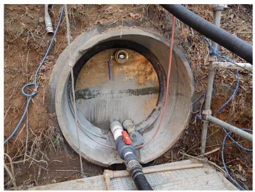
(Courtesy of Mobile Concrete and Grout of Alaska) Figure 8-3. Typical infill and vent ports through a temporary bulkhead.
