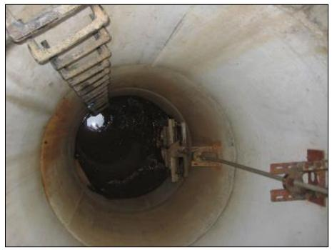
(Courtesy of USACE Louisville District) Figure 9-11. Typical manhole with sluice gate.
