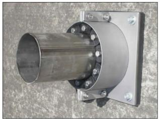
From SPEC-NET, 2017) Figure 5-45. Casing with a surface-mounted flange and annular seal on existing floodwall.
