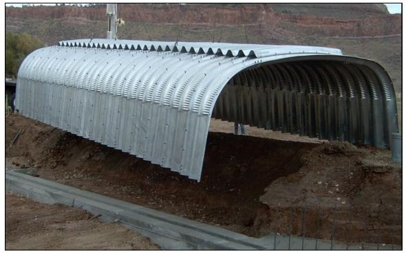
(Courtesy of National Corrugated Steel Pipe Association) Figure 3-4. Installation of a corrugated steel box culvert.
