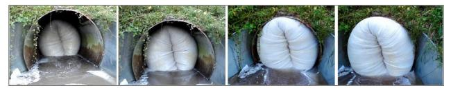
(From JTV Inc., 2017) Figure 7-28. Fabric tube advances through host pipe as pressure is applied during the inversion process.
