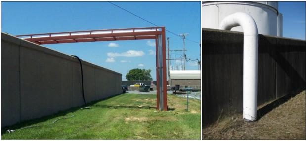
(Courtesy of USACE Louisville District) Figure 5-14. Supported (left) and freestanding (right) pipes over a floodwall.
