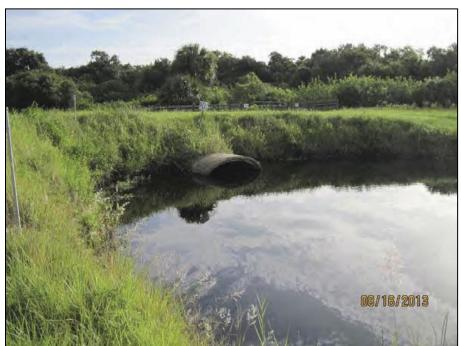
(Courtesy of USACE Jacksonville District) Figure 9-24. Pipe without a gate for canal water level control.
