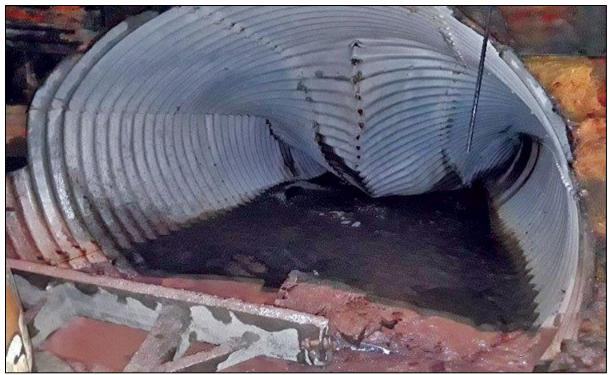
(From Trenchless Technology Magazine, 2019) Figure 2-54. Pipe deformation that could restrict flow and cause interior ponding.
