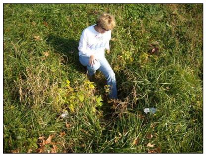
(Courtesy of USACE Louisville District) Figure 2-31. Collapsed toe drain accepting soil infiltration.
