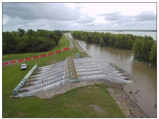
(From FOX 8 WVUE-TV, Plaquemines Parish, LA) Figure 5-10. Vehicular traffic routed around large diameter siphon pipes over levee crest.
