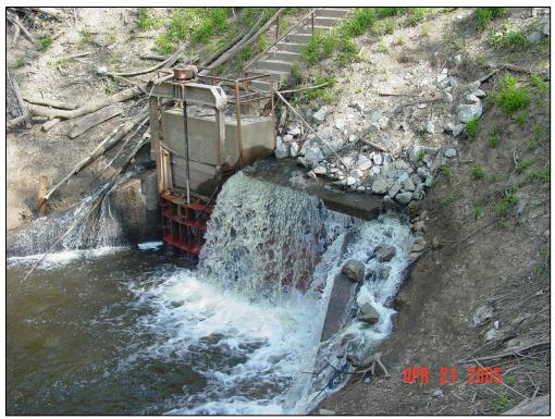
(Courtesy of USACE Louisville District) Figure 2-14. Trapped interior water (pressurizing pipe) exits through corrosion holes.
