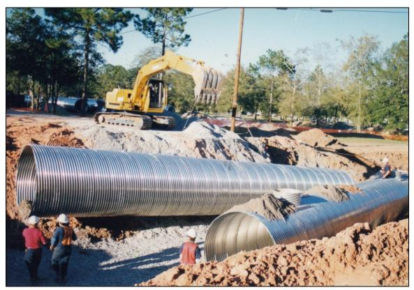
(Courtesy of the Aluminum Association) Figure 3-5. Installation of a corrugated aluminum culvert.
