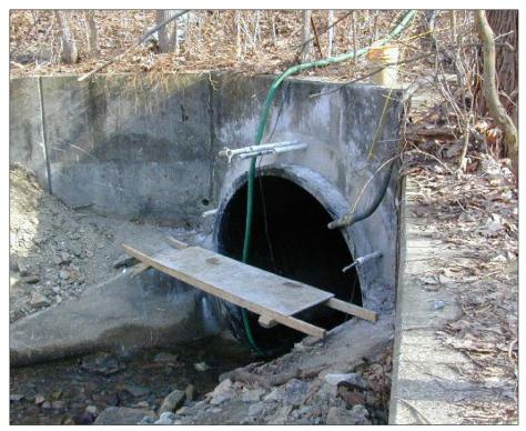
(Courtesy of IPC Sales) Figure 7-25. Grout ports through bulkhead.
