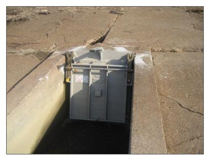
(Courtesy of USACE Louisville District) Figure 9-14. Typical headwall with wingwalls and flap gate on concrete slope.
