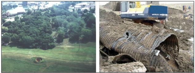
(Courtesy of USACE Louisville District) Figure 2-23. Holes in a pipe allowed continued soil loss to create a sinkhole in the levee crest.
