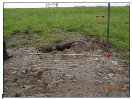
(Courtesy of USACE St. Louis District) Figure 2-25. Sinkhole over a gravity drain, more than halfway up a 30-foot high embankment.
