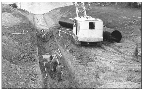
(Courtesy of USACE Louisville District) Figure 5-20. Manual construction of a soil pipe cradle for a 66-inch diameter pipe.
