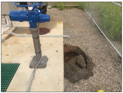
(Courtesy of USACE St. Louis District) Figure 2-32. Soil loss from compromised relief well collector pipe connection to pump station.
