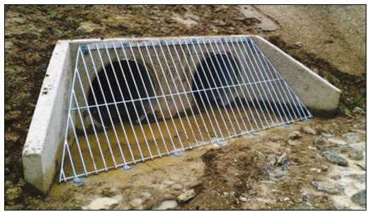
(From SPEC-NET, 2017) Figure 2-57. Fabricated debris screen for poured-in-place headwall.
