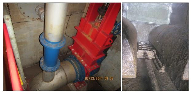
(Courtesy of USACE Louisville District) Figure 10-12. Bypass knife gate (left) and bypass valve (right).
