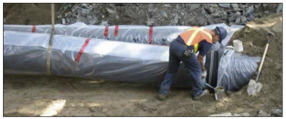
(Courtesy of Ductile Iron Pipe Research Association) Figure 3-11. Installation of DIP encased in polyethylene.
