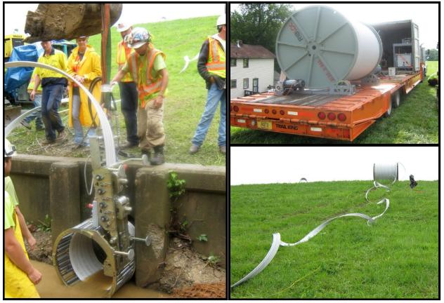
(Courtesy of USACE Louisville District) Figure 7-16. Setup at headwall access to install a fixed-diameter spiral wound pipe liner.
