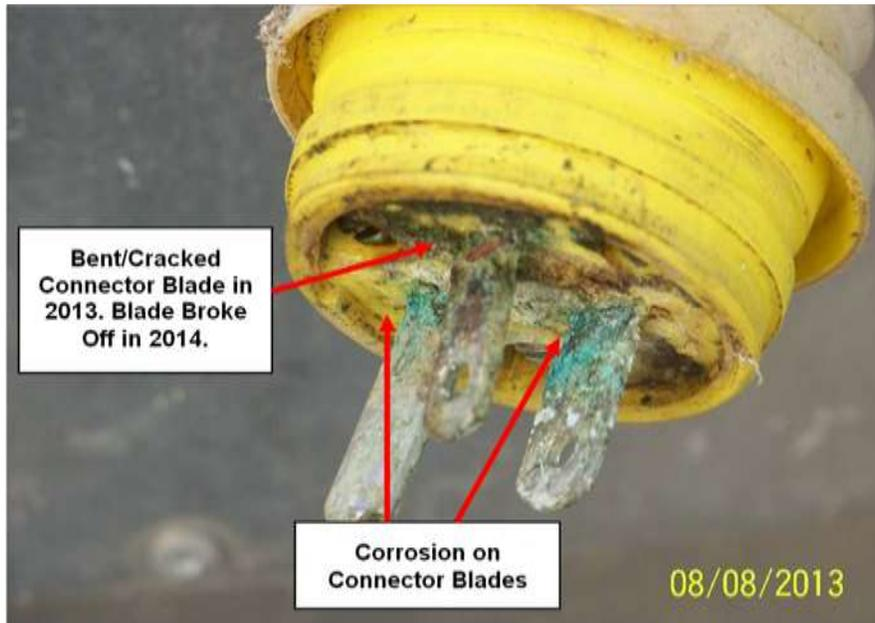
Figure J.5. Lower Gate, Right Leaf Rectifier AC Power Connector
