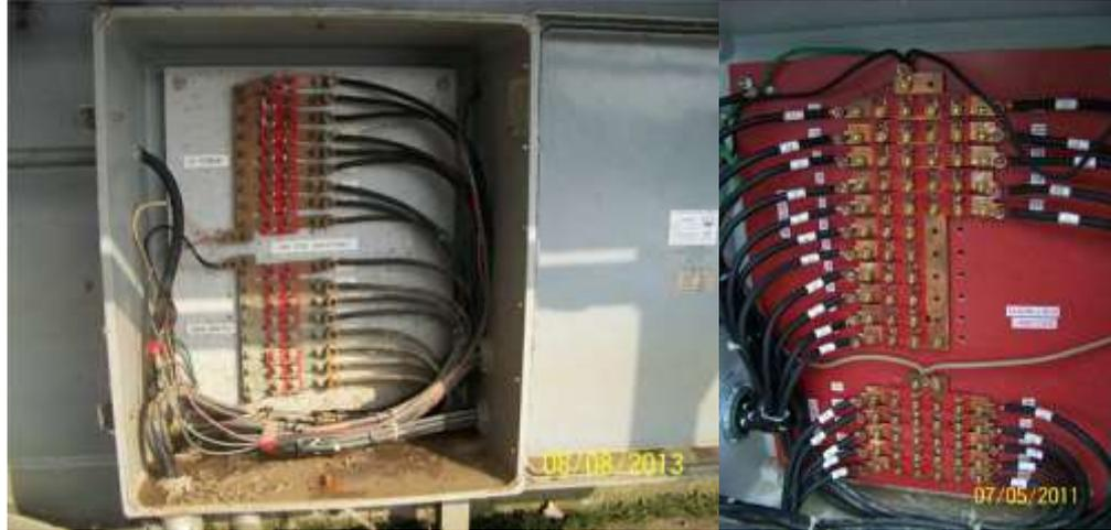
Figure J.12. Inside View of Typical Anode Terminal Cabinet, Upper and Lower Gates
