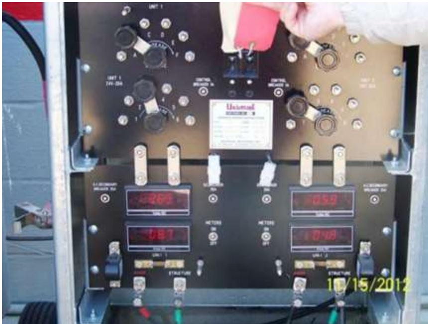
Figure G.4. Typical Interior View of One Rectifier
