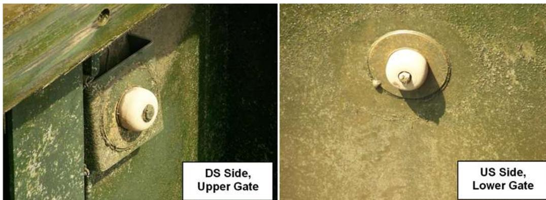
Figure J.11. Typical Button Anodes on Miter Gates
