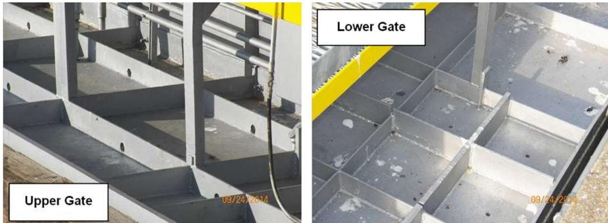
Figure J.1. Demopolis 2014—Coating Beneath Gate Walkway in Excellent Condition
