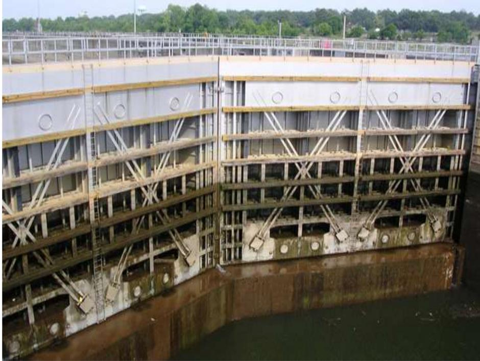
Figure I.7. Upper Gates, Downstream Side
