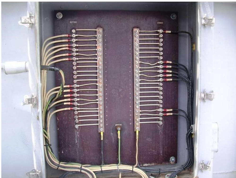
Figure I.9. Typical Inside View of Anode Terminal Cabinet
