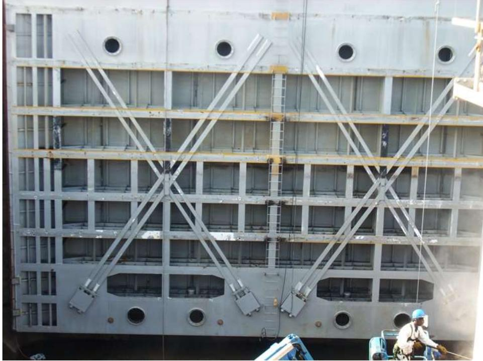
Figure K.3. View of Gates Showing Good Condition of Existing Paint
