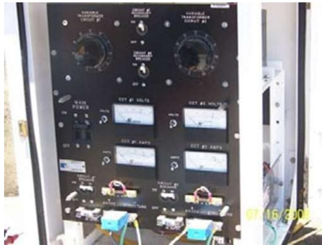
Figure F.4. Bankhead Lock Lower Left Gate Rectifier (Typical)
