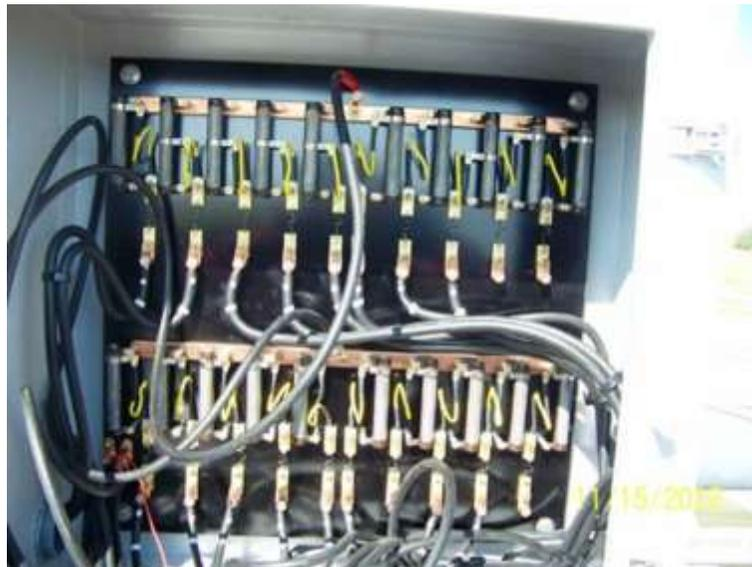
Figure G.6. Interior View of One Anode Terminal Cabinet
