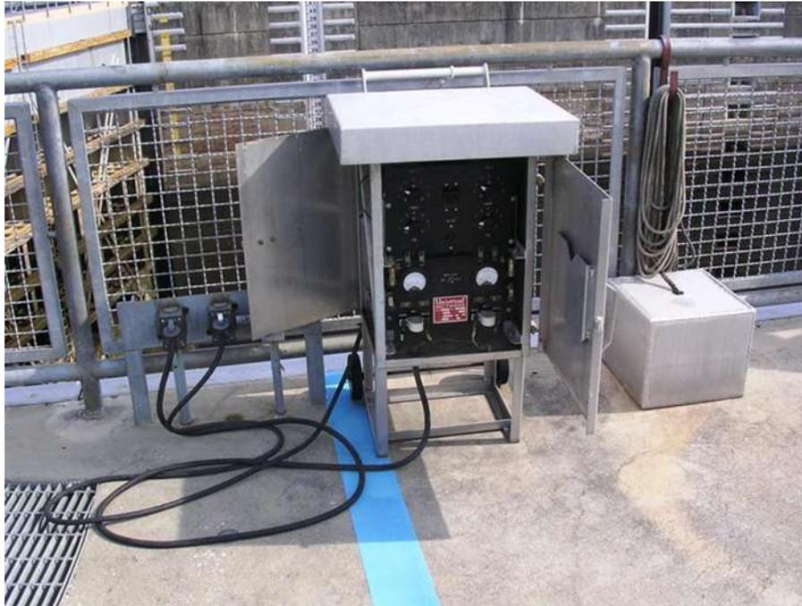
Figure I.5. Typical Rectifier at Oliver Lock
