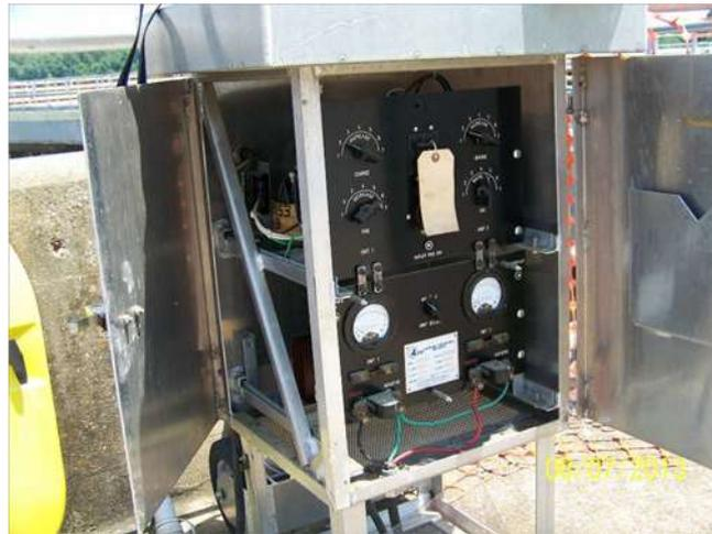
Figure J.13. Typical DC Rectifier, Demopolis Lock
