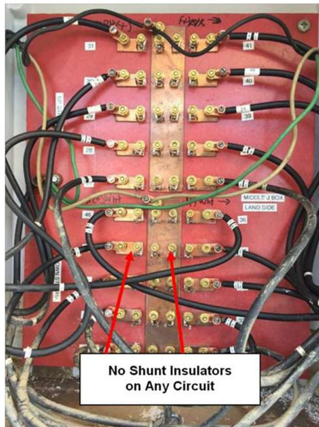
Figure J.4. Upper Gate, Anode Terminal Box, Shunts with No Insulators
