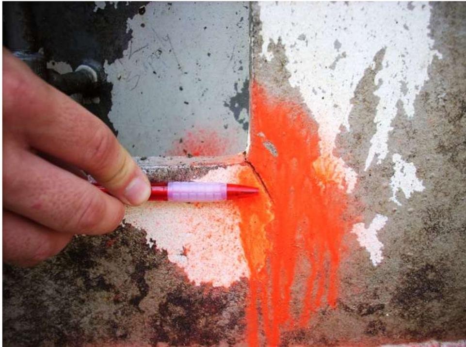
Figure K.4. Structural Cracks on the Downstream Side of the Lower Left Gate near the Quoin
