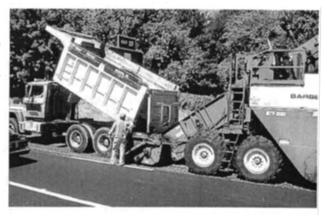
FIGURE 13-5 Material transfer vehicle.
