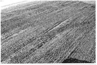
FIGURE 14-6 Tack coat on milled surface.
