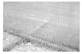
FIGURE 14-4 Bump caused by use of excessive crack sealant.
