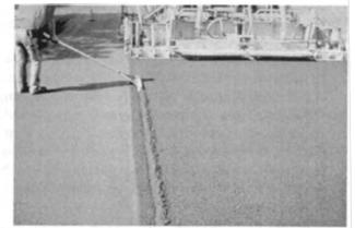
FIGURE 17-13 Raking of longitudinal joint.
