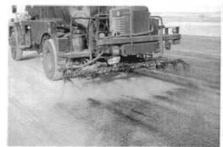
FIGURE 14-8 Improperly adjusted distributor.
