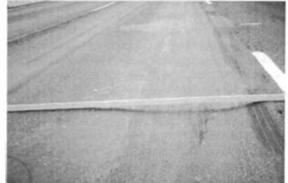
FIGURE 19-6 Rutting of unstable asphalt mixture.
