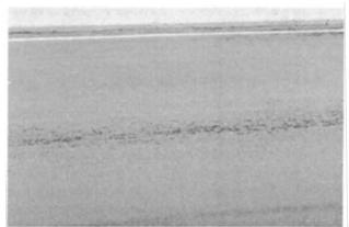
FIGURE 19-2 Poor longitudinal joint due to unsatisfactory workmanship.
