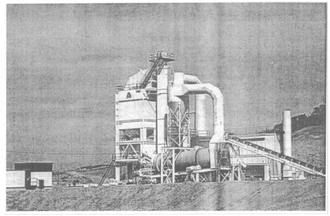
FIGURE 5-1 Typical HMA batch plant.
