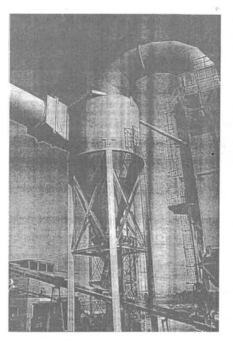
FIGURE 12-1 Vertical cyclone dry collector.
