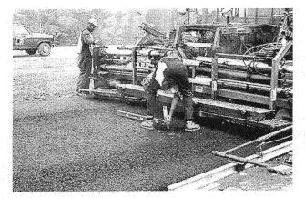
FIGURE 16-11 Checking slope of mat surface behind paver.
