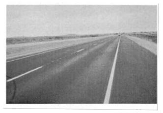
FIGURE 19-7 Asphalt bleeding in travel lane.
