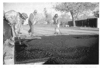
FIGURE 17-7 Excessive raking of transverse joint.
