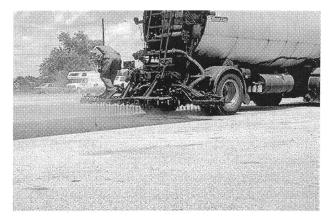
FIGURE 14-7 Distributor applying tack coat.
