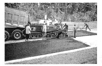
FIGURE 14-1 Patches placed with paving machine.
