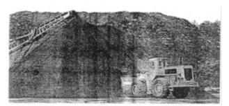
FIGURE 6-3 RAP stockpile using radial stack.
