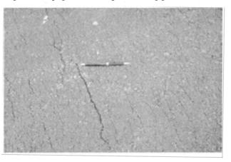
FIGURE 19-4 Hairline cracks caused by roller checking.
