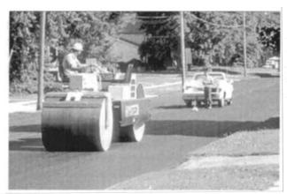
FIGURE 18-3 Static steel wheel roller.
