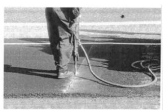
FIGURE 17-2 Removal of material at butt joint.
