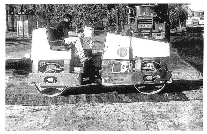
FIGURE 14-3 Compaction of patch.
