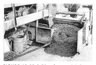
FIGURE 15-22 Buildup of excess mix in front of extended screed.
