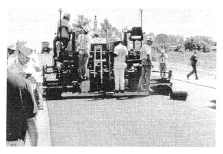
FIGURE 17-17 Compaction of mix in wedge joint.
