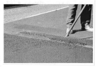
FIGURE 17-6 Raking of transverse joint.
