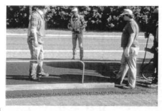
FIGURE 17-8 Checking smoothness at transverse joint.
