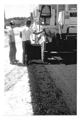
FIGURE 15-19 Difference in texture under strike-off extension.
