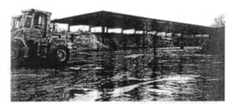
FIGURE 6-1 Covered aggregate stockpiles.
