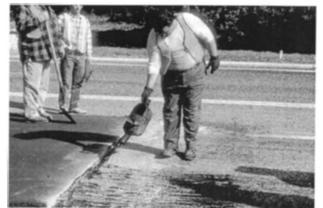
FIGURE 17-3 Application of tack at butt joint.
