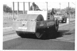
FIGURE 17-10 Longitudinal rolling of transverse joint.
