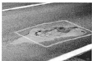
FIGURE 13-7 Pothole caused by overlaying of spilled diesel fuel.
