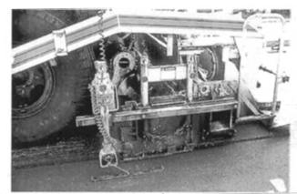
FIGURE 16-9 Operation of joint-matching shoe.
