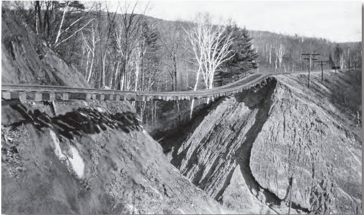
Caving banks undermined a railroad in Vermont, 1927.
