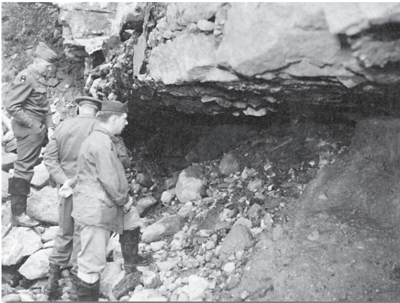
Engineer officers inspected the erosion under the spillway apron of Chittenden Dam after the Rutland, Vermont, flood of June 1947.
