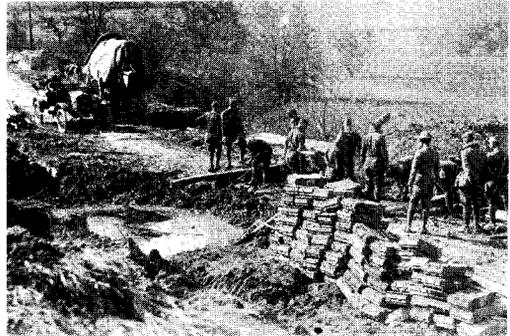
*Another view of road constructed by 4th Engrs night before attack. Used 4,000 sand bags in it.*
