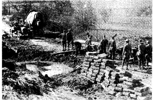
*Another view of road constructed by 4th Engrs night before attack. Used 40,000 sand bags in it.*
