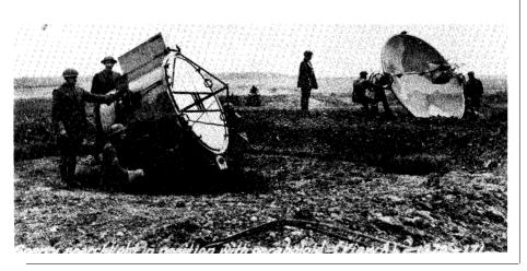
American paraboloid and searchlight in position to track and illuminate attacking enemy aircraft.
