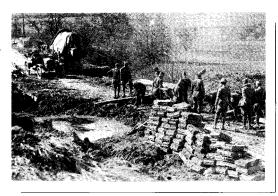
Another view of road constructed by 4th Engra. night before attack. Used 40,000 sand bacs init.
