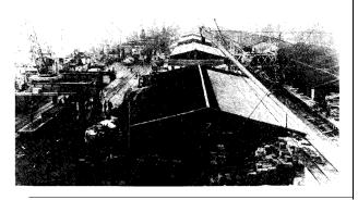
The derricks at this American-built dock at Bassens could lift cargo from ship holds and place it directly in waiting railroad cars.
