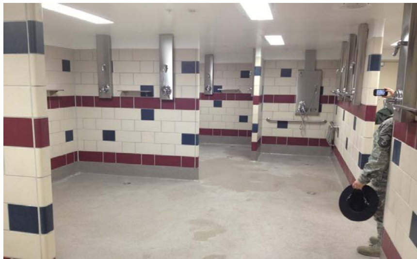
Open Showers at an Air Force Base
