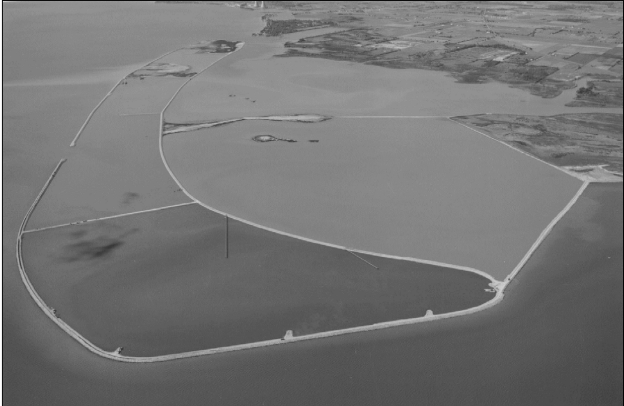
Figure 5-56. Pointe Mouillee, a 1,900 ha CPF for Contaminated Credged Material in Western Lake Erie, also Serves as a Multipurpose Beneficial Use Site
