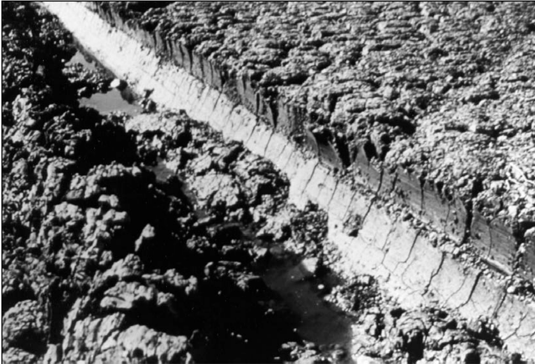
Figure 4-43. Close-Up View of Trenches Formed by a Rotary Trencher
