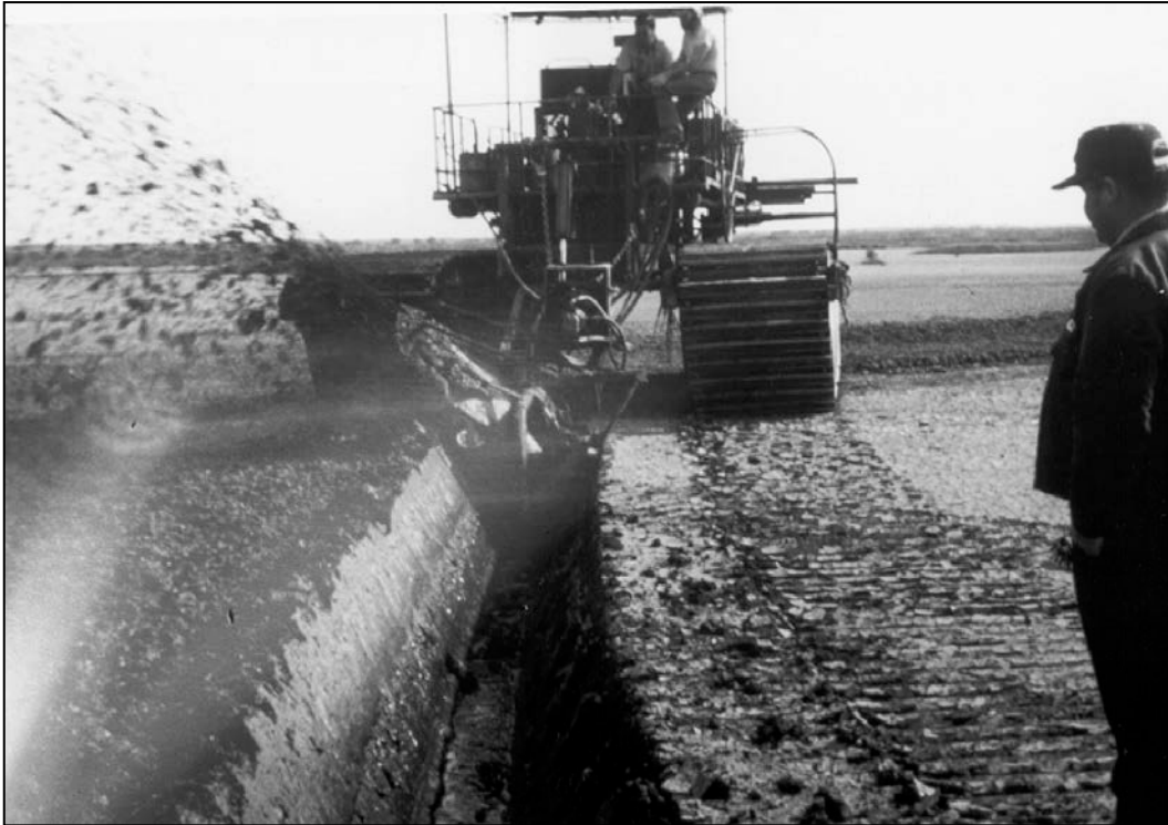
Figure 4-41. Rotary Trenching Device in Operation
