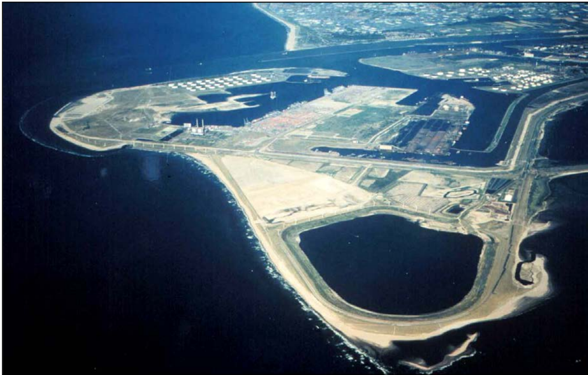
Figure 4-2. Shelfter CDF in Rotterdam, The Netherlands
