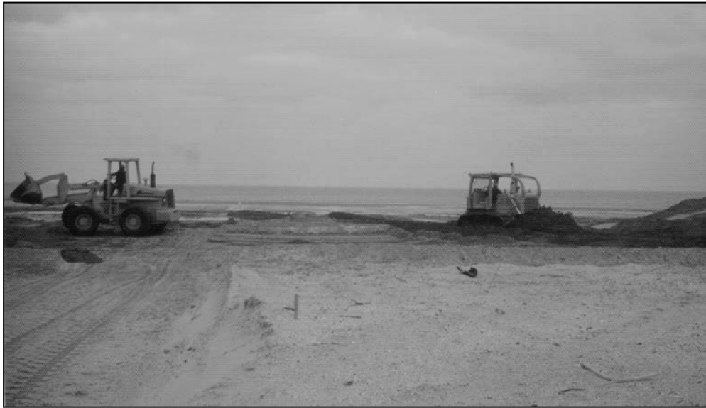
Figure 5-21. Heavy Equipment was Required to Shave Down Sandy Dredged Material Deposits to Intertidal Levels at Bolivar Peninsula, TX, and at Other Man-Made Wetland Sites
