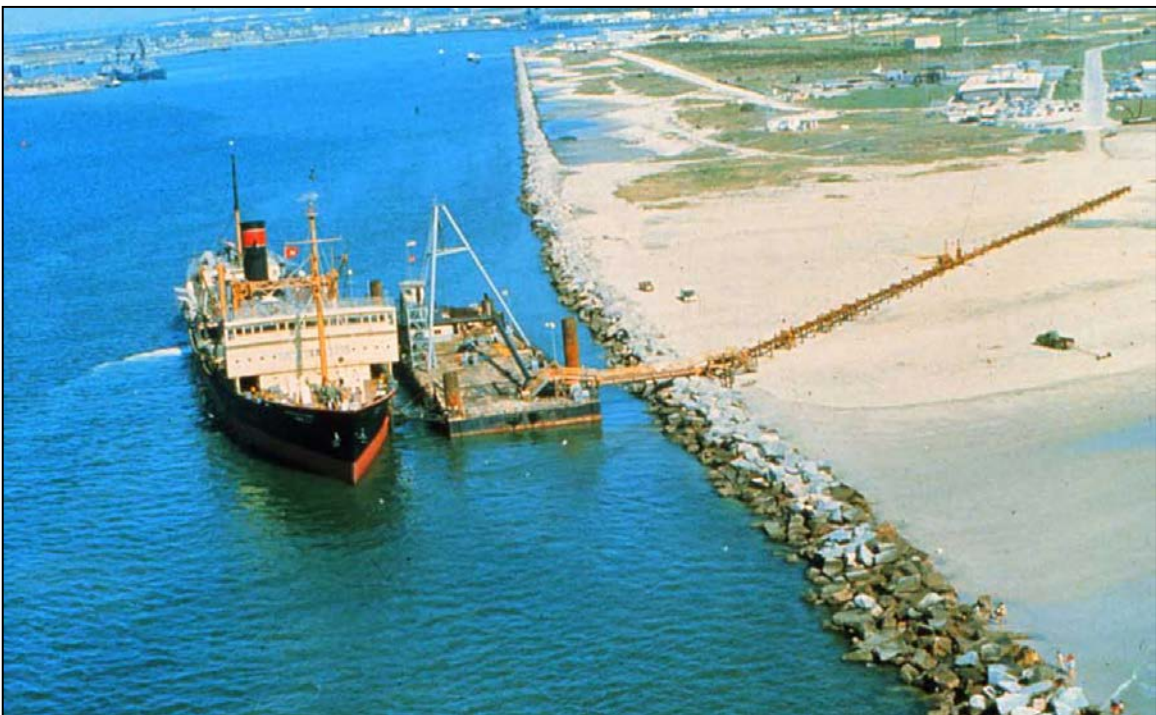
Figure 4-7. Hopper Dredge Pumpout Operation with a Pipeline Leading to the CDF
