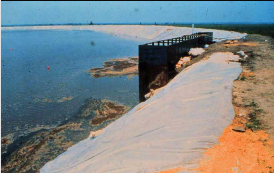
Figure 4-19. Rectangular Weir (1)
