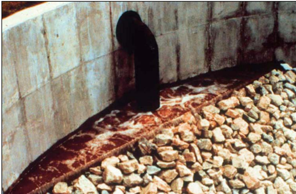
Figure 4-72. Granular Media Filtration
