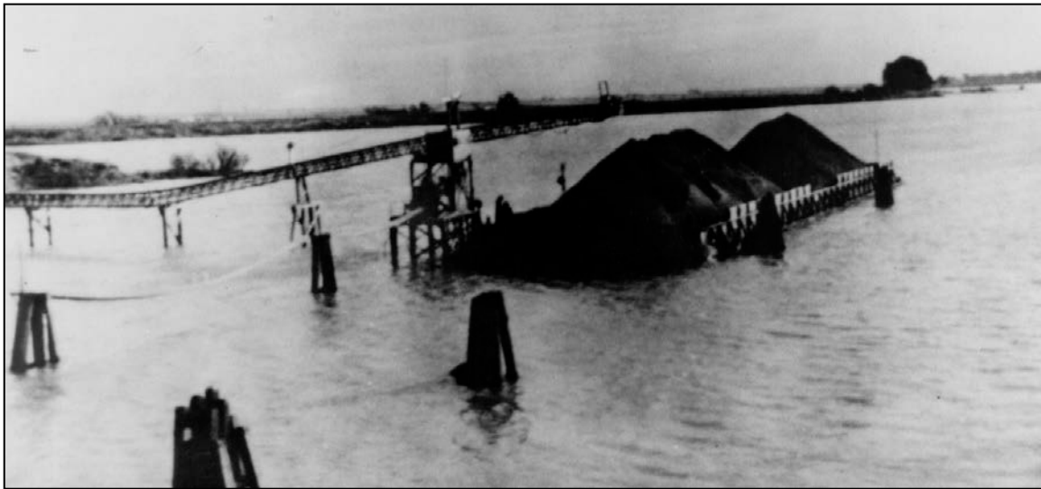
Figure 5-5. A 1 m (3.3 ft) Belt Conveyor Dredged Material Loading Operation
