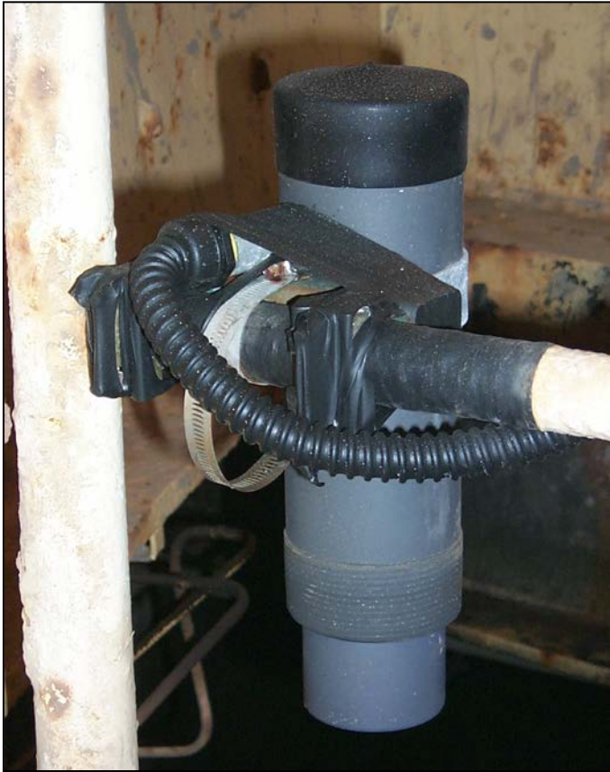
Figure 2-45. Acoustic Hopper Level Sensor
