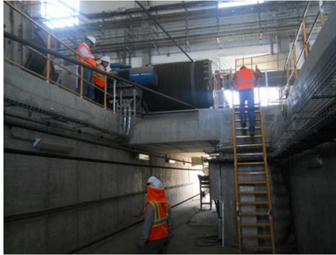
Figure 3-27. Panama Canal – Wire Rope Drum and Guide Rollers.
