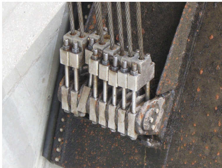
Figure 5-7. Tainter Gate Wire Rope Connection with a Broken Bolt on One Block
