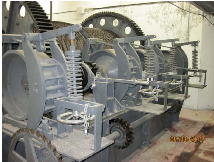
Figure 3-45. Welland Canal Brake System.
