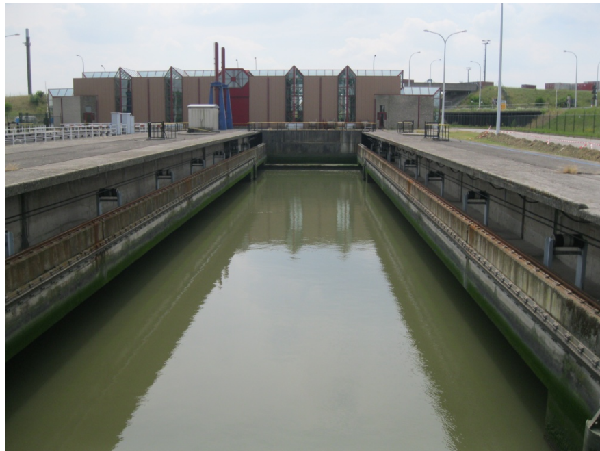
Figure 3-29. Berendrecht Rolling Gate Recess – Note Wire Rope Drives on Each End.
