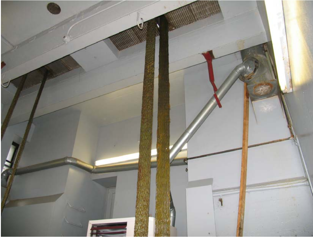
Figure 2-7. Flat Wire Rope at East Branch Lake Dam – PA.
