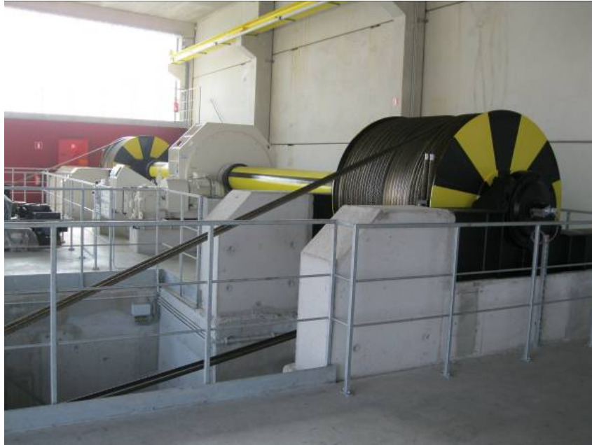
Figure 3-31. Wire Rope Winch Drive – Van Cauwelaert Lock.
