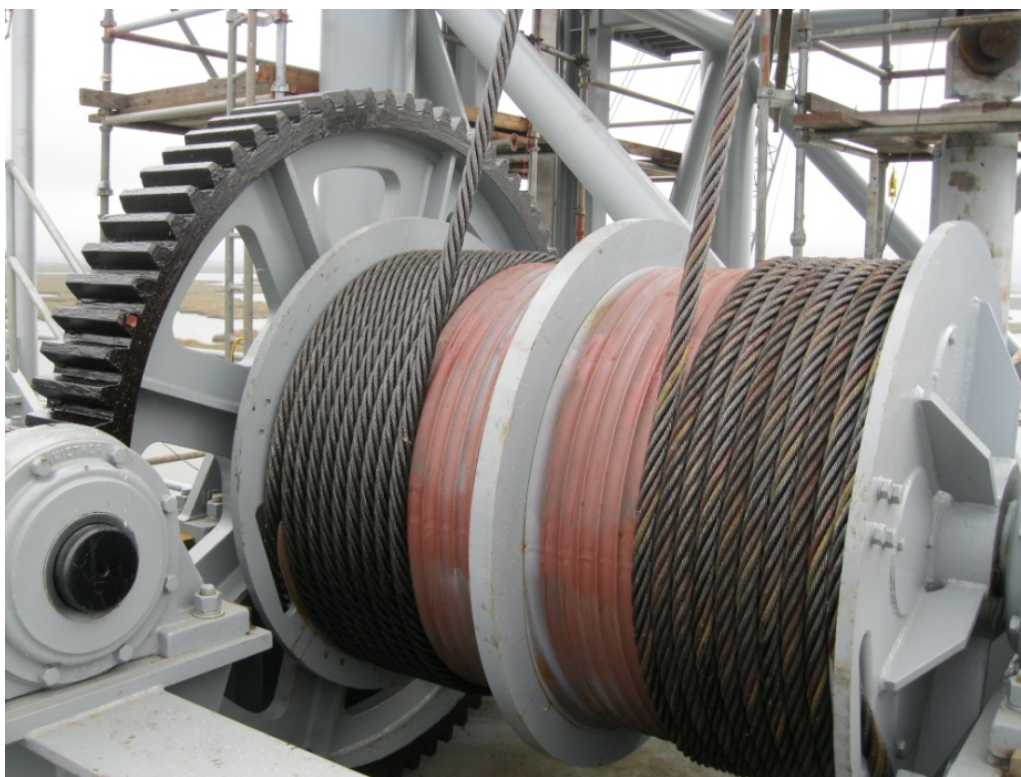
Figure 3-12. Vertical Lift Gate Bayou Bienvenue – Double Cable System – Grooved Drum.
