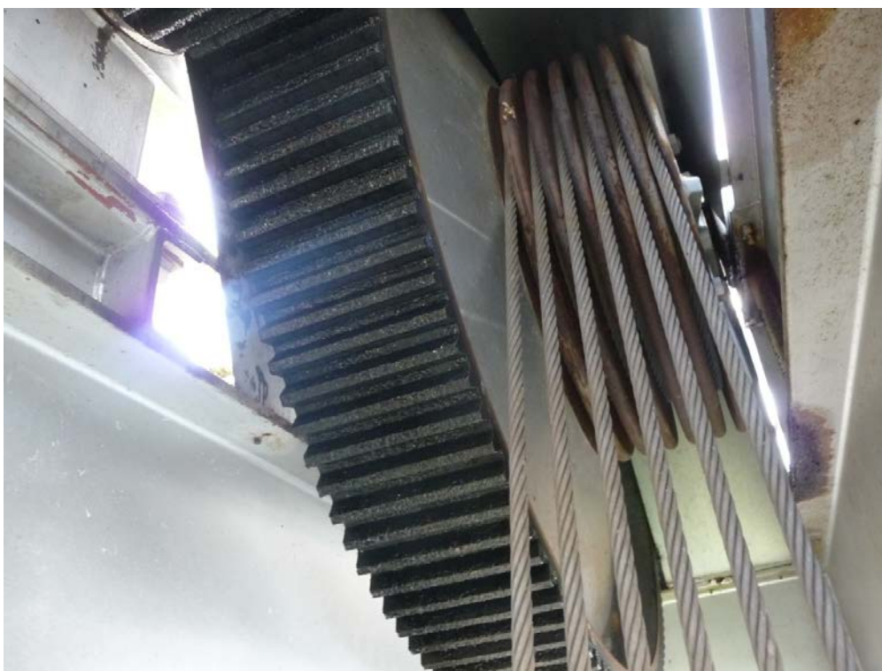
Figure 3-4. Tainter Gate – Multi Part Wire Disc Layered Drum Detail.
