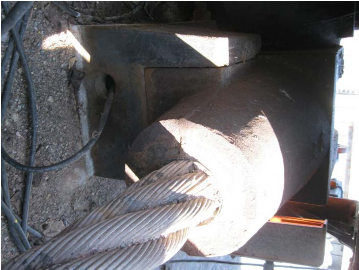
Figure 3-38. Macarthur Lock – 3½-in. Wire Rope Swaged End.
