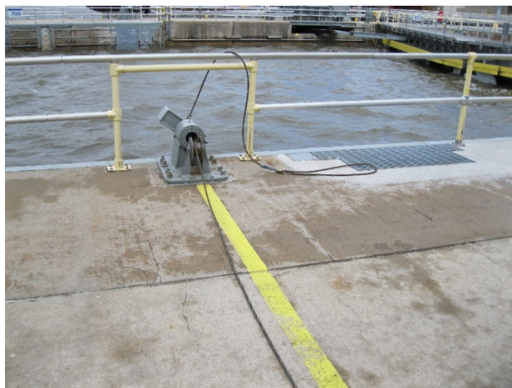
Figure 3-48. Tow Haulage Winch Fairlead.
