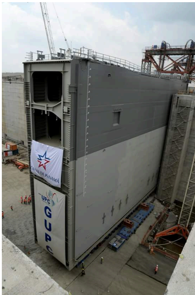
Figure 3-25. Installation of New Panama Canal Rolling Gates.
