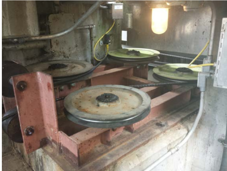
Figure 3-21. Sheaves for Sector Gate Wire Rope Reeving.
