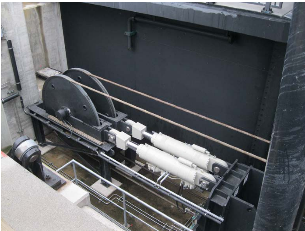
Figure 3-36. Automatic Wire Rope Tensioners – Kaiser Lock.
