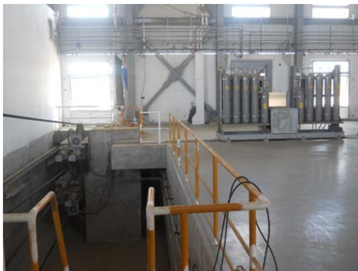
Figure 3-26. Panama Canal – Wire Rope Tensioning System with Nitrogen Tanks in Background.
