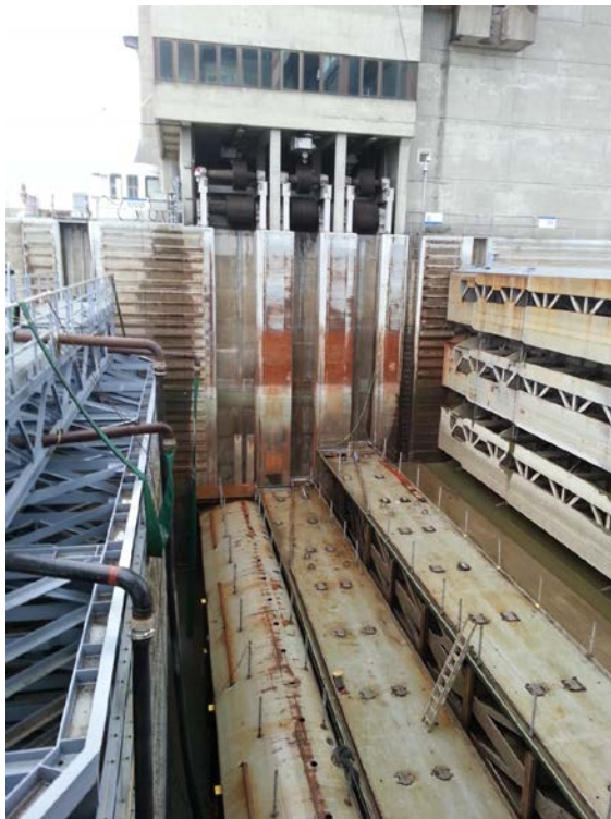
Figure 3-13. Mel Price Vertical Lift Gate – Showing Three Gate Leafs and the Wire Rope Drums in Background.
