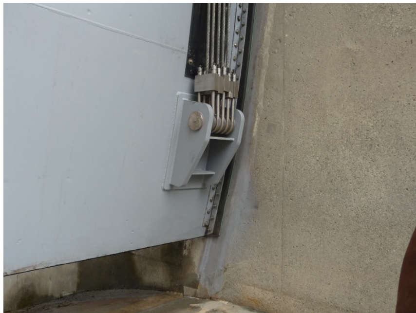
Figure 4-12. U-Bolt Rope Tensioning System on a Spillway Tainter Gate.
