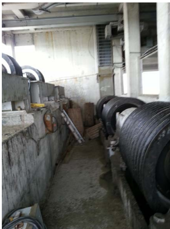
Figure 3-14. Mel Price Vertical Lift Gate Machinery and Hoist Drums.
