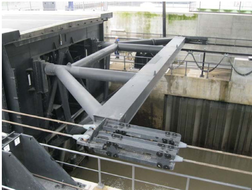
Figure 3-34. Wire Rope Connection to Gate.
