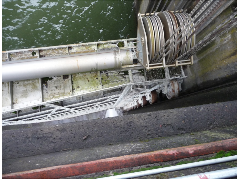
Figure 4-6. Gate Hoist Sheave Block System.
