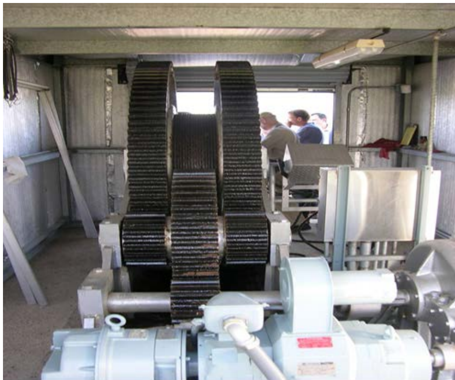
Figure 3-52. Bulkhead Lifting Machinery Port Allen Lock.
