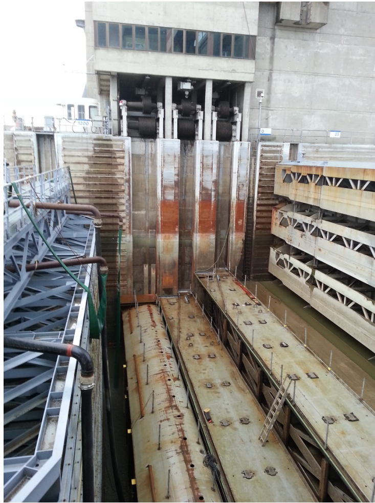
Figure B-1. Vertical Gate Leafs with Hoist Drums in Background.
