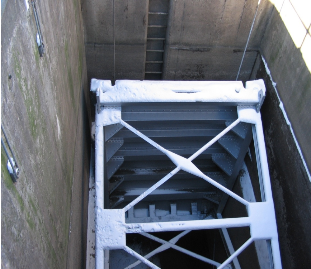
Figure 3-7. Wire Rope Connection to Tainter Valve.
