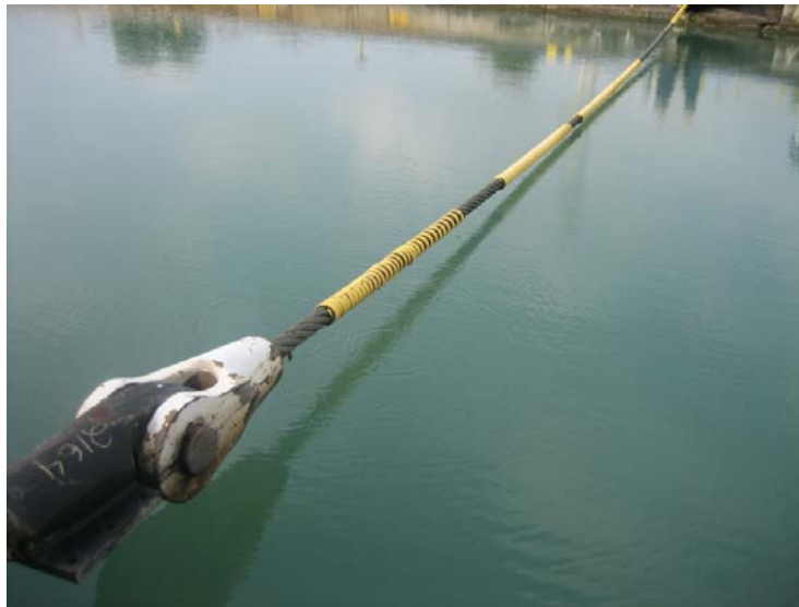
Figure 3-43. Welland Canal Ship Arrestor – Free Boom Type in Place.
