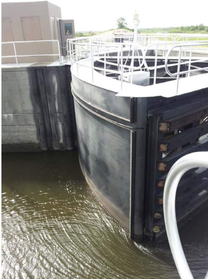
Figure 3-22. New Orleans Bayou Bienvenue Sector Gate – Wire Rope Driven.
