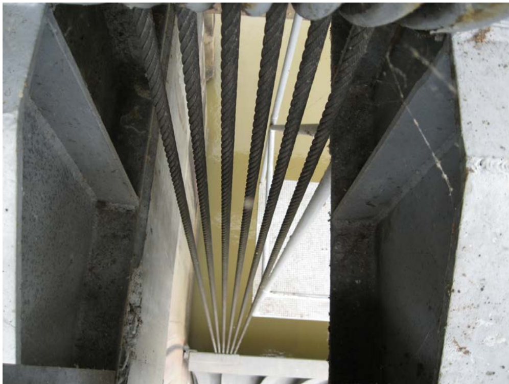
Figure 3-3. Tainter Gate Wire Rope Detail – Disc Layered Drum.
