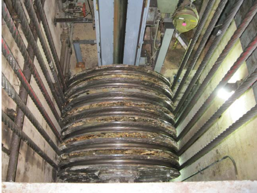
Figure 8-8. Wire Rope Cable Sheaves – Lockport.
