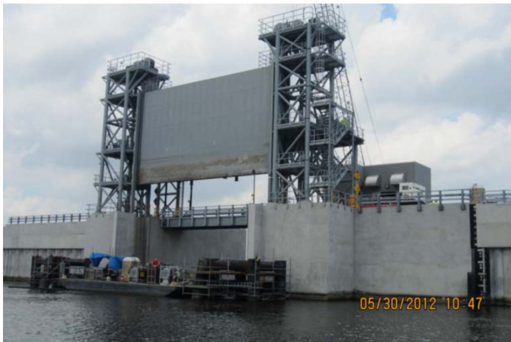
Figure 3-11. New Orleans Surge Barrier – Bayou Bienvenue – Vertical Lift Gate Hoisting System and Lifting Towers.
