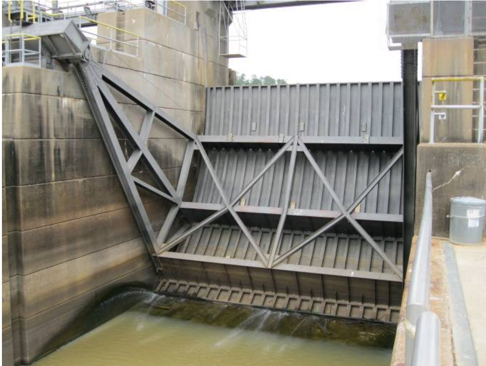
Figure 3-1. Tainter Gate Structure Lifted with Wire Rope.
