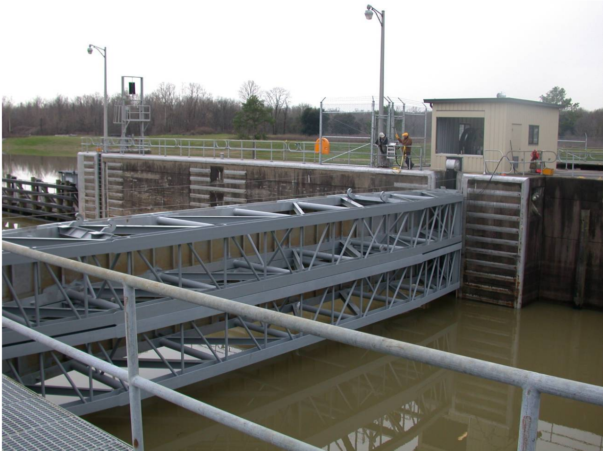
Figure 3-49. View of Two Existing Bulkheads Stacked on the Lowering Carriage.
