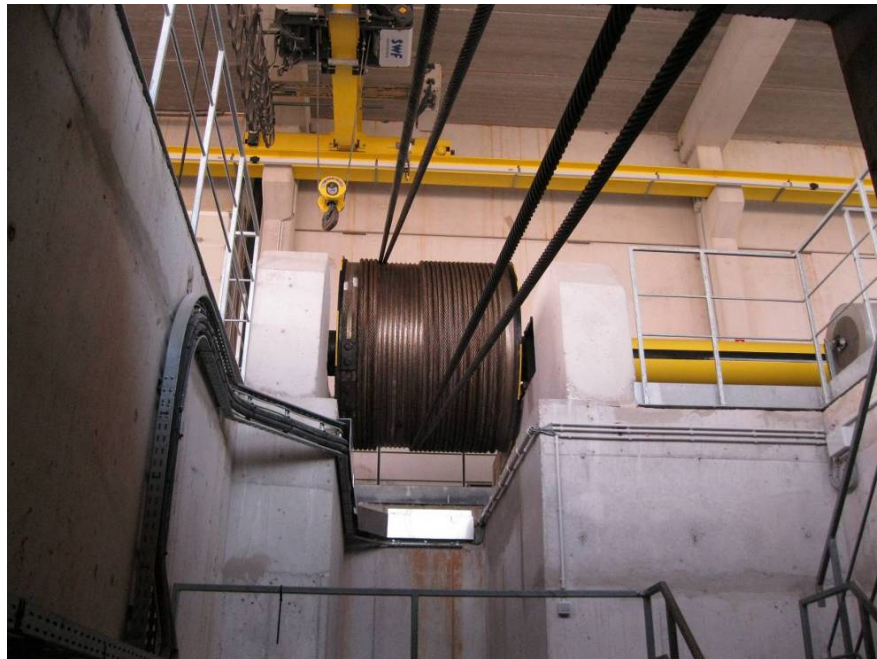
Figure 3-32. Winch Drum and Cables – Van Cauwelaert Lock.
