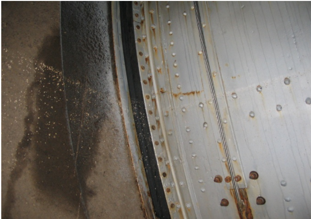
Figure 3-8. Wire Rope Connection to Tainter Valve.
