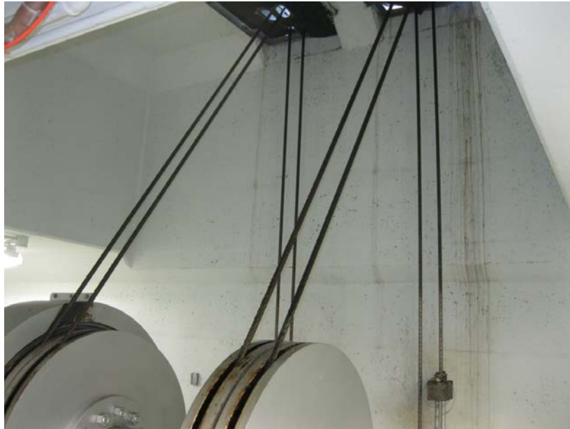
Figure 3-54. Bulkhead Winch Cable System – Bonneville Lock.
