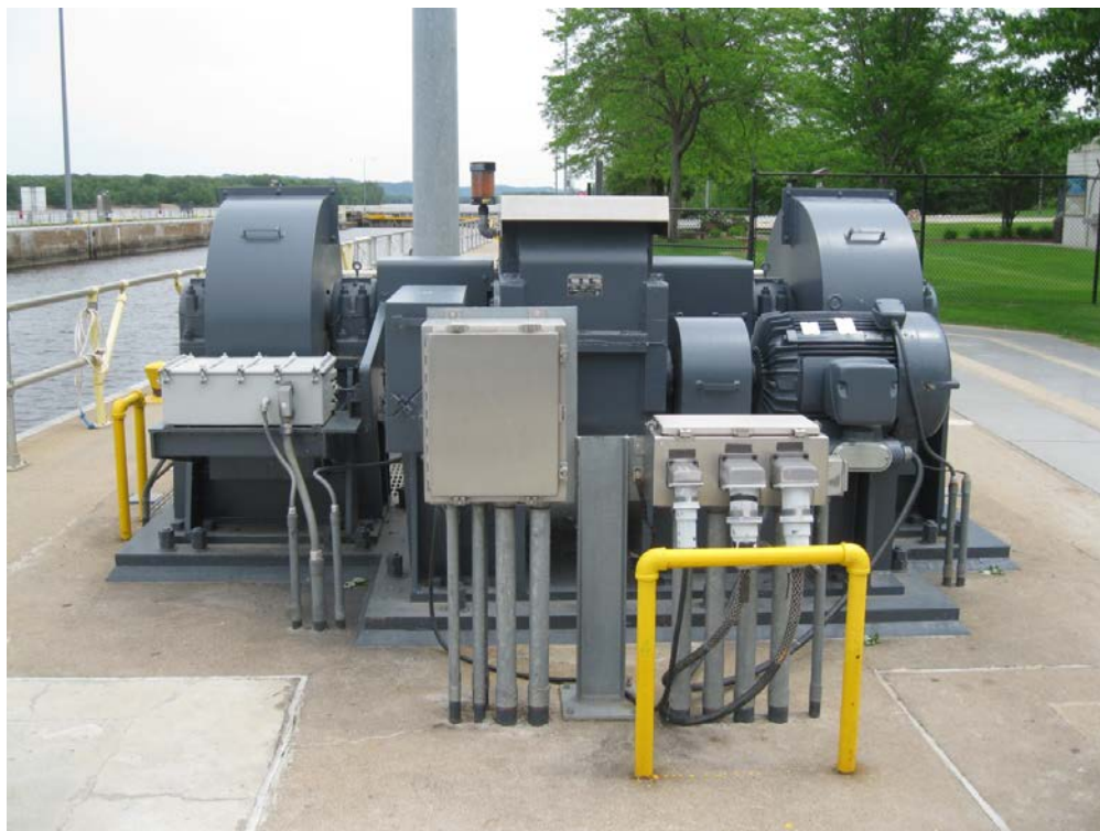
Figure 3-5. Tainter Valve Drive System with Wire Rope Drums on Each End.
