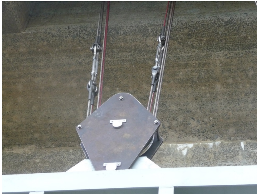
Figure 4-11. Turnbuckle Rope Tensioning System.
