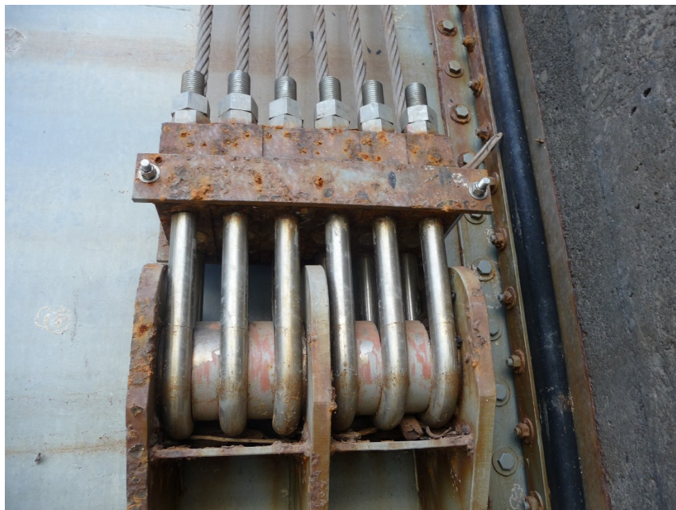
Figure 7-3. Tainter Gate Wire Rope U-Bolt Connection.
