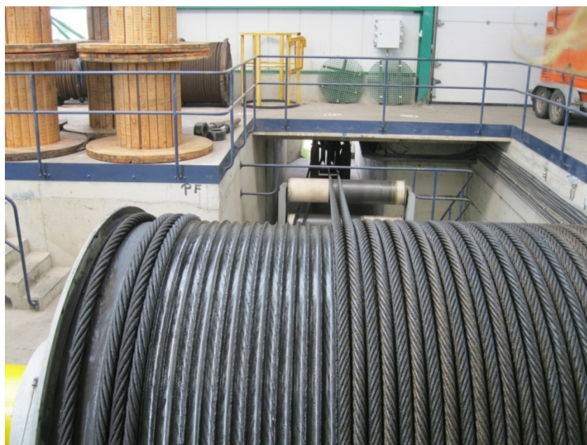
Figure 3-30. Wire Rope Drum – Berendrecht Lock.
