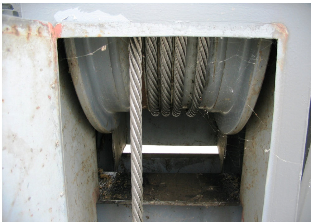
Figure 3-6. Tainter Valve Lifting Cable and Drum.
