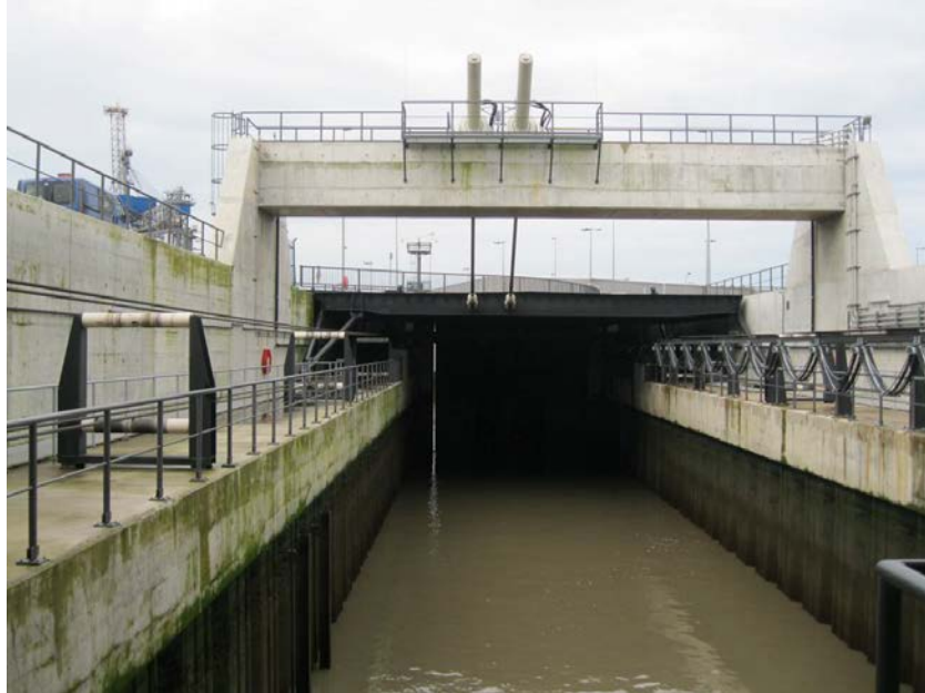
Figure 3-33. Rolling Gate Recess and Wire Rope Cables – Note the Guide Rollers.
