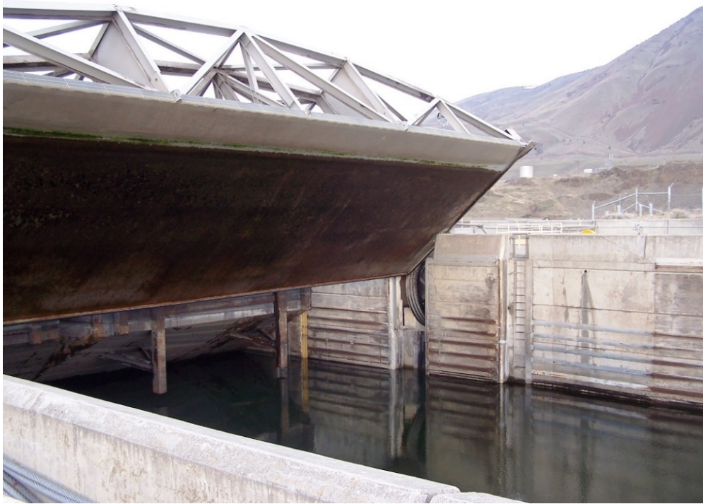
Figure B-7. John Day Lock Upstream Gate after 2008 Accident.
