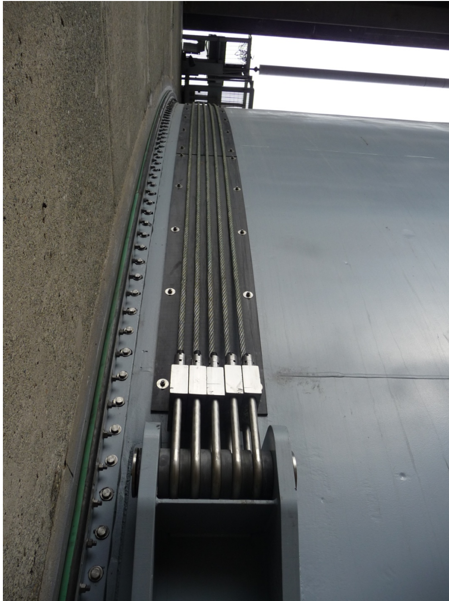
Figure 4-14. UHMW-PE Wire Rope Wear Plates.
