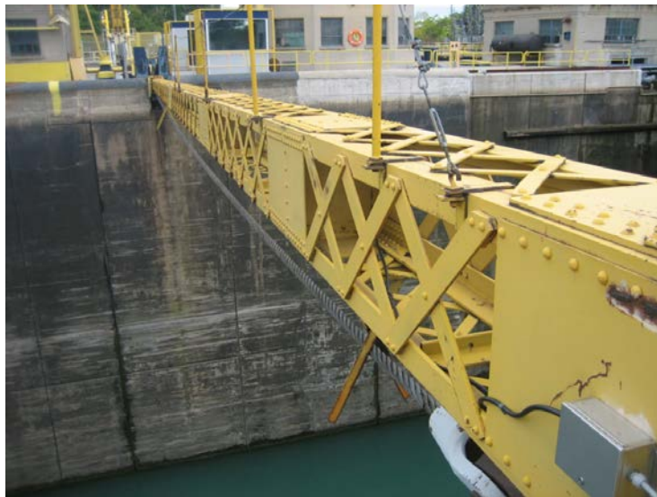
Figure 3-44. Welland Canal Fixed Boom Type (Similar to Soo Locks).
