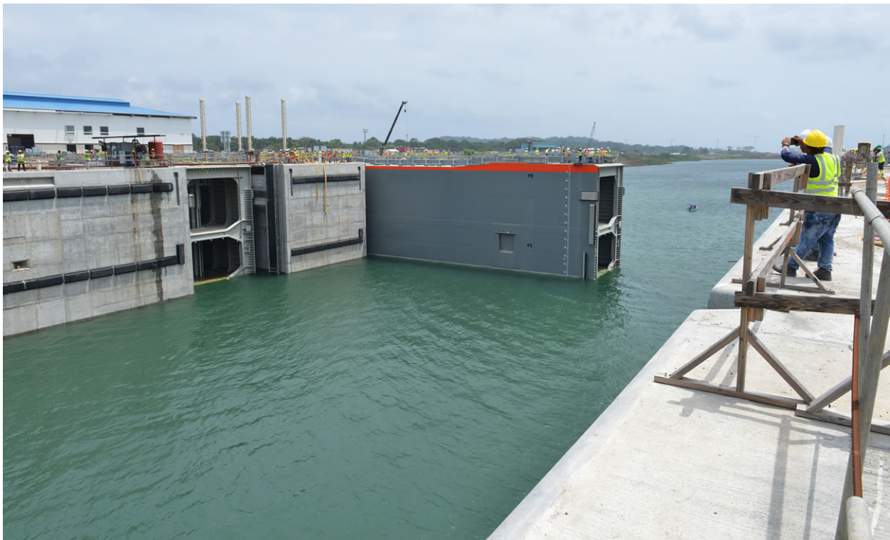
Figure 3-24. Redundant Rolling Gates – Panama Canal Third Lane (Courtesy ACP).
