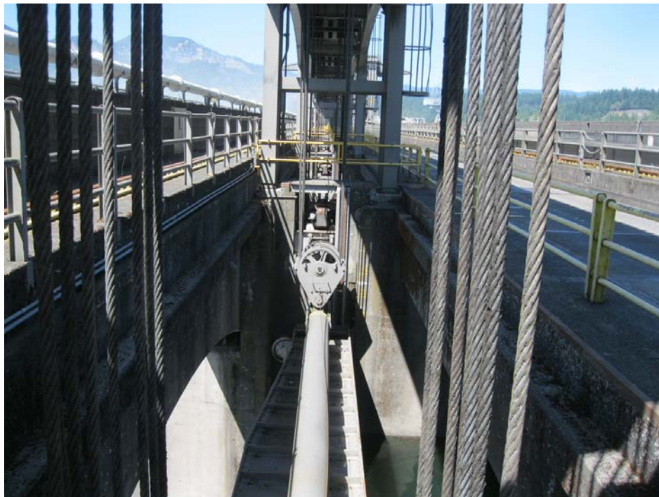
Figure 3-9. Bonneville Dam Wire Rope Lifting System.
