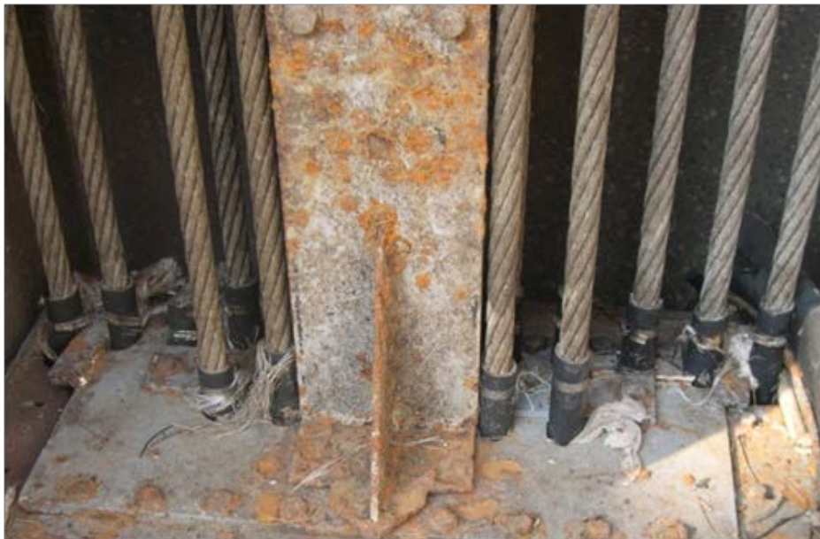
Figure B-3. View of Cable/Socket Connection to Gate Leaf from Top of the Leaf Looking into the Slot.
