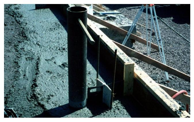
Figure 6-5. Installation of waterstop, joint drain, and crack initiator
