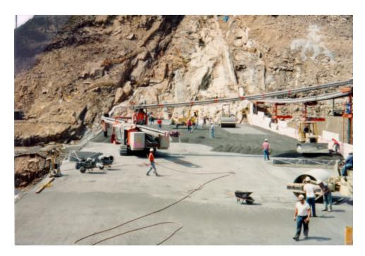
Figure 6-1. Conveyor system with self-propelled crawler-placer
