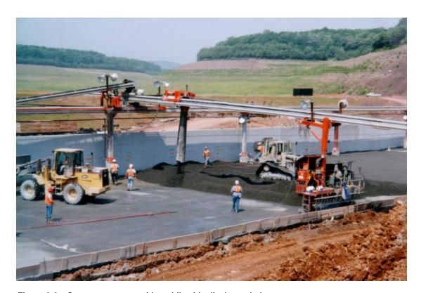
Figure 6-2. Conveyor system with mobile side discharge belt
