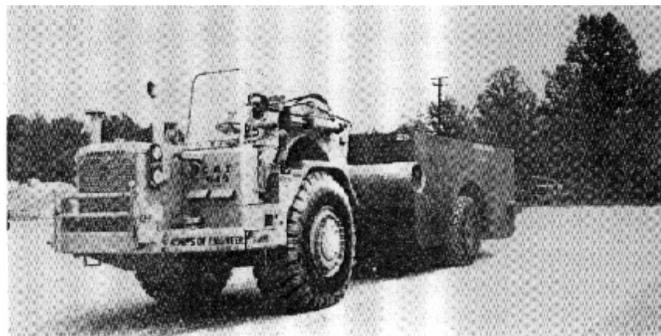
Figure 5-2. Rubber-tired roller
