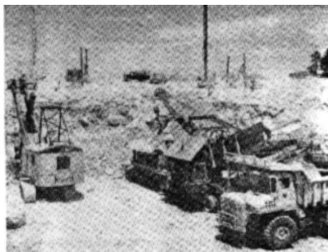
Figure 4-7. Grizzly wobbler discharging +2-in. rock into end-dump truck and -2-in. material into bottom-dump truck (spillway-powerhouse excavation at Stockton Lake Dam, Missouri)
