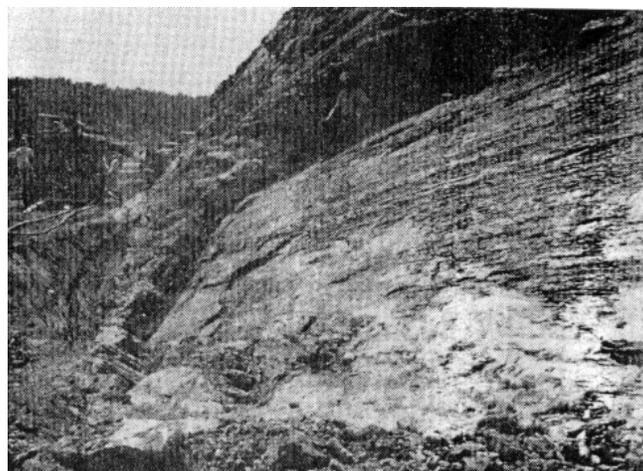
**Figure 3-7. Abutment overhang, DeGray Dam, Arkansas**
