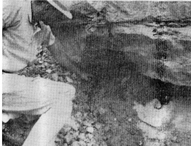
**Figure 3-10. Seepage from spring in abutment at Green River Dam, Kentucky**
