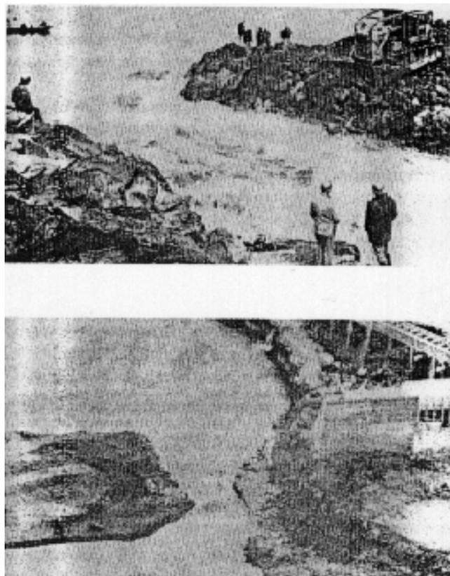
**Figure 6-1. Examples of end fill closure method. (a) River closure, cofferdam, Mica Dam, British Columbia; (b) two days before final closure, Dalles Closure Dam, Columbia River**
