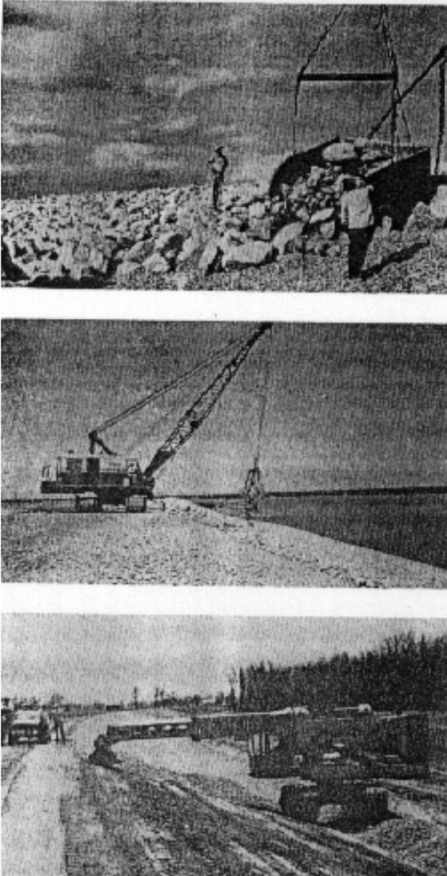
**Figure 5-16. Placement of riprap and bedding material. (a) Dragline with skip placing riprap at Texarkana Dam, Texas; (b) Dragline with orange peel attachment placing riprap at Lavon Dam, Texas; (c) Gradall used to place bedding material, main stem levee, Chariton River Project, Missouri**
