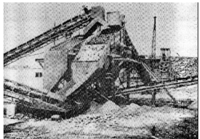
Figure 4-5. Vibrating screen separating plant
