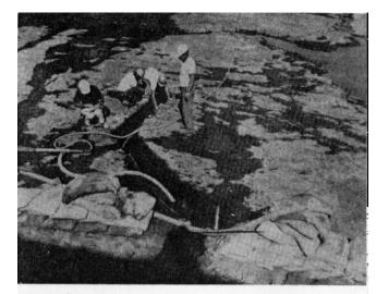
a. Drainage trench dug along water-producing crack in shale
