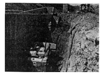
Figure 5-13. Placement of pervious material adjacent to stilling basin wall, Brookville Dam
