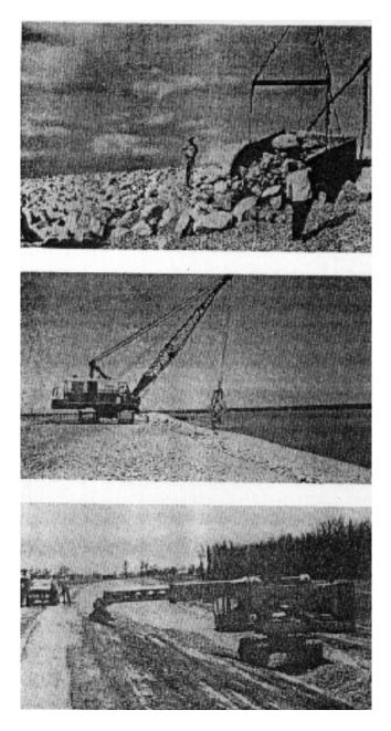
Figure 5-16. Placement of riprap and bedding material. (a) Dragline with skip placing riprap at Texarkana Dam, Texas; (b) Dragline with orange peel attachment placing riprap at Lavon Dam, Texas; (c) Gradall used to place bedding material, main stem levee, Chariton River Project, Missouri
