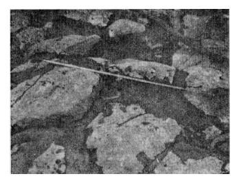
Figure 3-5. Mortar-treated rock surface
