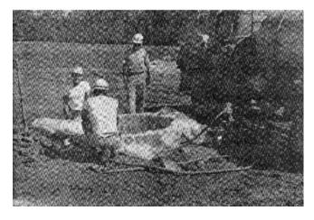
Figure 5-8. Large-scale water displacement density test in progress at New Hope Dam, North Carolina
