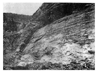
Figure 3-7. Abutment overhang, DeGray Dam, Arkansas
