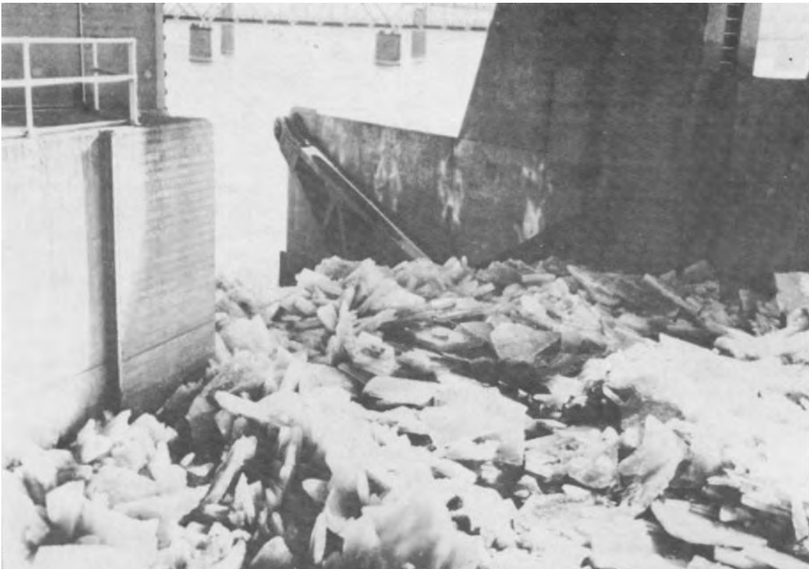
Figure 5-23. Ice on control gate
