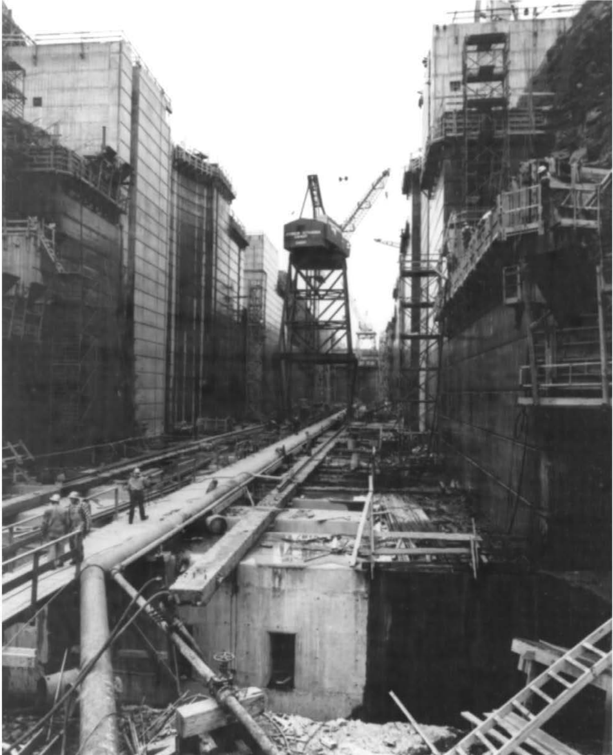
Figure 2-3. Lock with thin walls. The Dalles Lock, Columbia River, with design lift = 88 ft (under construction)
