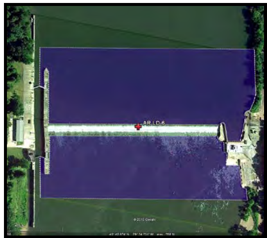
AR Lock & Dam # 6 Survey Coverage Area
