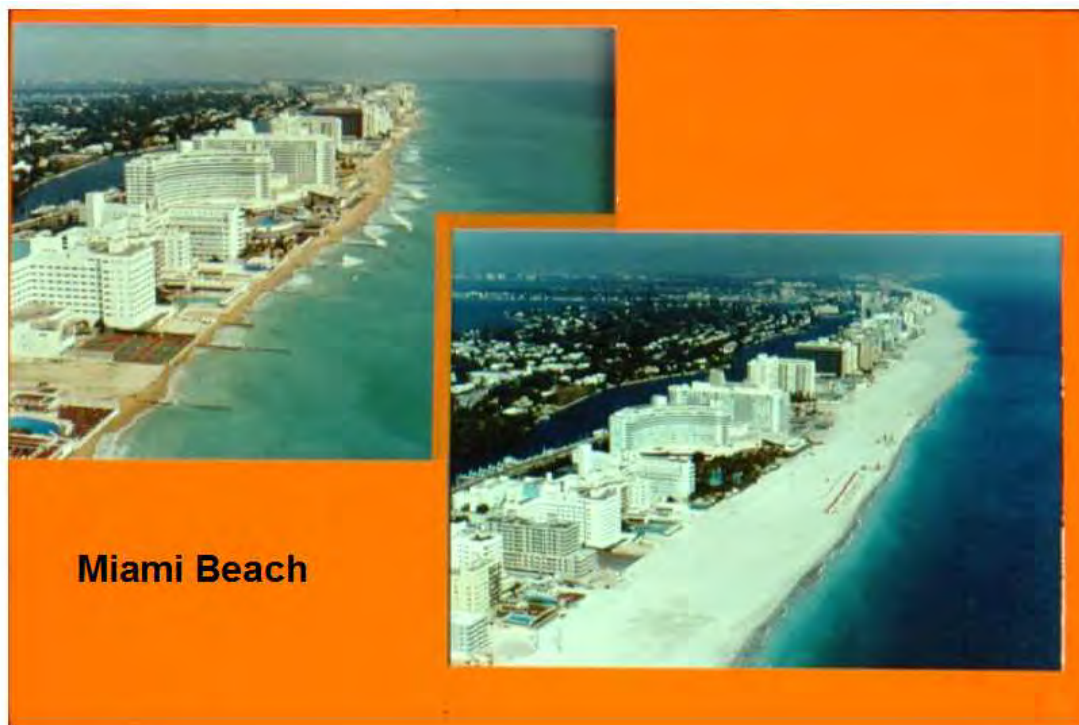
Figure 11-25. Beach renourishment project ca 1975--Miami Beach, FL (Jacksonville District).
