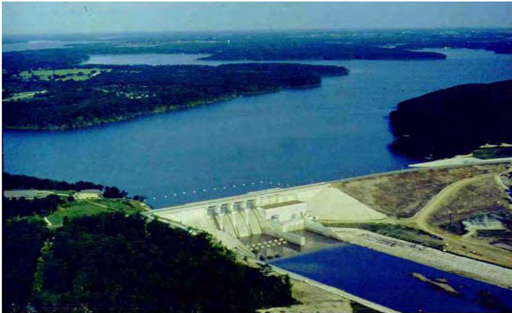
Figure 9-15. Reservoir behind Clarence Cannon Hydropower Dam and Mark Twain Lake, Missouri. (St. Louis District)
