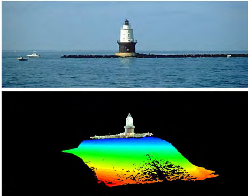
Figure 11-21. Combined terrestrial laser scanner with multibeam hydrographic surveys of Harbor of Refuge Light - Lower Delaware Bay. (Philadelphia District)
