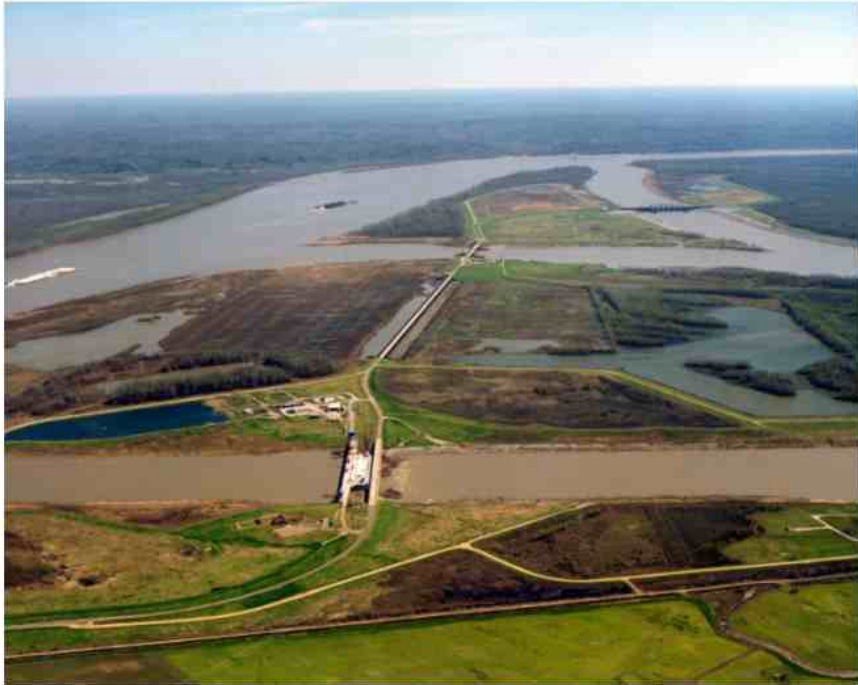
Figure N-17. Old River Control Structures—surveys were performed at the Low Sill Structure. (New Orleans District)
