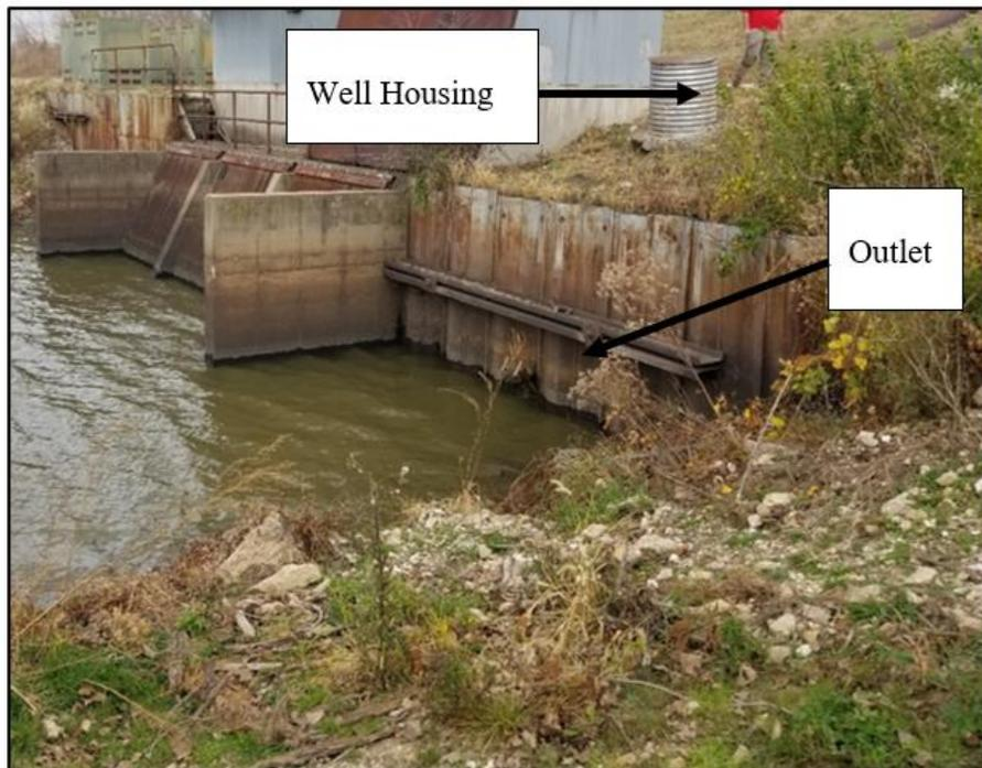
**Figure 10–3. T-type relief well (South River Drainage District)
