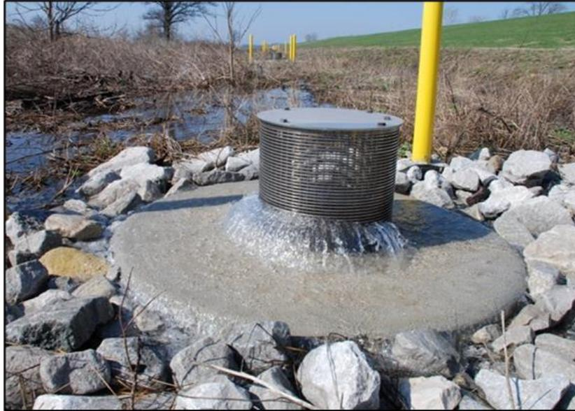
Figure 10–1. D-type relief well reach (photo courtesy of Memphis District)
