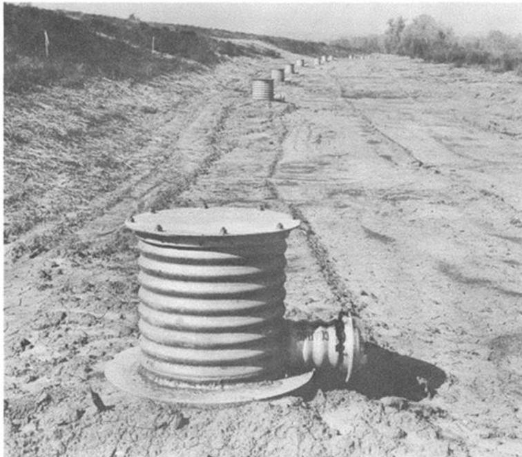
**Figure 1–3. Line of wells at Upper Wood River Levee District (USACE 1956b)**
