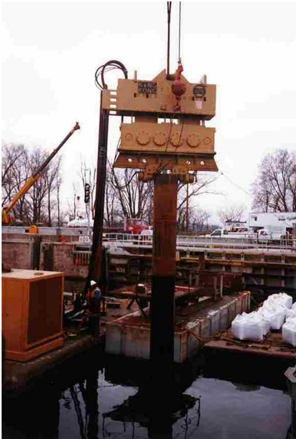
Figure 69. Driving 30-inch diameter steel casing inside lock chamber with vibratory pile hammer for installation of 16-inch diameter pressure relief wells at Lock and Dam 25, Mississippi River, Winfield, MO (Courtesy of AECOM, St Louis, MO, 1998)
