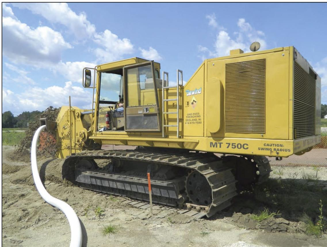
Figure 18. Trencher installing sock-encased 5-inch diameter extra-heavy perforated corrugated HDPE pipe 20 feet deep (Courtesy of DeWind Trenching)
