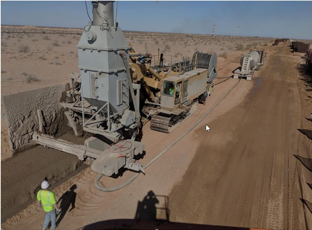
Figure 24. Trencher installing mixed-in-place cutoff wall (Courtesy of DeWind Trenching)
