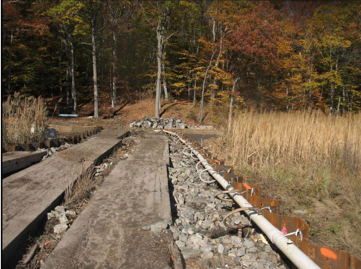
Figure 7. Typical wellpoint system (Courtesy of Keller)
