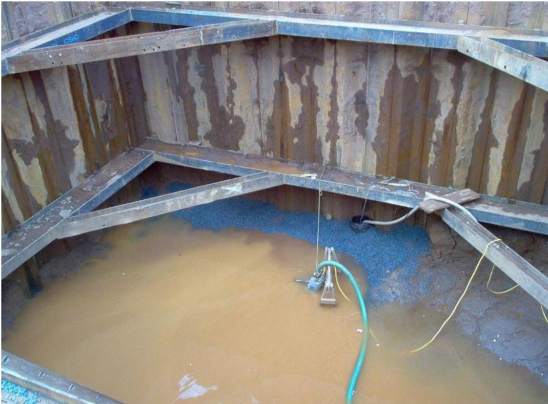
Figure 5. Improperly constructed sump (Courtesy of Keller)
