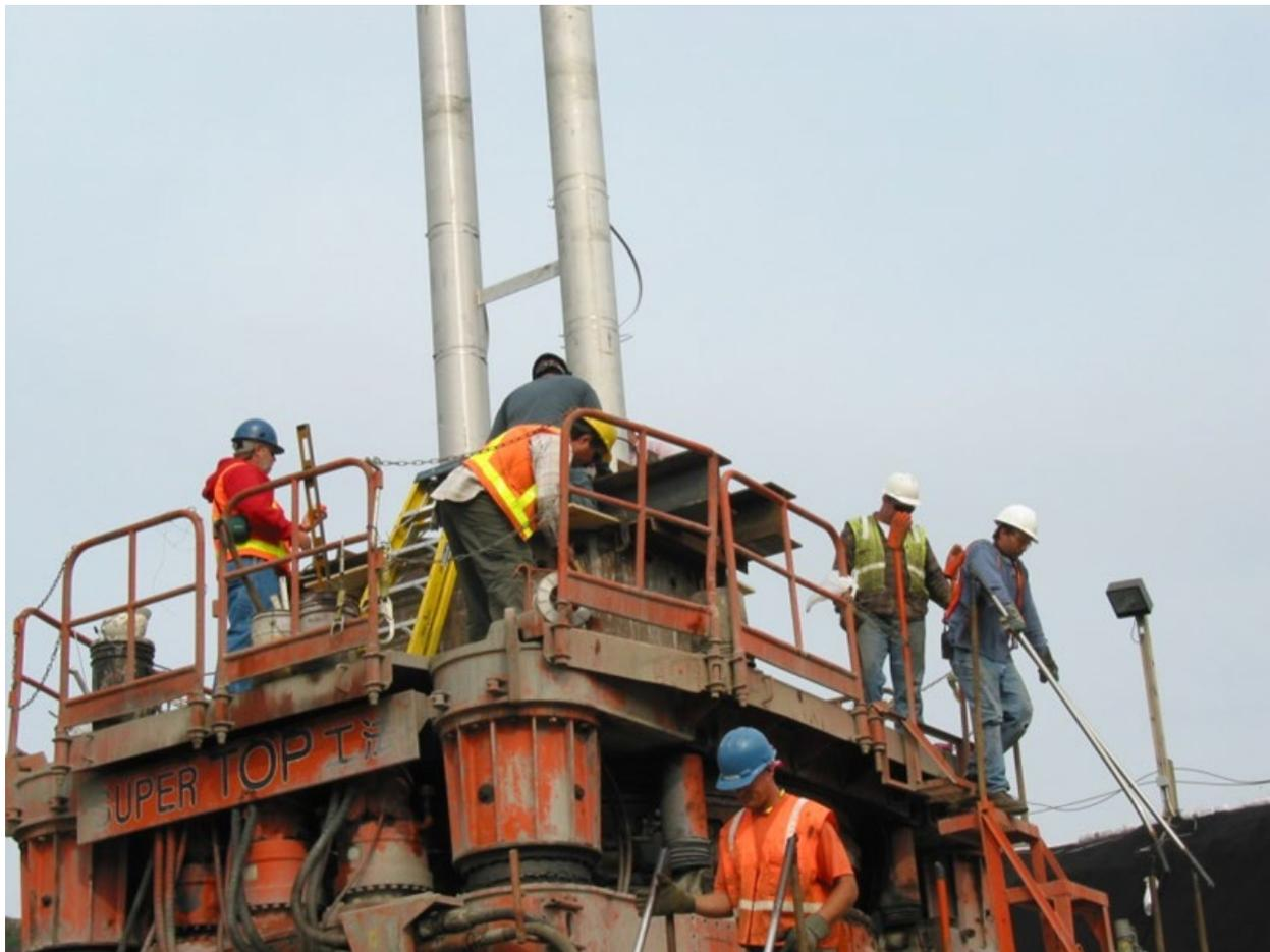
Figure 70. Setting two 12-inch drainage wells into 6.5-foot diameter steel casing installed with Nippon Sharyo SuperTop™ casing rotator at Waterbury Dam, Vermont (October 2004, photograph by Baltimore District, US Army Corps of Engineers)
