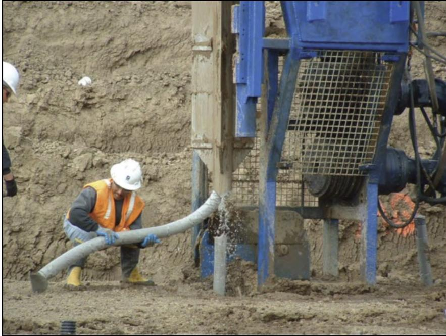
Figure 20. Installing 3-inch diameter drain using hollow tube advanced with vibratory hammer. Primary purpose of this drain was for rapid dissipation of excess pore pressures during an earthquake. (Courtesy of Keller)
