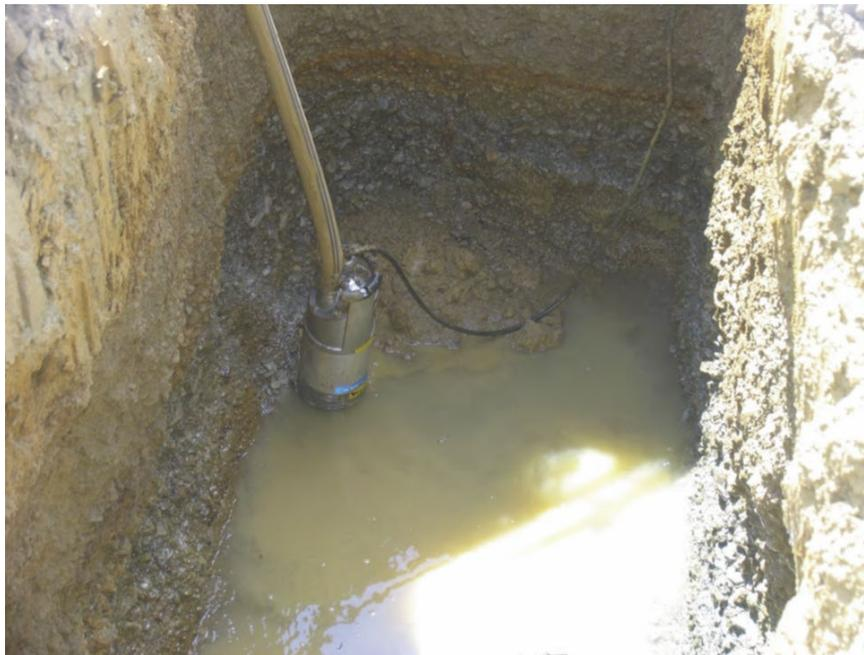
Figure 3. Use of 2-inch submersible pump to dewater localized gravel pocket at downstream toe of an existing earth dam in preparation for a larger excavation to construct an aggregate drain along the toe (Lake Oneida Dam, Butler County, Pennsylvania, Courtesy of Keller)
