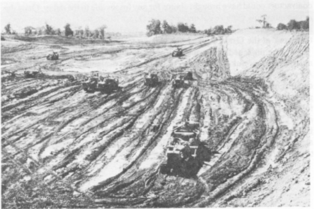
Model B. Scrapers doing early excavation, September 1955.
