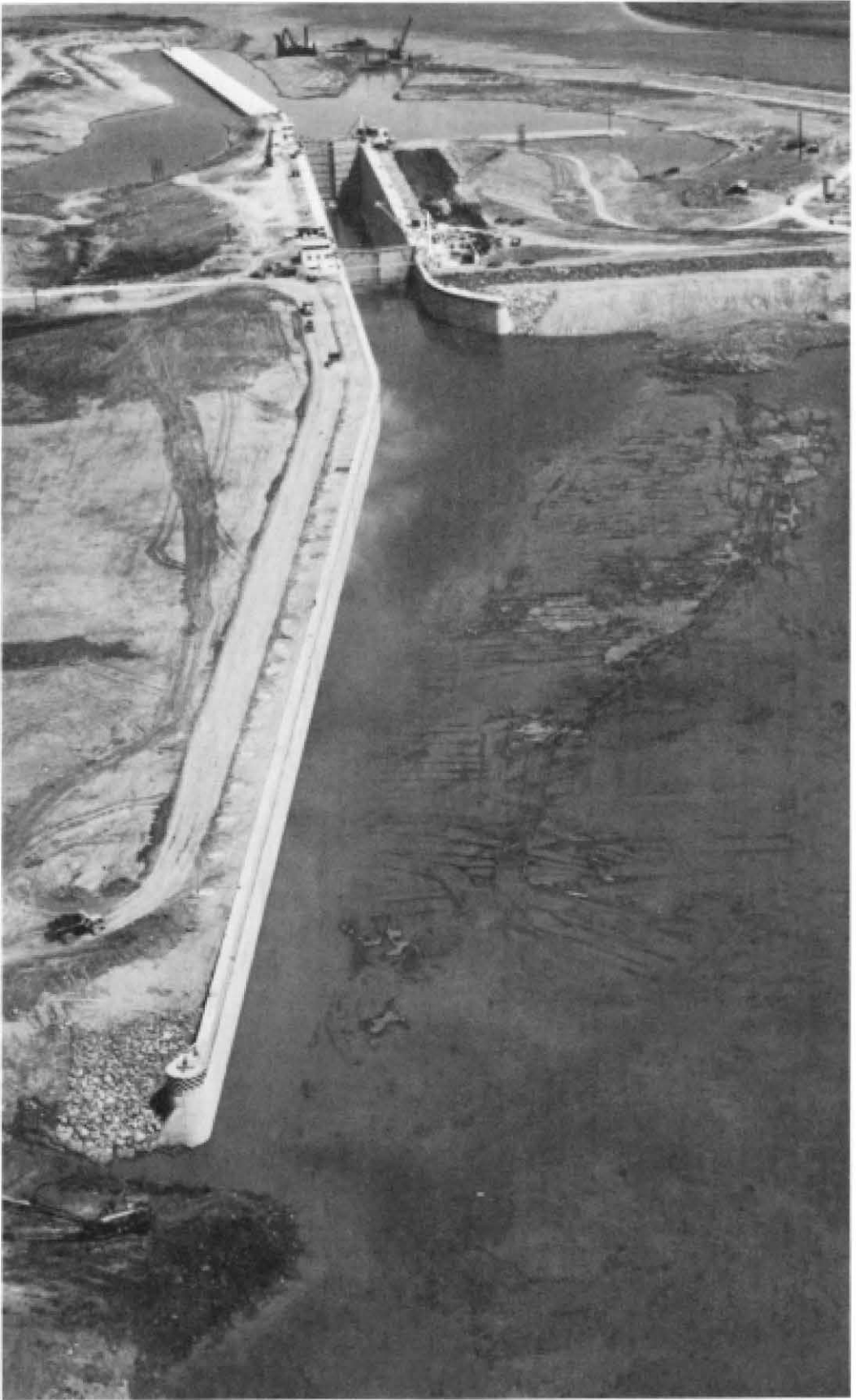
Removing the plugs, May 1958.
