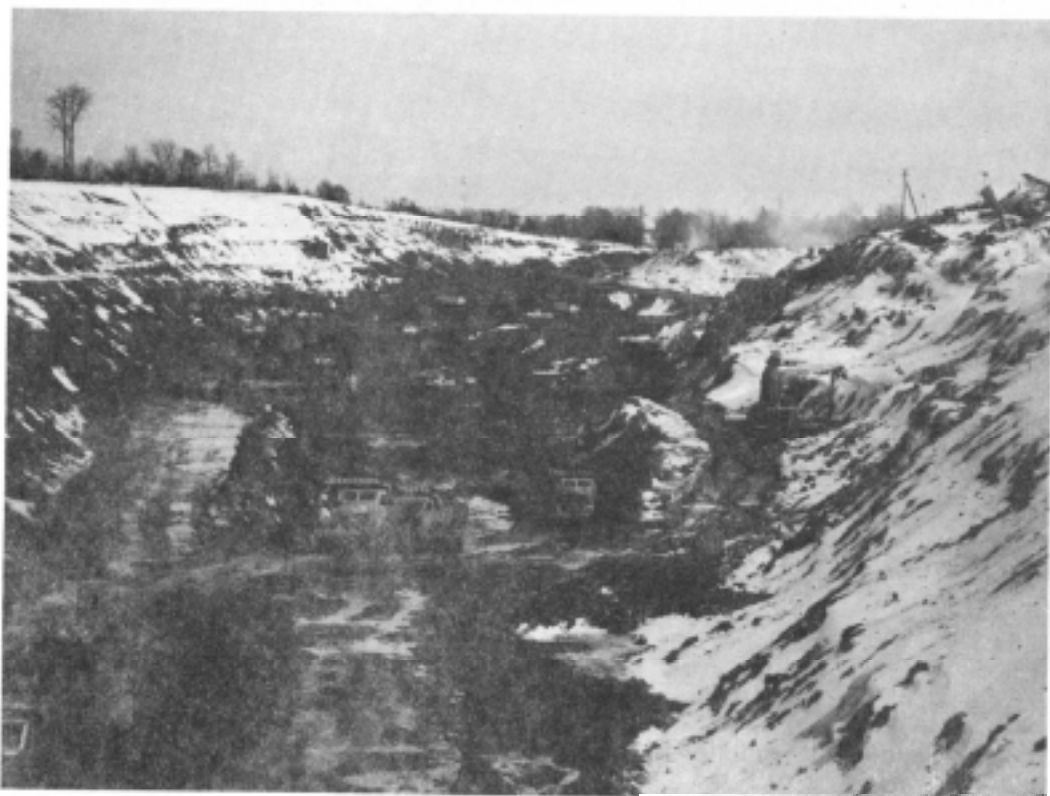
Construction traffic during the excavation, February 1956.
