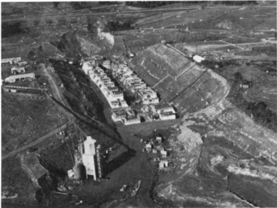
Lock and related construction activity, September 1956.
