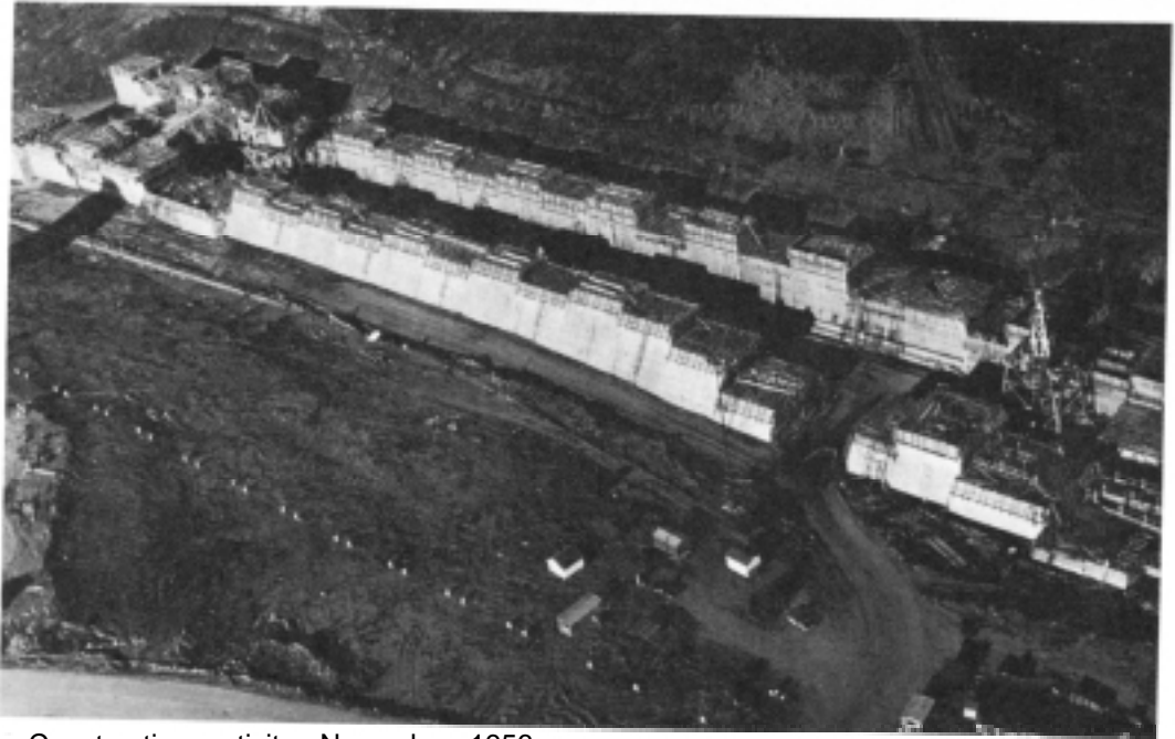
Construction activity, November 1956.
