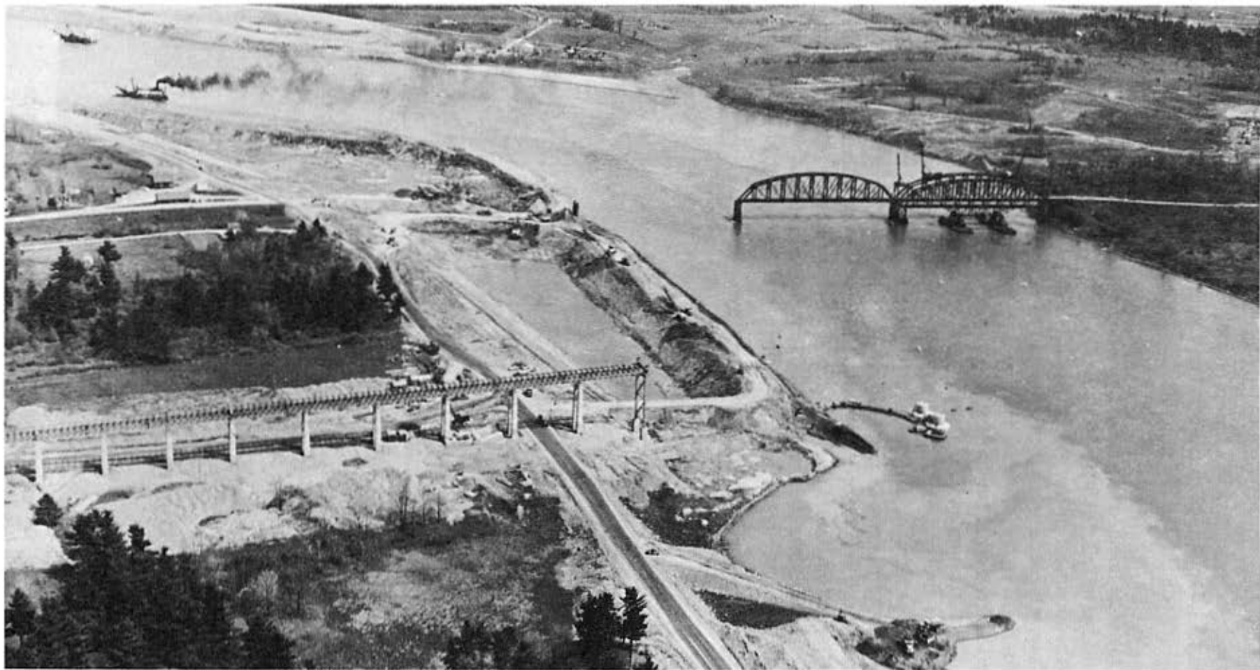
The partially removed Roosevelt Bridge, May 1958. Its north span rests on temporary piers. Also shown is the excavation on Cornwall Island and the partially built high-level bridge.
