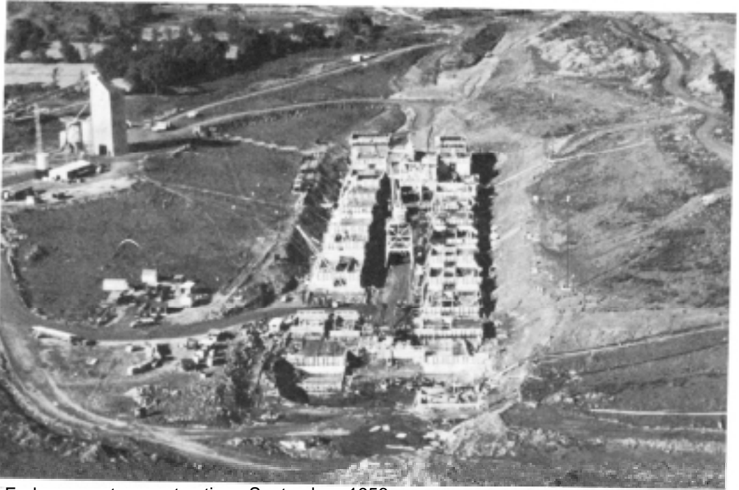
↑ Early concrete construction, September 1956.
