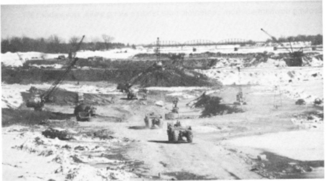
Excavation, February 1956. Glacial till in foreground, marine clay in background.
