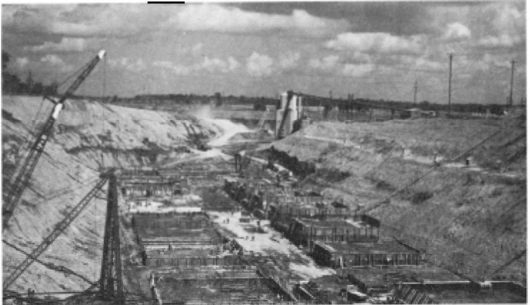
Construction, looking eastward, August 1956.
