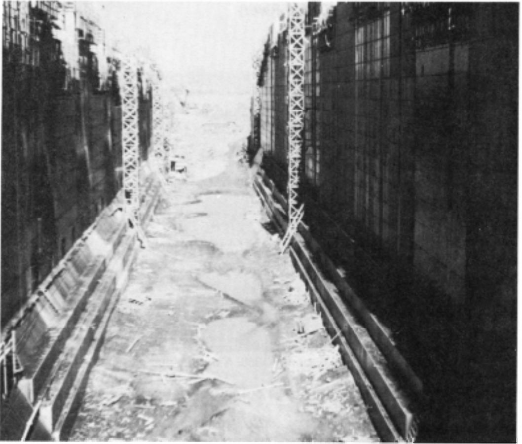
Looking downstream from centerline; note fenders along walls, November 1957.
