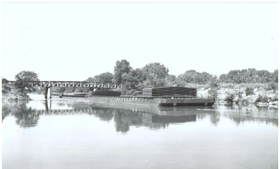
Figure 36. Calumet-Sag Channel before improvements, 1955. Typical fixed bridge with limited clearance of fourteen feet at low water. (NCD Files)
