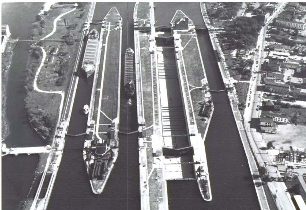
Figure 35. St. Marys Falls Canal, Sault Ste. Marie, Michigan, September 30, 1968. Aerial view looking east, showing New Poe Lock in unwatered condition. (Detroit District)
