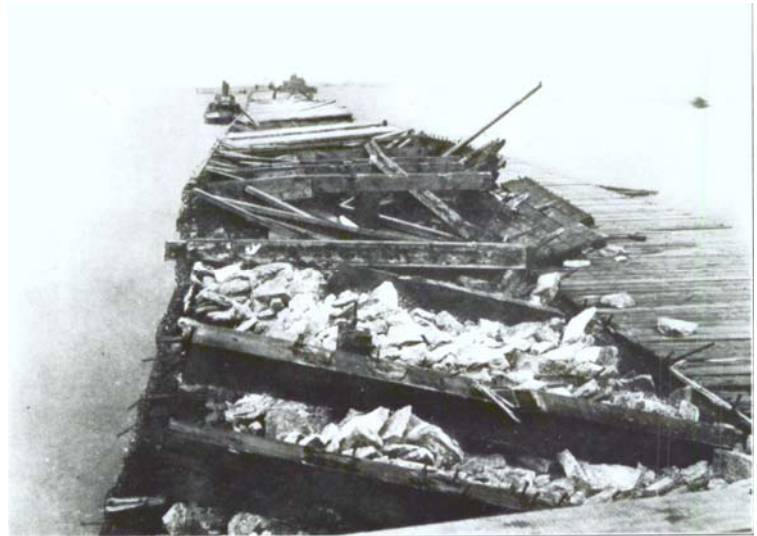
Figure 6. West Breakwater, Cleveland harbor, 1905. Showing timber superstructure in a state of decay before it was improved with concrete. ( Transactions of the American Society of Civil Engineers , 54A)
