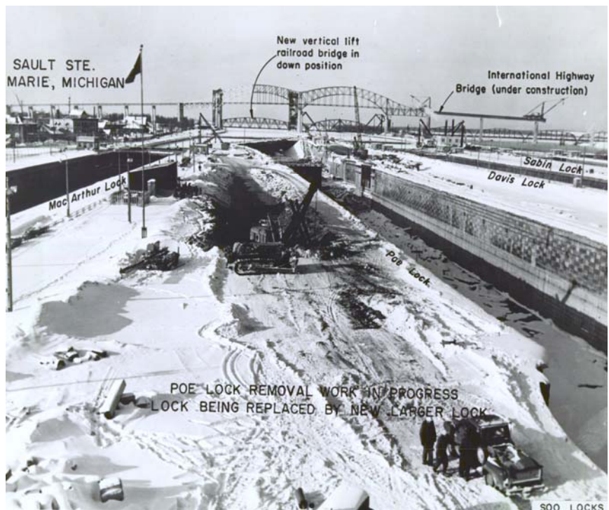
Figure 32. Poe Lock removal in progress. (NCD Files)
