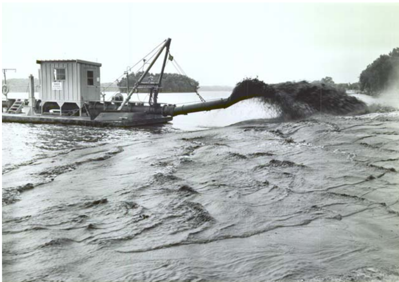
Figure 58. Shore end of the discharge pipe of the dredge William A. Thompson . Dredge material is being discharged into a spoil area along the right bank of the Mississippi River, downstream from Buffalo, Iowa, in September 1966. (Rock Island District)
