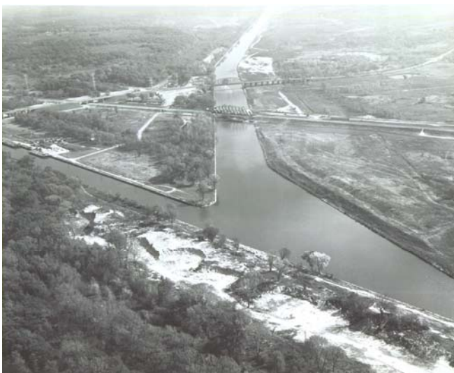
Figure 34. Junction of Sag Channel with main sanitary canal after widening, 1962. Note two new bridges constructed as part of the Calumet-Sag Channel improvement. (Chicago District)
