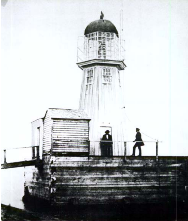
Figure 7. East pier at Ashtabula harbor, Ohio, 1859. Showing timber construction used on early harbor works and an example of the beacons constructed by Army engineers for the Treasury Department. (Canal Park Museum)
