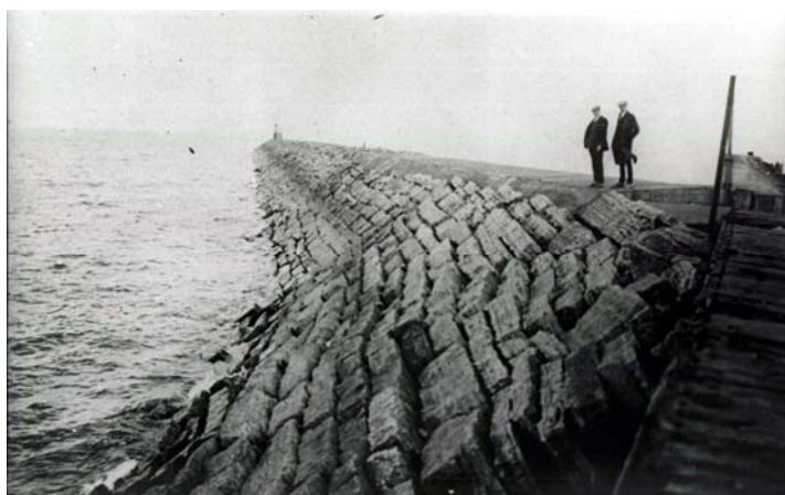
Figure 20. Rubble-mound south entrance arm breakwater at Buffalo harbor, N.Y., circa 1912. (NCD Files)
