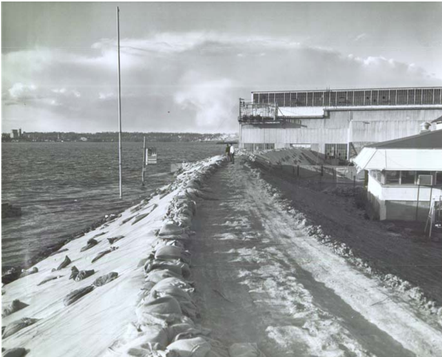
Figure 56. Operation Foresight flood emergency levee built at Rock Island, Illinois, in advance of 1969 spring flood on Mississippi River. There was not enough room on the river side of the building for the emergency levee, so it was built right through the middle of the building in background. (NCD Files)
