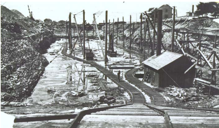
Figure 13. Excavation for the Weitzel Lock chamber at St. Marys Falls, 1876. It was 515 feet long, 80 feet wide, and 17 feet deep over its sill. (Michigan State Archives)
