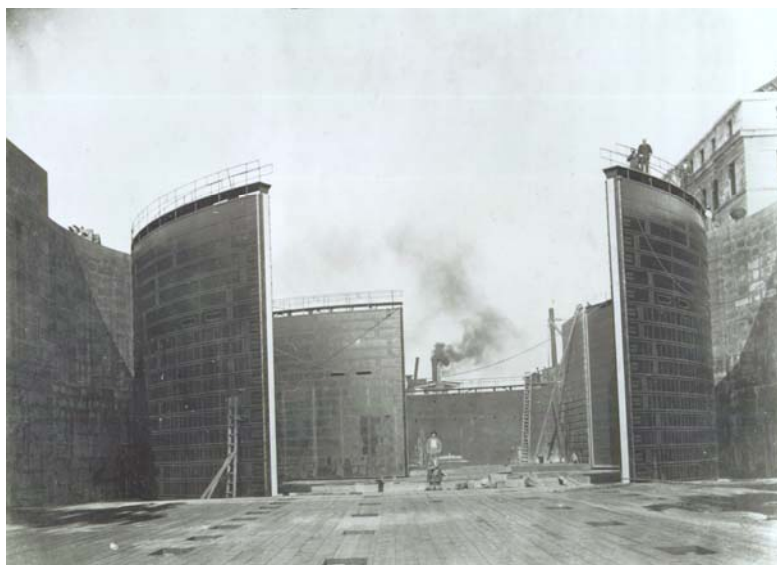
Figure 16. Gates in Poe Lock, July 1896. (NCD Files)
