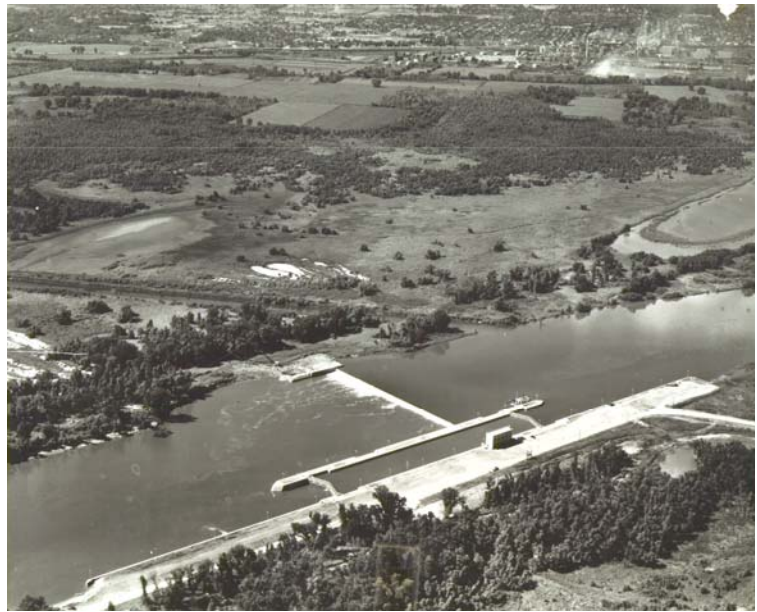
Figure 23. Peoria Lock and Dam, Illinois Waterway System, August 4, 1939. The wickets are in the raised position. (Chicago Aerial Survey Company)
