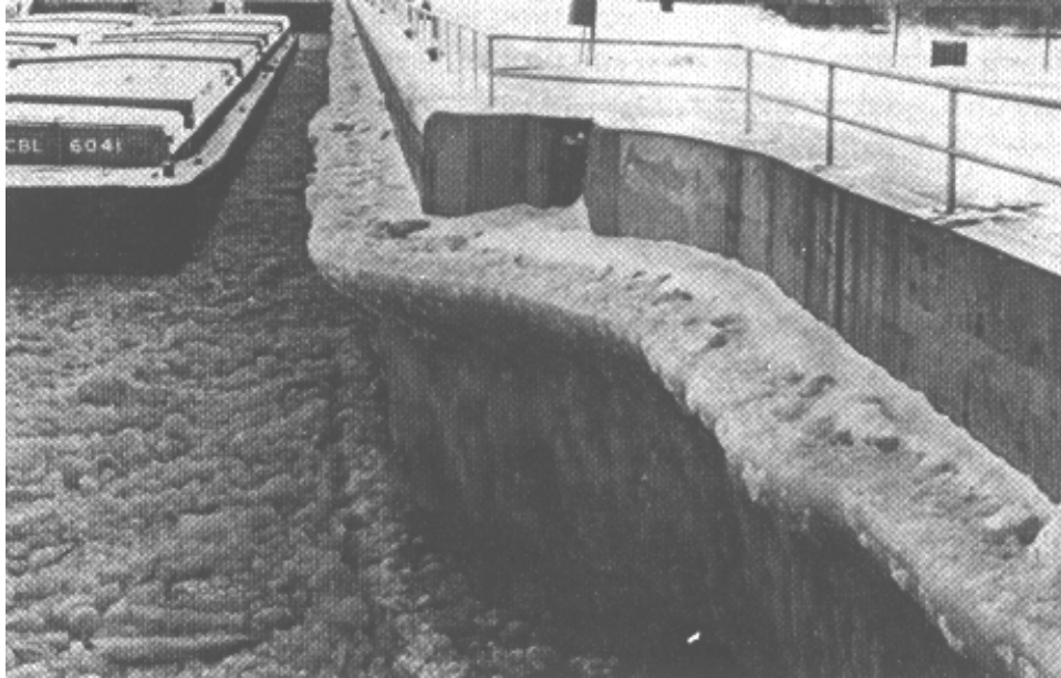
Figure 14-4. Ice collar formation on the gate recess and chamber walls, restricting the full opening of the miter gates and limiting the usable width of the lock
