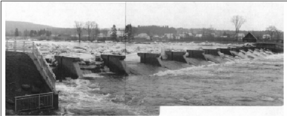
Figure 3-37. Weir with piers ice control structure on the Ste. Anne River, St. Raymond, Quebec. (Photo courtesy of Marc Delagrave, Roch Itée Groupe-conseil, Sainte-Foy, Quebec.)
