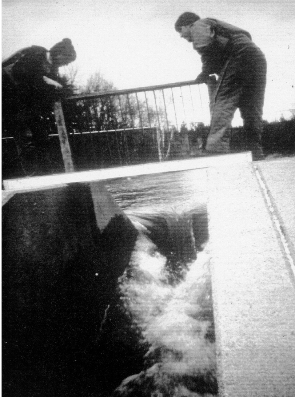
a. Installing racks in sluiceways
