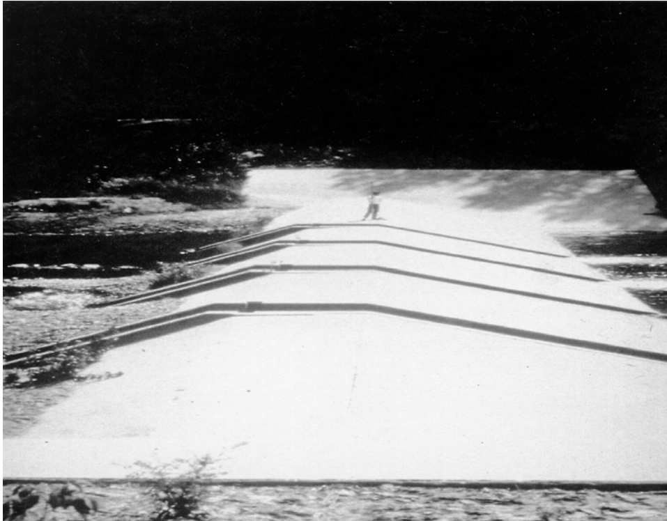
Figure 12-1. Lancaster, New Hampshire, ice-control structure
