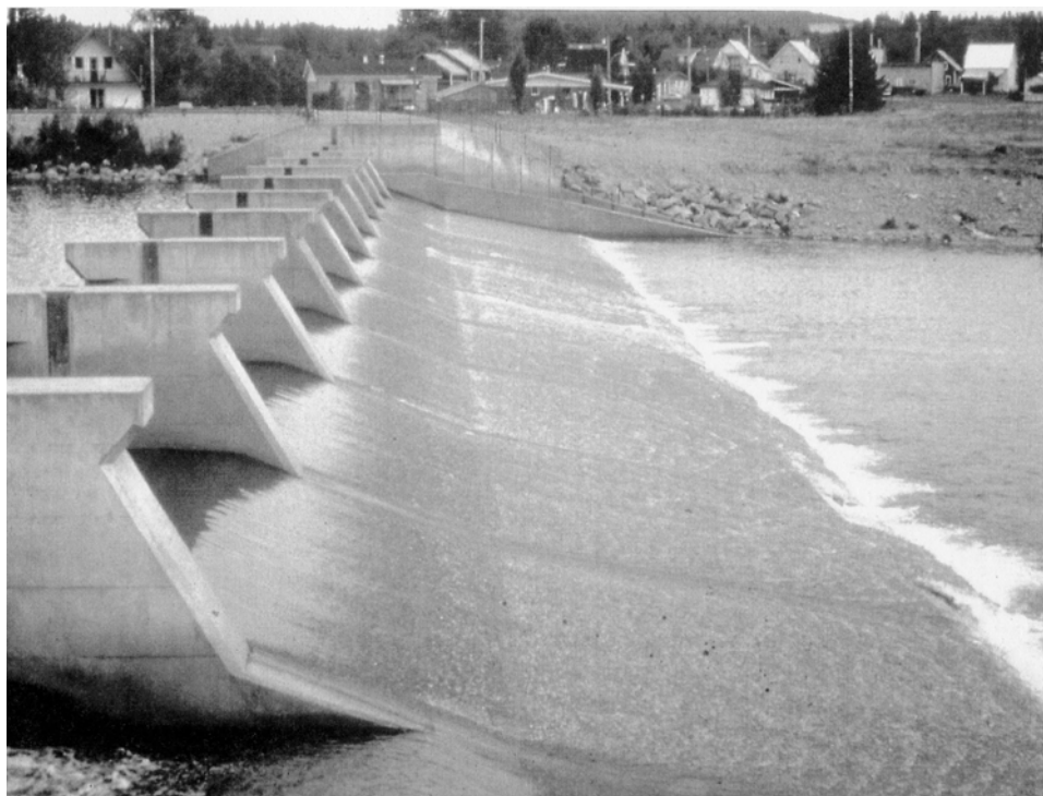
Figure 12-5. Ice piers for breakup control
