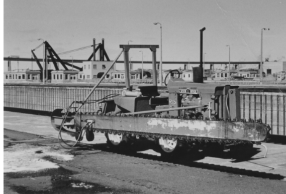
Figure 18-19. Ice cutting saw at Poe Lock.
