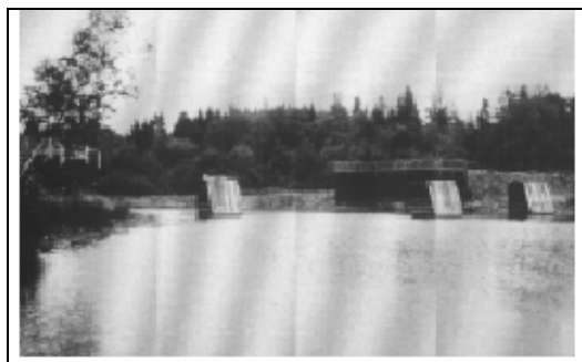
Figure 3-38. Rock-filled timber cribs upstream of the dam at Cherryfield, Maine.
