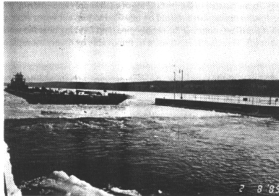
Figure 18-9. Upper screen in operation at Starved Rock Lock, Illinois Waterway. Much brash ice is prevented from entering the lock chamber, even with the entry of downbound tows.
