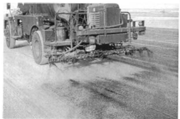
FIGURE 14-8 Improperly adjusted distributor.
