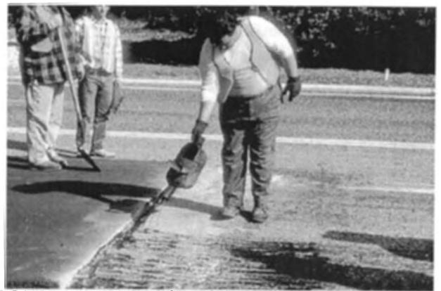
**FIGURE 17-3 Application of tack at butt joint.**
