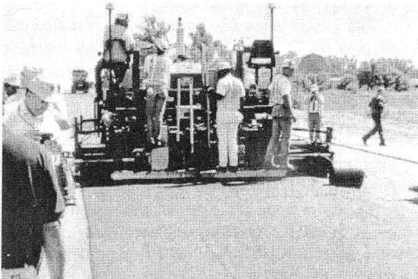
**FIGURE 17-17** Compaction of mix in wedge joint.
