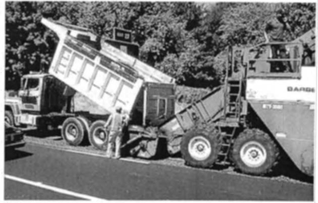
FIGURE 13-5 Material transfer vehicle.
