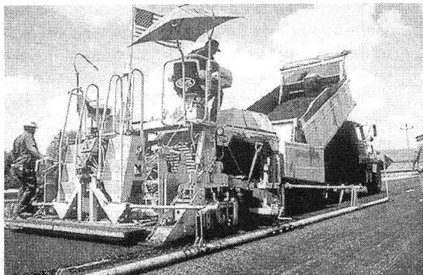
**FIGURE 16-4** Paver with mobile reference employing rigid pipe.
