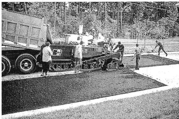
**FIGURE 14-1** Patches placed with paving machine.
