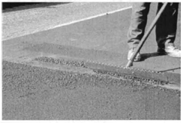
**FIGURE 17-6** Raking of transverse joint.
