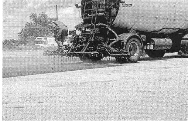
FIGURE 14-7 Distributor applying tack coat.
