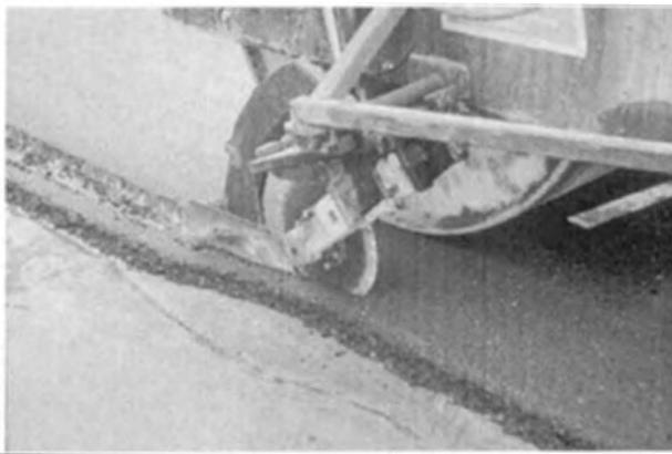
**FIGURE 17-11** Cutting wheel used to construct longitudinal joint.
