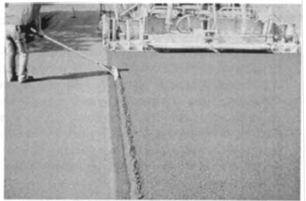
FIGURE 17-13 Raking of longitudinal joint.
