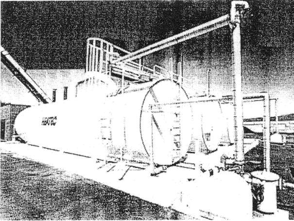
**FIGURE 7-1** Typical horizontal asphalt cement storage tanks.
