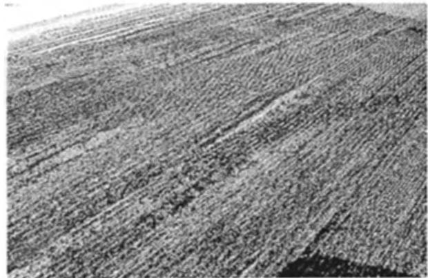
FIGURE 14-6 Tack coat on milled surface.
