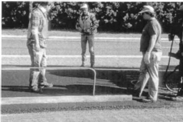
**FIGURE 17-8** Checking smoothness at transverse joint.
