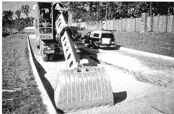
**FIGURE 14-2** Removal of existing pavement prior to patching.
