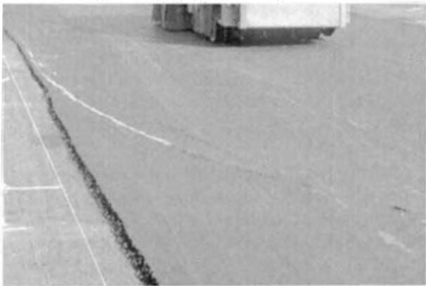
**FIGURE 19-10** Roller marks in freshly laid asphalt pavement.
