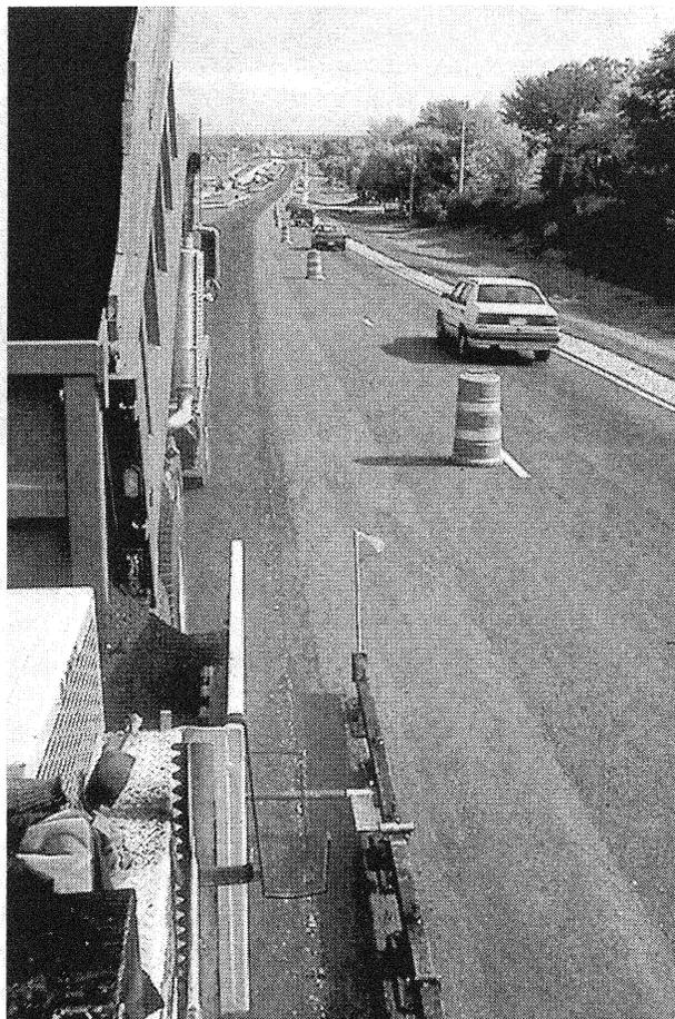
**FIGURE 16-5** Floating-beam mobile reference.
