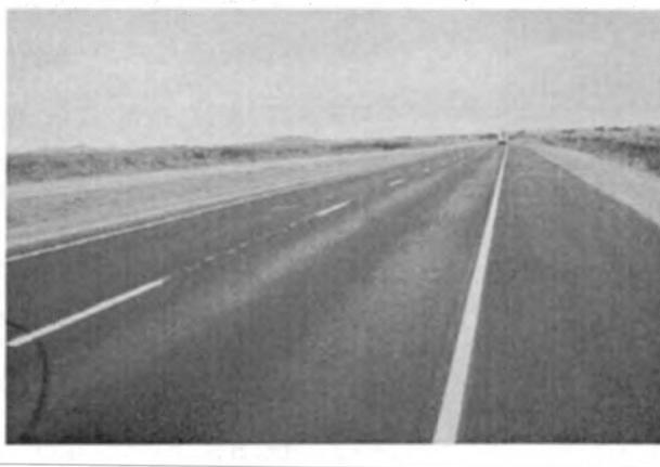
FIGURE 19-7 Asphalt bleeding in travel lane.
