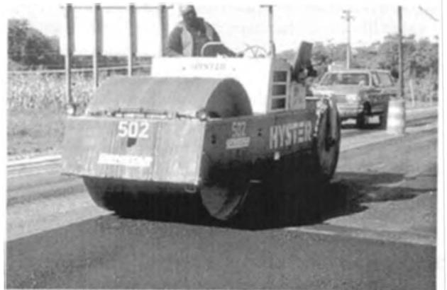
**FIGURE 17-10** Longitudinal rolling of transverse joint.
