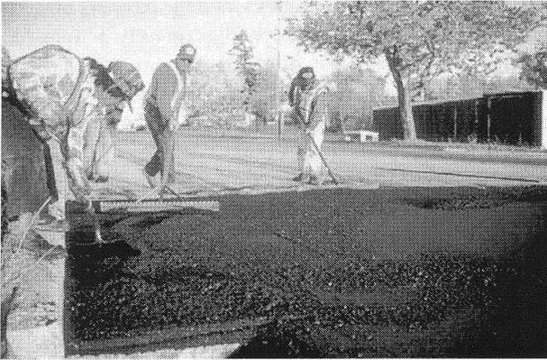
**FIGURE 17-7** Excessive raking of transverse joint.
