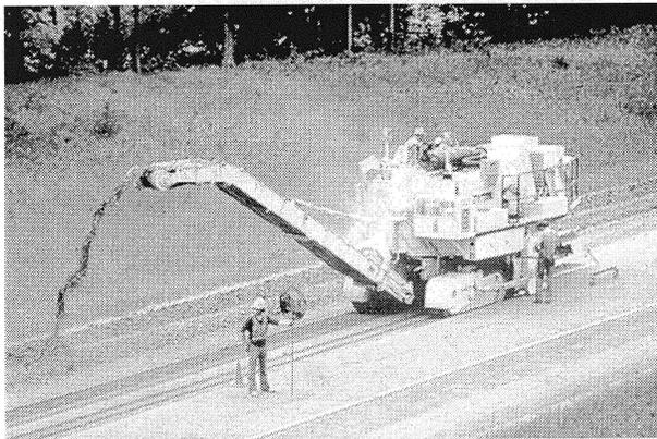
FIGURE 14-5 Typical milling machine.
