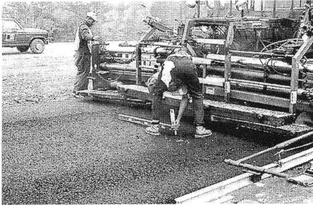
**FIGURE 16-11** Checking slope of mat surface behind paver.
