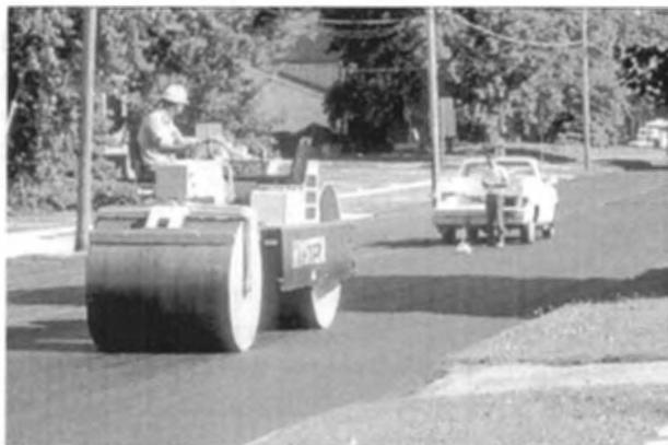
FIGURE 18-3 Static steel wheel roller.
