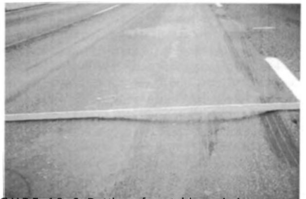
**FIGURE 19-6** Rutting of unstable asphalt mixture.
