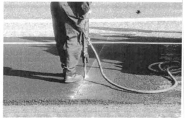
**FIGURE 17-2 Removal of material at butt joint.**
