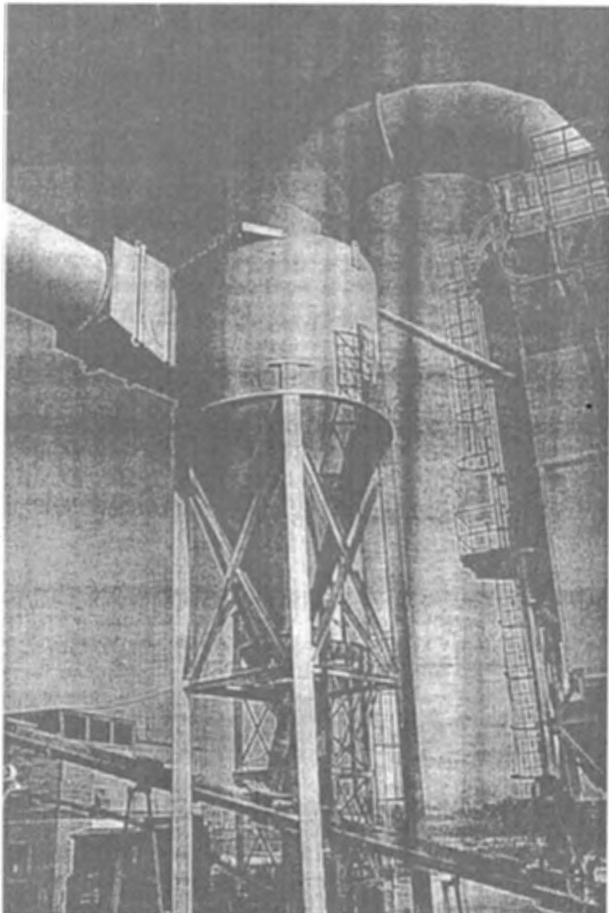
**FIGURE 12-1** Vertical cyclone dry collector.
