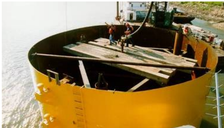
Figure A-112. Placing tremie concrete.
