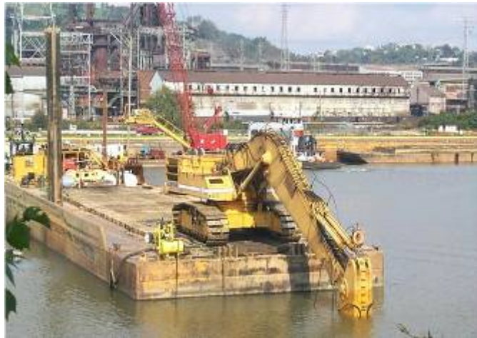
Figure A-76. Hydraulic backhoe dredging dam footprint.
