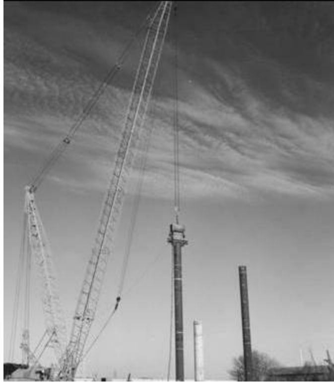
Figure A-72. Pile-mounted submersible hammer.
