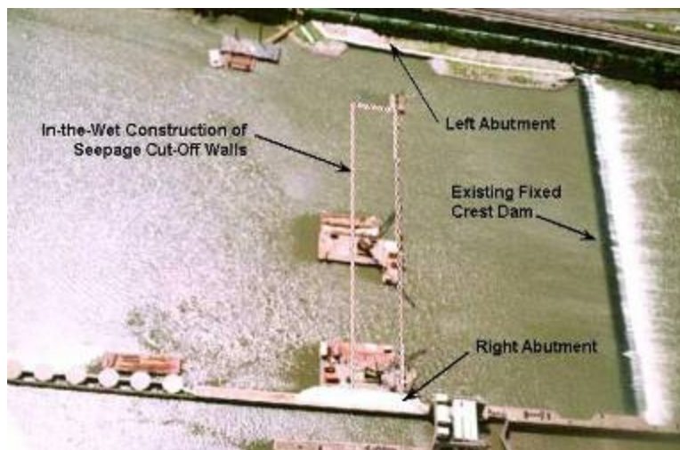
Figure A-77. Alignment of seepage cut-off walls.
