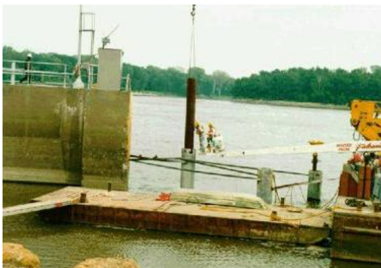
Figure A-104. Installation of a guide pile.
