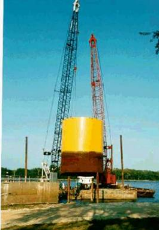
Figure A-109. Cell installation.
