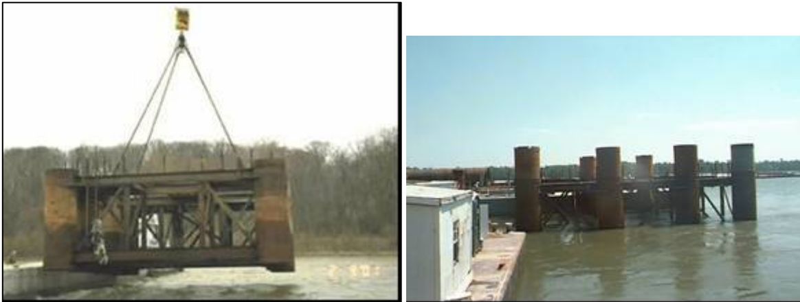
Figure A-63. Nose pier template.
