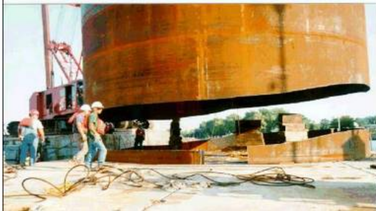
Figure A-108. Bottom of cell scribed and cut to match rock surface.
