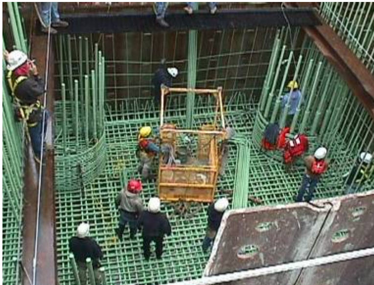
Figure A-16. Bath-Woolwich Bridge dewatered cofferdam.
