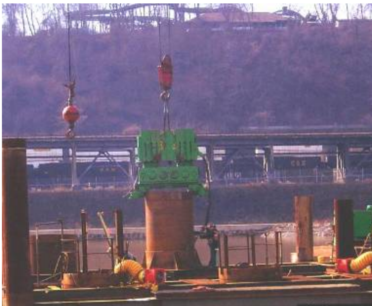
Figure A-89. Vibratory driving drilled shaft casing.
