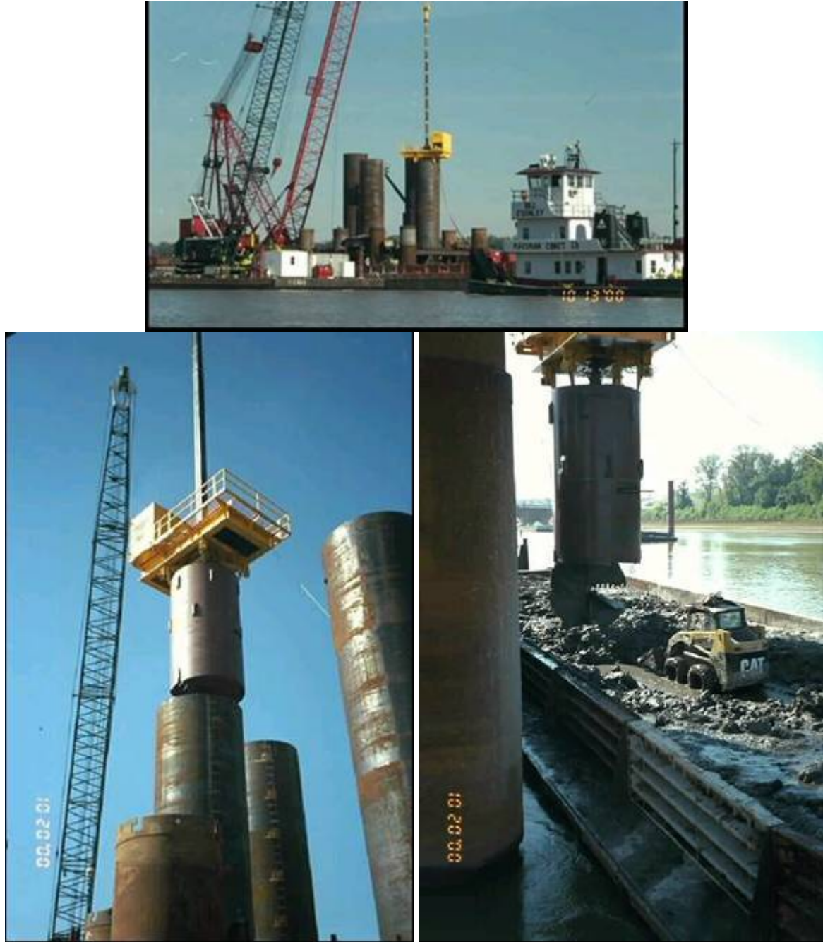
Figure A-65. Pile top drill with 9-foot cleanout bucket with extendable wings to 9 ft 8 inches.
