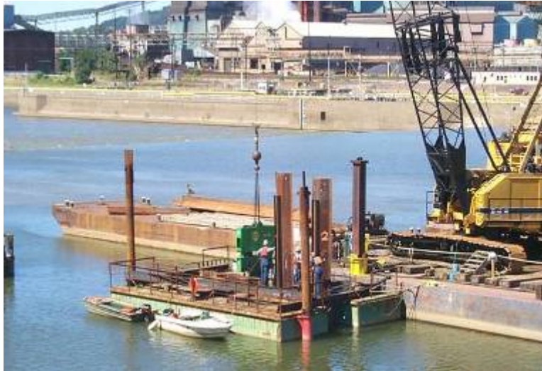
Figure A-85. Driving sheets for left side cut-off wall.
