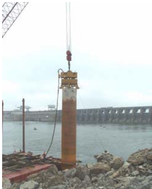
Figure A-116. Driving temporary casing.
