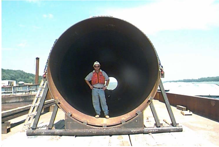
Figure A-62. Shaft casings with 10-foot diameter.
