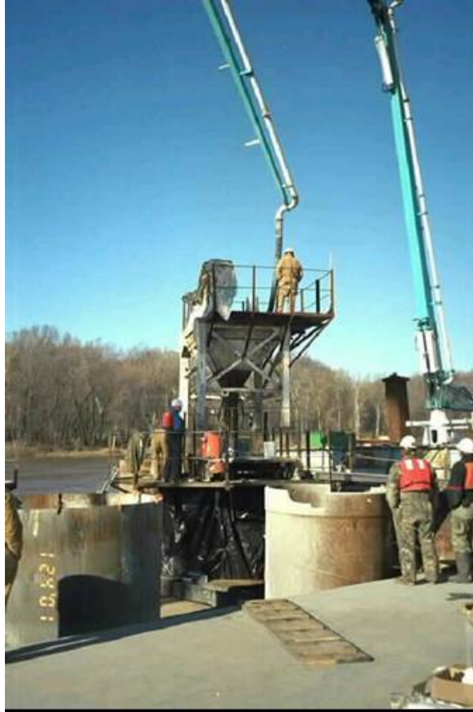
Figure A-70. Tremie concrete placement.
