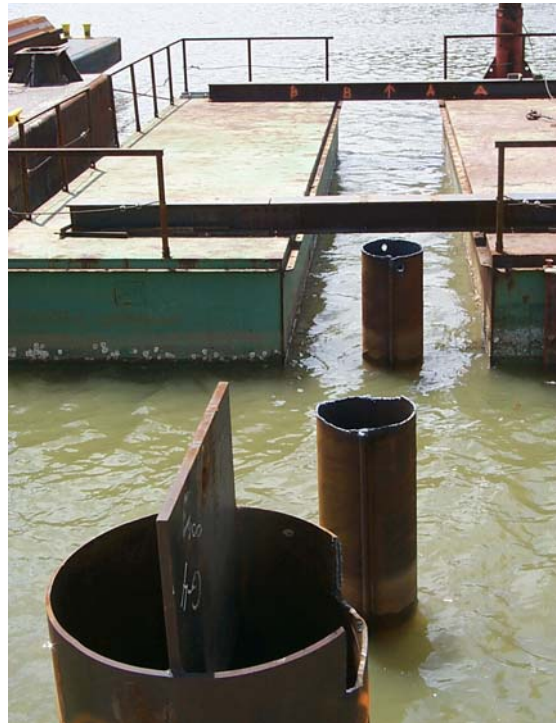
Figure A-28. King-piles floating template.
