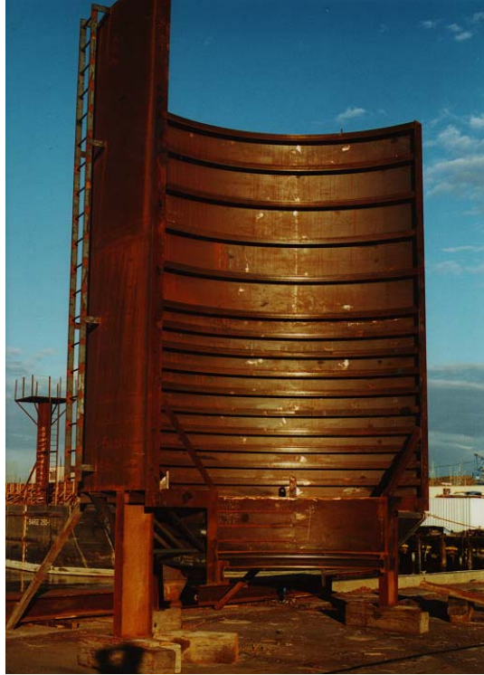
Figure A-1. One-half of temporary circular cofferdam used to cut off the 3-meter-diameter drill shaft casings underwater at the New Carquinez Bridge.
