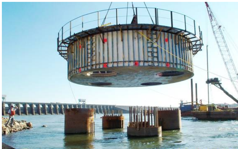
Figure A-129. Setting pier base form.
