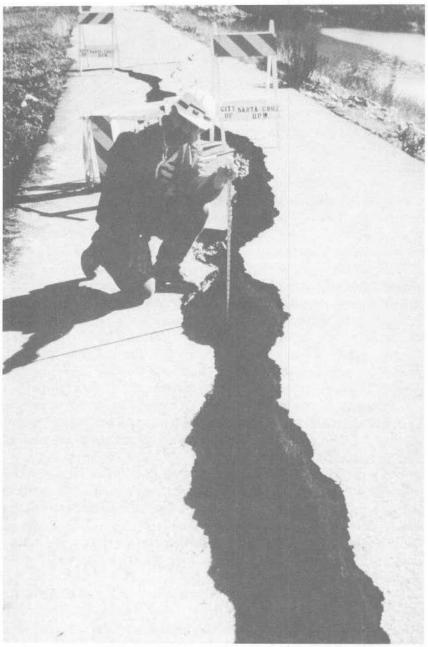
A Corps inspector measures a fracture in the Pajaro River levee.
