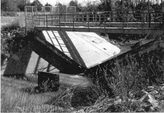
Figure 6-12. Flume-type grade control/gauging structure
