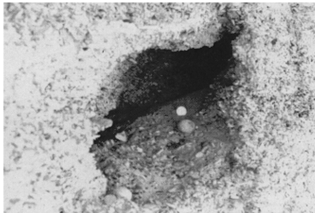
Figure 4-7. Piping and seepage in bank
