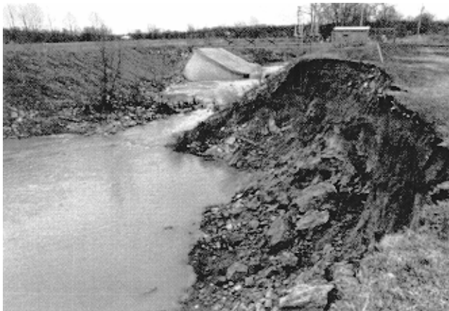
Figure 4-6. Bank failure
