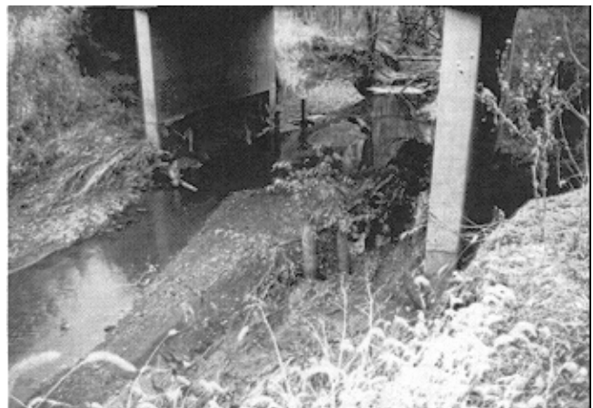
Figure 4-11. Exposed bridge piling
