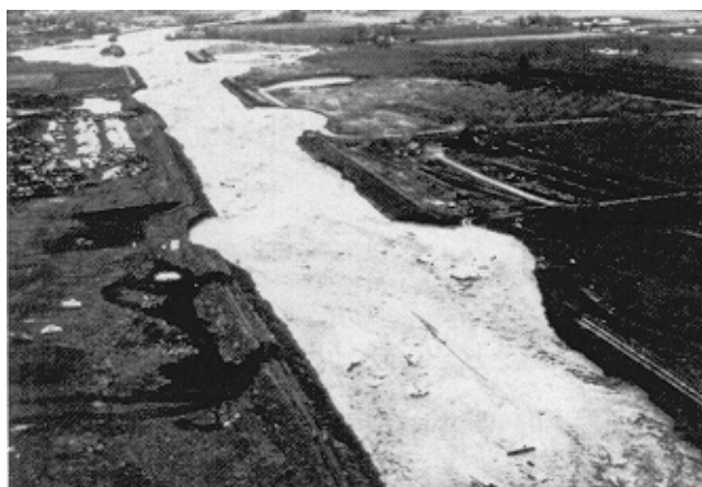
Figure 3-6. Lateral instability in realigned channel
