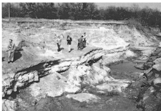
Figure 3-13. Grapevine Spillway Channel after erosional episode
