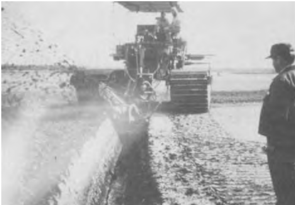
Figure 5-19. View of rotary trenching device in operation
