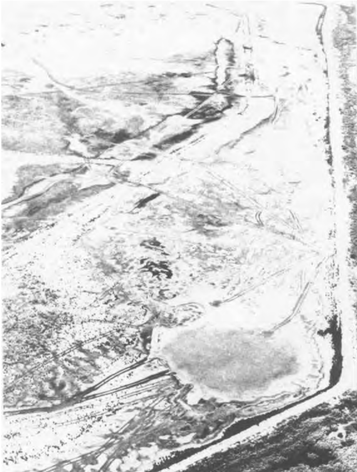
Figure 5-24. Aerial view of sequential radial trenching procedure used when interior cross dikes are encountered, South Blakely Island Disposal Site of the Mobile District
