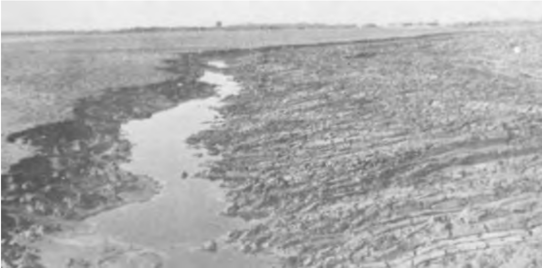
Figure 5-11. Construction of ditch 12 to 18 inches deep with excavated material cast on interior slope of perimeter dike
