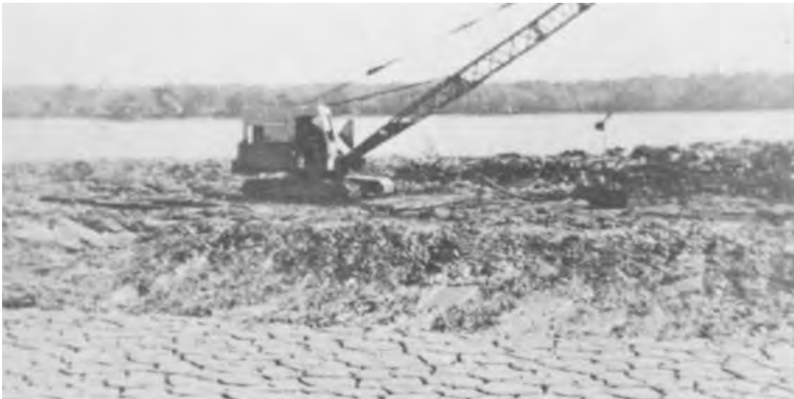
Figure 5-10. Small dragline on mats working on berm deepens shallow perimeter drainage trench
