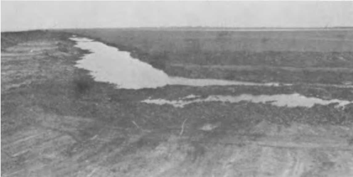
Figure 5-13. A well-developed perimeter trenching system, Morris Island Disposal Site, Charleston District
