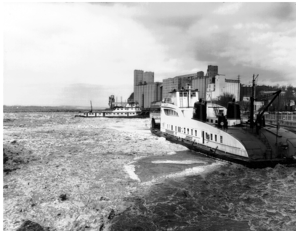
Figure 10-6. Towboats H.L. Frieberg (left) and Dan Luckett (right) breaking ice in the upper lock forebay, Lock and Dam 26, February 1966.
