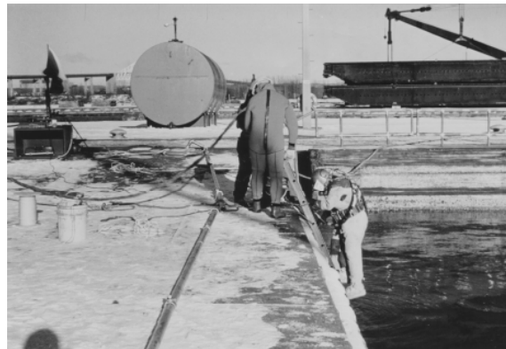
Figure 18-13. Diver working to install air screen system.
