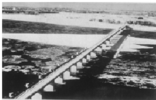
Figure 18-4. Montreal Harbor ice control structure. (From Lawrie 1972.)
