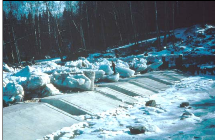
Figure 3-27. Ice control weir on the Israel River, Lancaster, New Hampshire, July 1994.
