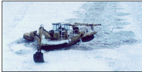
Figure 3-11. Breaking ice with an amphibious excavator on the Aroostook River, Ft. Fairfield, Maine.
