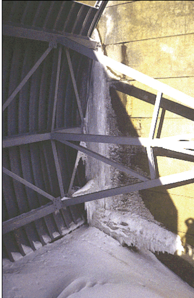
Figure 20-1. Column of ice formed on the downstream side of a tainter gate from water leaking past the side seal. The ice forms a bridge between the gate and pier. Such accumulations prevent movement of the gate. To restore normal gate operations, the ice needs to be removed by melting, chipping, or cutting. Photo of Gavens Point Dam, Yankton, SD.
