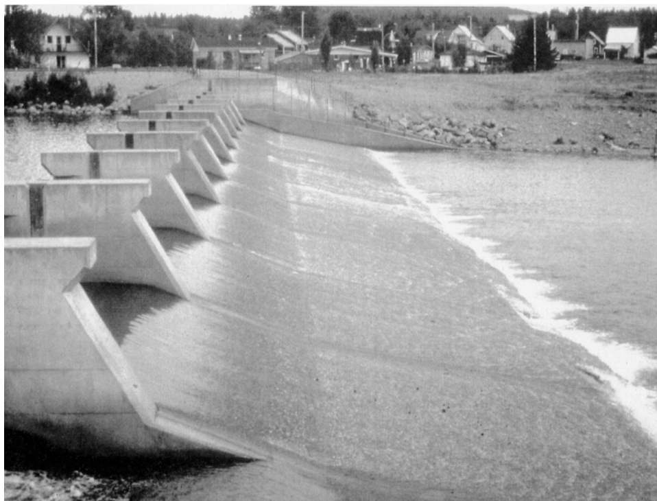
Figure 12-5. Ice piers for breakup control
