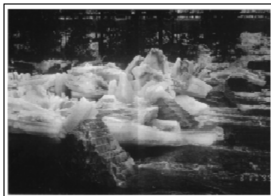
Figure 3-34. Cut granite block ice control structure in Hardwick, Vermont, following breakup, March 1995.
