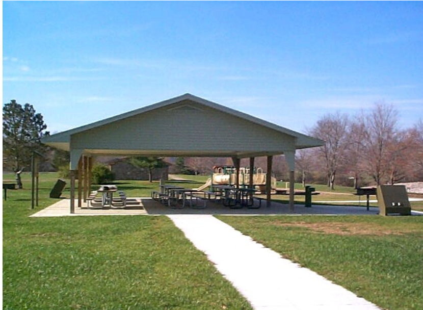
Photo P-7. Picnic shelter features and amenities, View 1. Cave Run Lake, KY. Shelter is UA, has concrete apron, and is convenient to restroom and playground equipment ( Table 3.2 )
