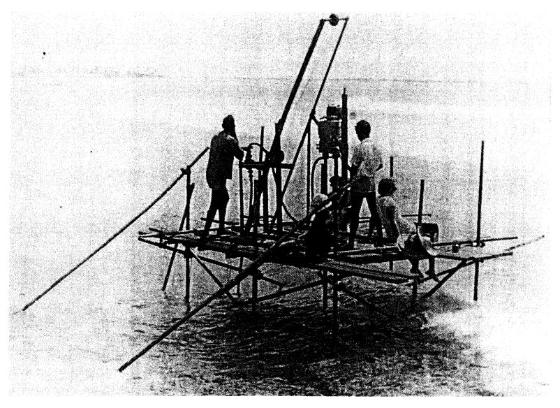
Figure 10-1. Photograph of a small drill rig on a scaffold. Note: Safety is a very important consideration for Corps of Engineer Projects. Safety items, including hardhats, gloves, safety shoes, protective clothing, life vests, and dust or vapor masks, should be worn, as appropriate, for the particular drilling and sampling operations. (Figure provided by the U.S. Naval Facilities Engineering Service Center)
